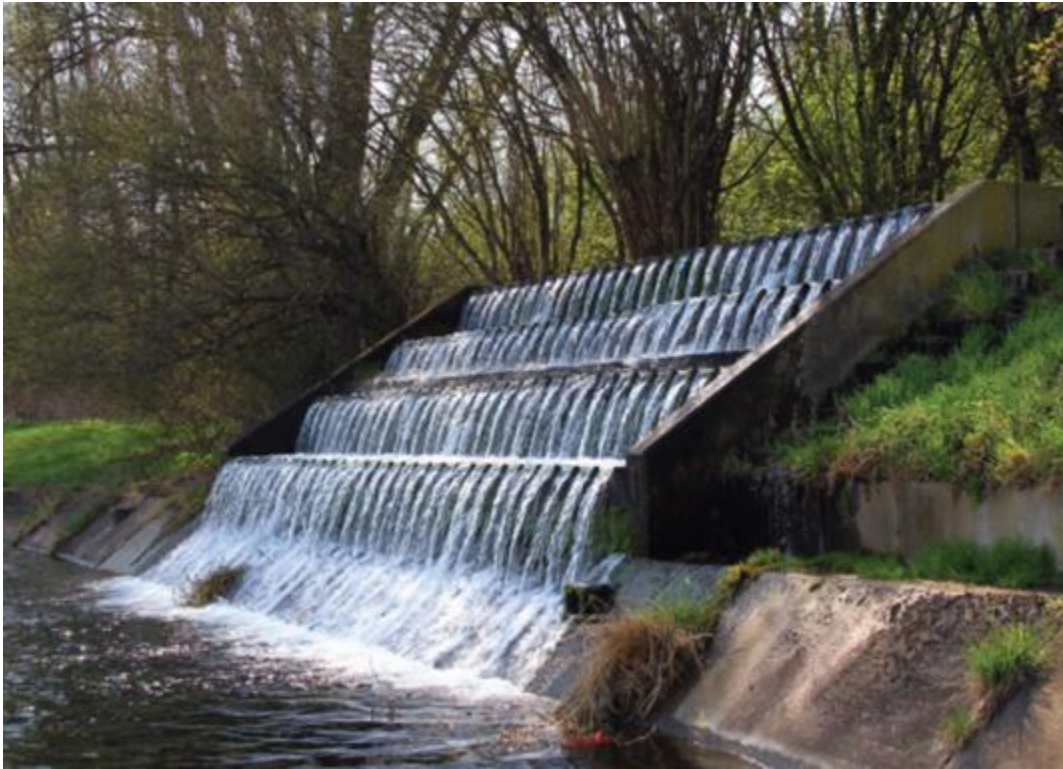
Figure 2-1 Low-cost cascade aeration system that enhances the air-water transfer of atmospheric gases (e.g., oxygen, nitrogen) and volatile organic compounds. The term “green technology” commonly invokes images of such technologies; however, green technologies span a broad spectrum of treatment typologies.
