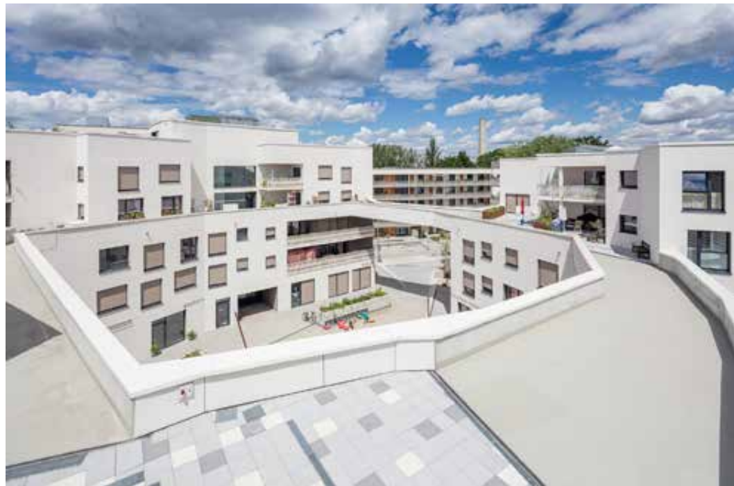
Fig. 4.51 WagnisART Roof Walkway
