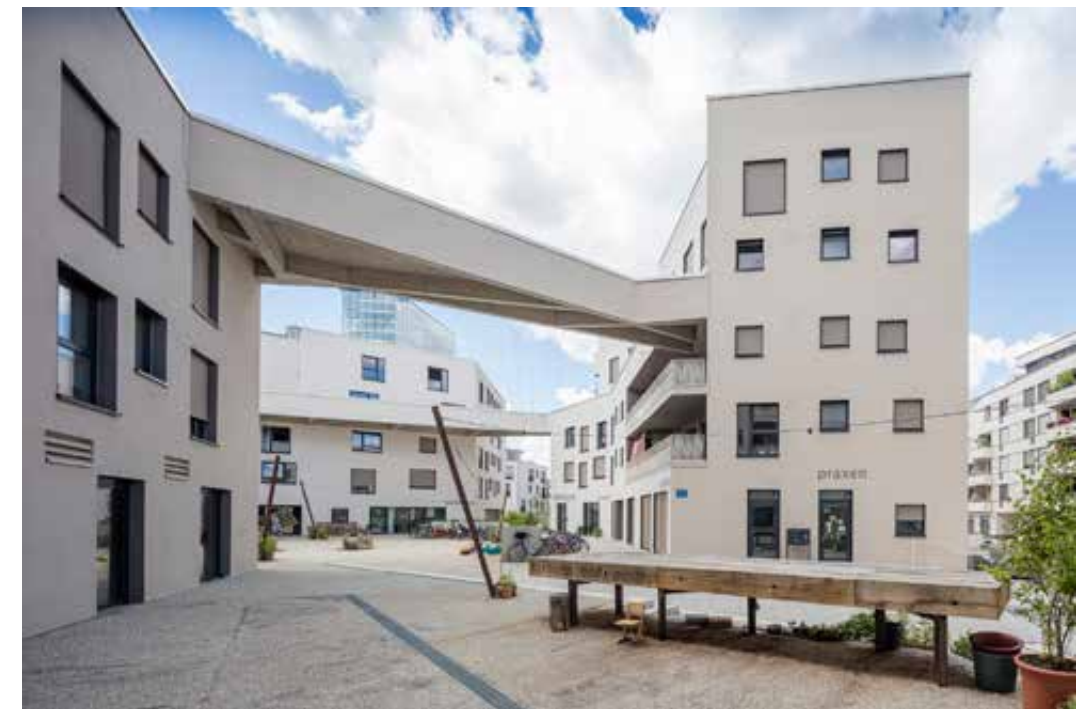
Fig. 4.49 WagnisART Exterior Complex Entrance
