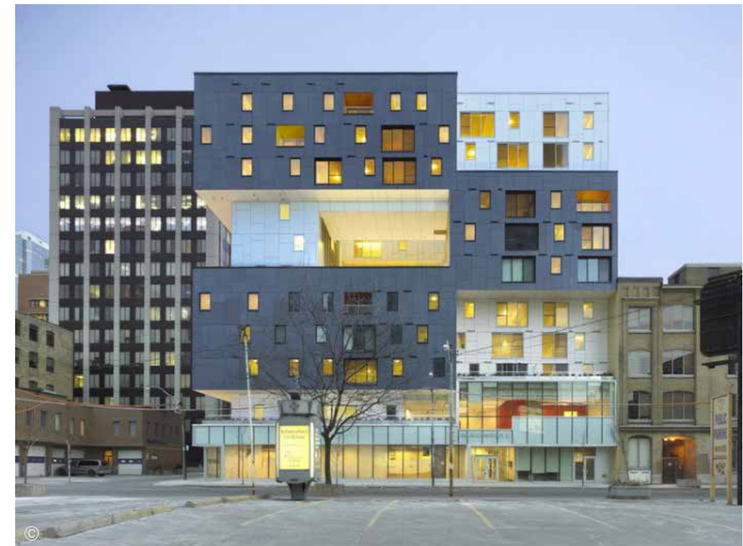
Fig. 3.5 60 Richmond Exterior View
