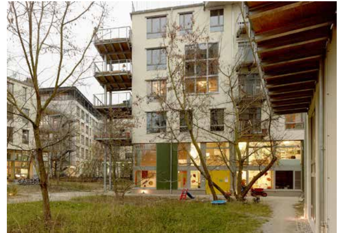
Fig. 4.14 River Spreefield Exterior View
