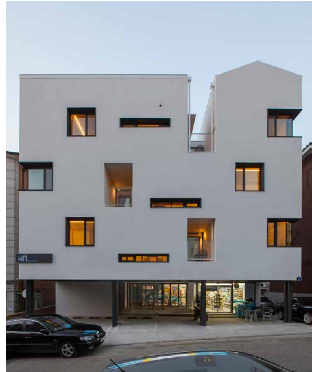
Fig. 4.42 Gap House Exterior View
