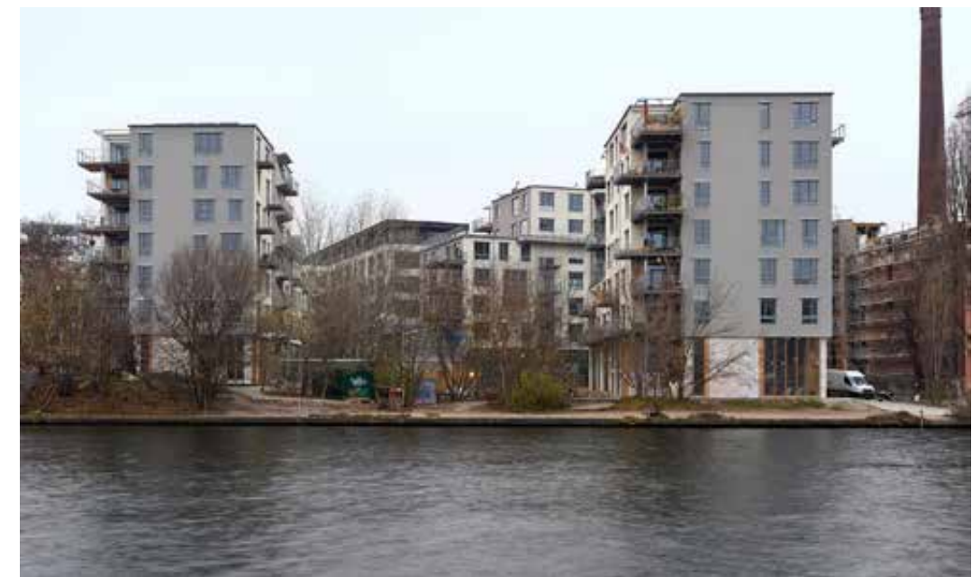
Fig. 4.15 River Spreefield River View
