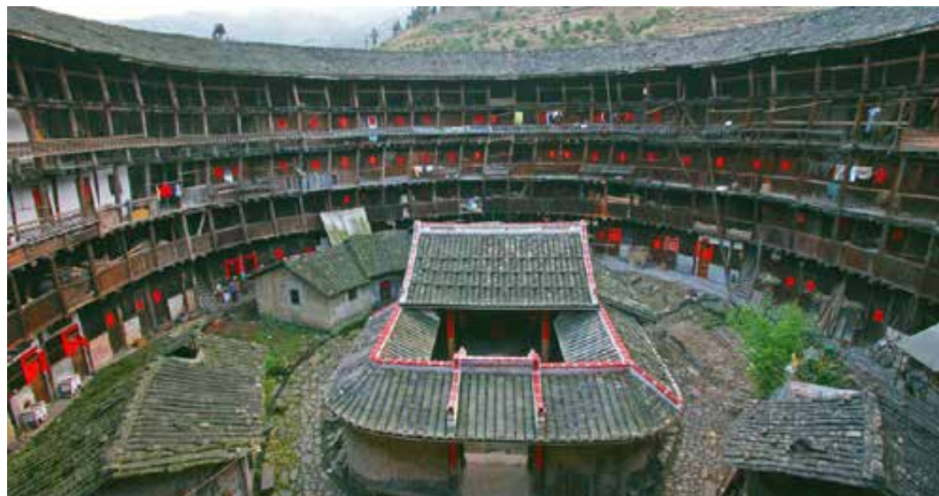
Fig. 2.9 Fujian Tulou Courtyard
