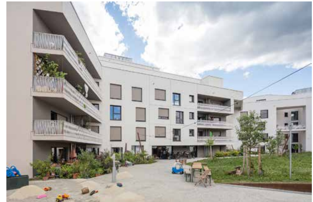
Fig. 4.53 WagnisART Exterior View
