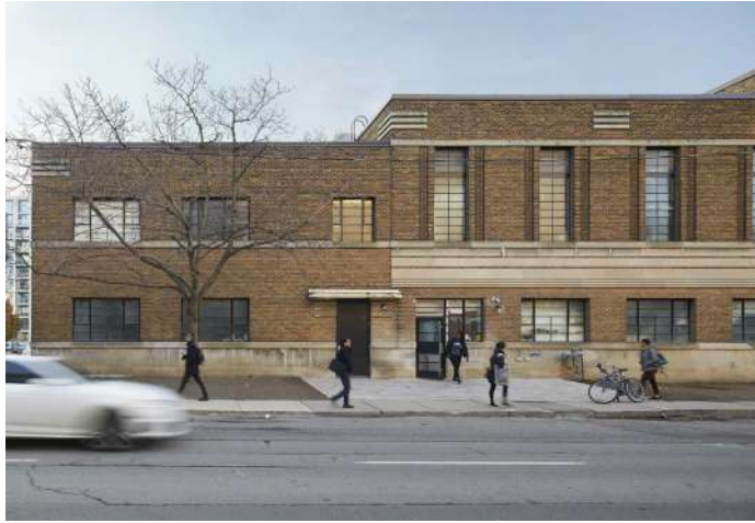
Fig2.26. The Last Precedent is Eva's Phoenix by LGA architects. A warehouse that is repurposed to be used as transitional housing for youth. Eva's offers safe and inclusive long-term shelter, education and skills training to marginalized youth aged 16-24 in transition from homelessness to independent living.
