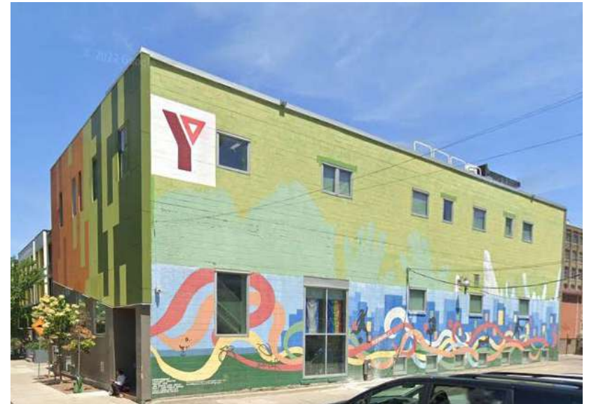
Fig2.16. Wagner Green shelter has 40 beds and we provide harm-reduction and trauma-informed residential services to at-risk homeless young men, ages 16–24.
