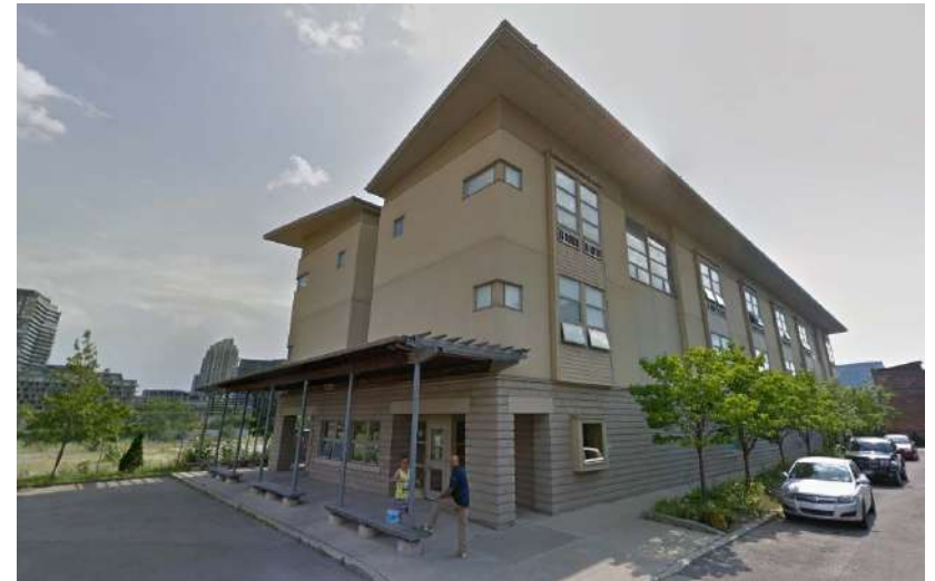
Fig2.13. Fort York Residence is three storeys and houses 74 shelter beds and 24 self-contained bachelor units. The shelter beds are dormitory-style with low level walls dividing the spaces into groups of two or eight. Each resident is provided a locker to store personal belongings and access to a shared laundry facility, lounge, dining hall and resource center.
