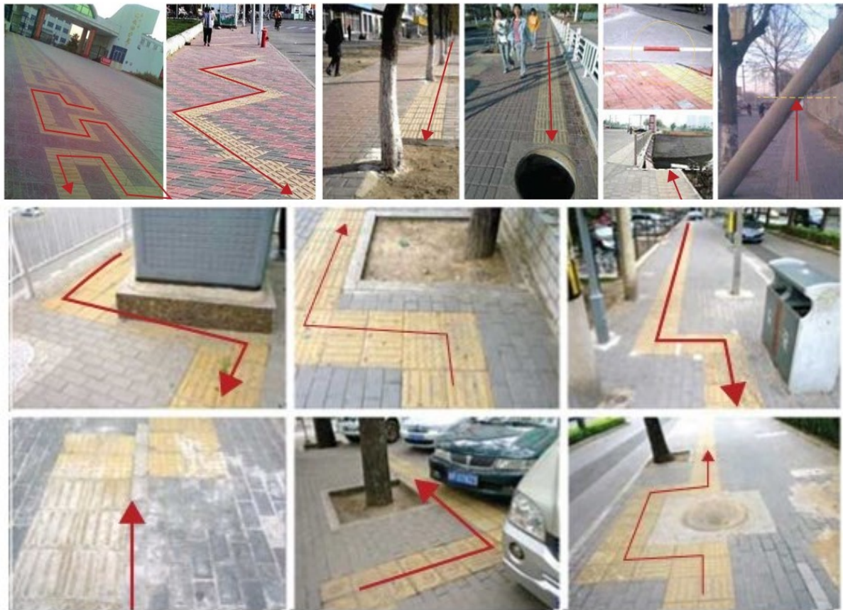
Figure 3.15 Examples of Compliance becoming Inconsistent with introduction of code in China
