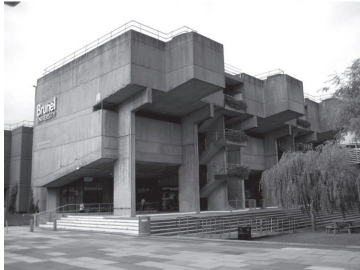
Figure 1.4 Stairs at Brunel University, UK (Photo by Ken MacLeod)
