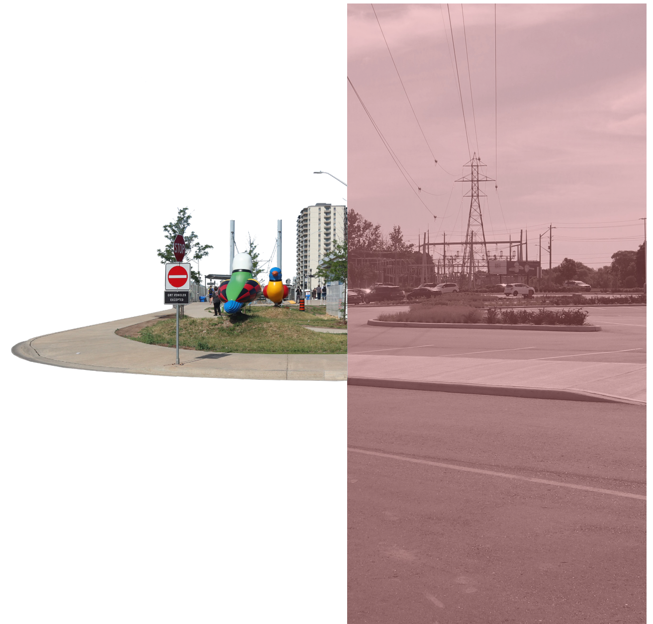
FIG. 5. 39. The south end of Phase 1. The terminal sculpture is not so far from low income neighbourhoods that have had their mobility reduced by the LRT. There's a visual tension between the necessary power infrastructure that looms in Fairview's parking lot and the sanitization that the LRT represents.
