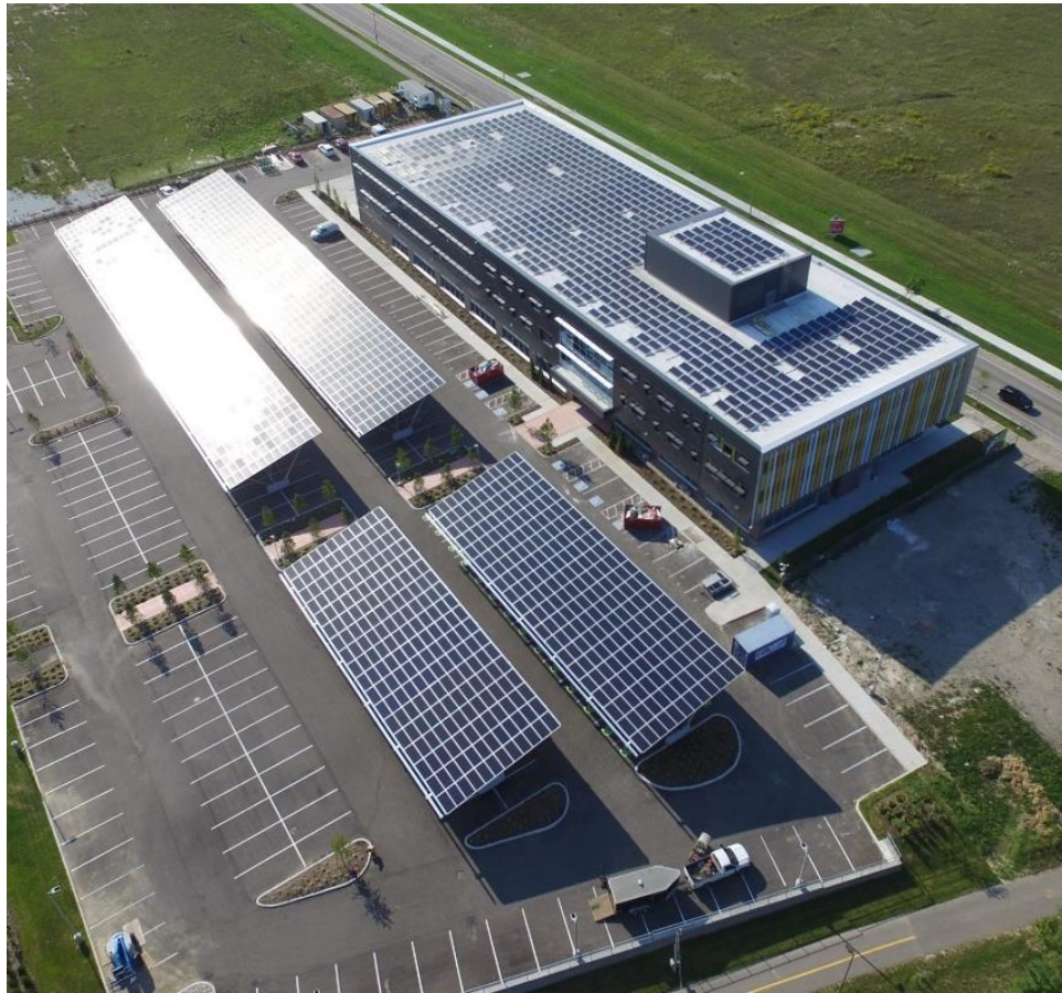
Figure 7: Case study building exterior showing parking lot and roof solar PV systems, image from (87)
