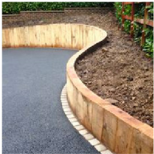
Timber Retaining wall
