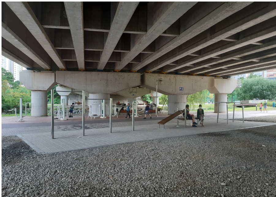
Fig. 5.29 Pet park in underpass Fig. 5.30 Exercise park in underpass
