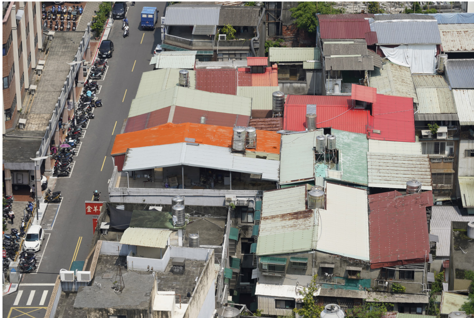
Fig. 2.11 A series of streethouses in Datong District with colourful corrugated steel rooftop additions that are used for outdoor domestic activities or rented out as low-cost apartment units. All of these additions are illegally made and cause fire-safety issues.
