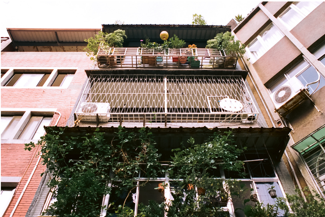
Fig. 1.3 A modern streethouse that has been localized by their owners through facade additions that provide shading strategies, protection from break-ins and a space for planting greenery.
