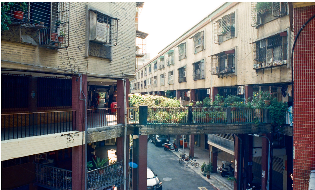
Fig. 5.101 The rows of housing segments are joined together on the second level by bridges that span across the streets.
