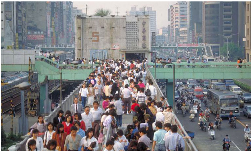
Fig. 5.89 Elevated walkways that joined together each of the housing blocks created a network of overpass bridges that stretched over the busy ground floor streets.
