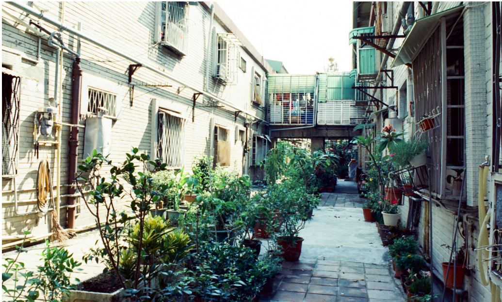
Fig. 5.100 The upper level corridor serves as an open-air terrace that is used by residents to create gardens and patios outside their units.
