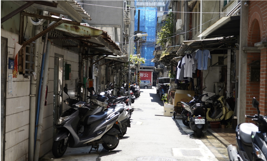
Fig. 4.67 View into the laneway on the west end of the project site. This image shows the residential entrances into the streethouses, which are constructed with illegal extensions that expand the ground floor area.
