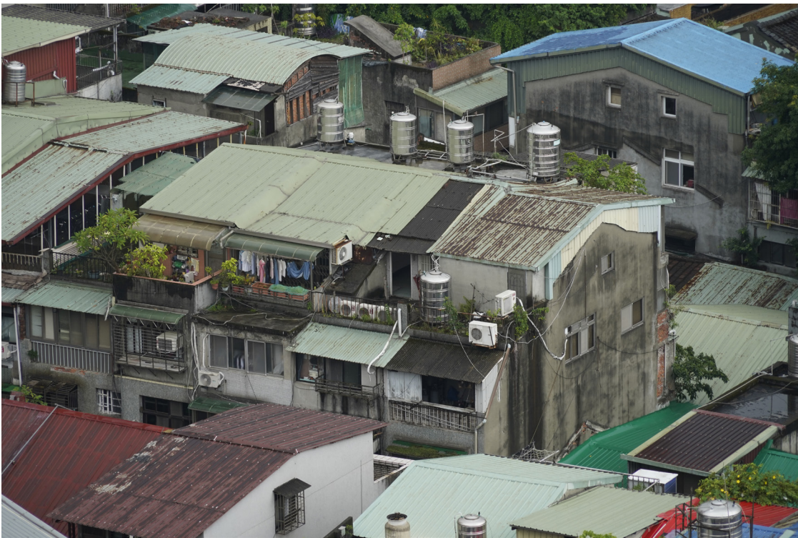
Fig. 2.6 Aerial view of a series of modern streethouse rooftops that form additional apartment units, terraces and platforms for water tanks.
