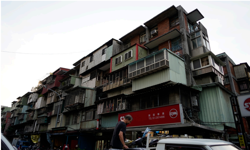
Fig. 5.94 The facade of the Nanjichang Housing Development is covered with facade extensions that households have added to increase their interior living spaces.
