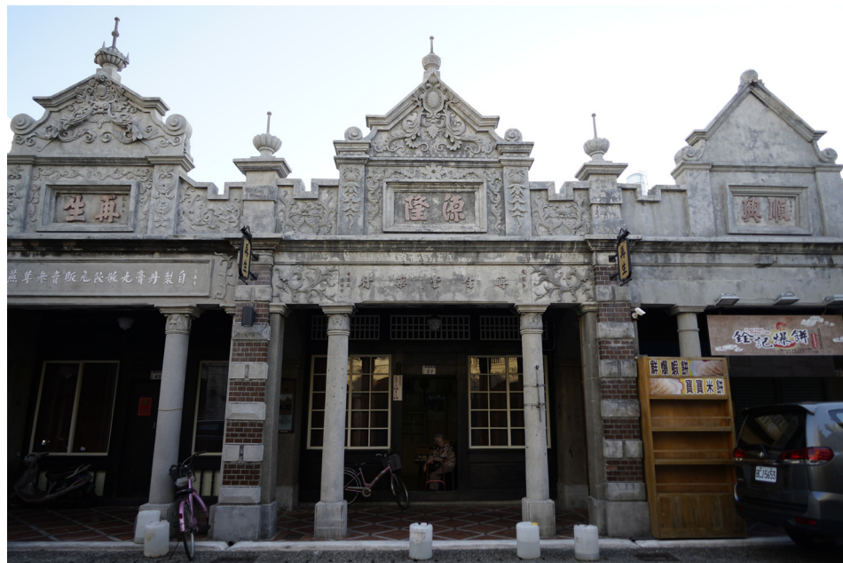
Fig. 2.10 Early Japanese-style streethouses in Daxi Old Street in Taoyuan reveal intricate ornamentation learned from the West on its facade. Each stone carving here symbolizes the meanings associated with the families that live within the streethouses.
