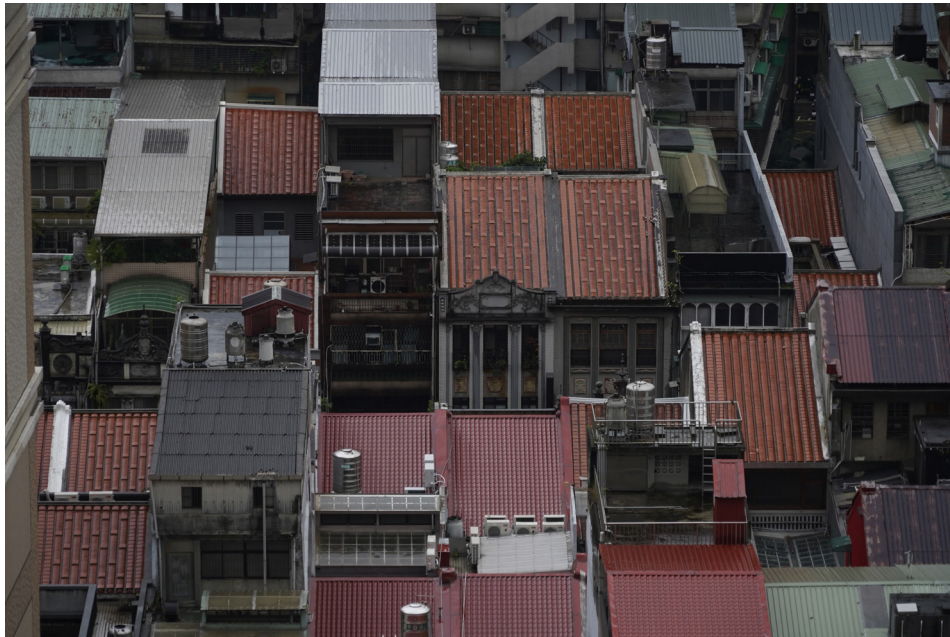
Fig. 2.9 View of streethouses from each colonial period on a single block in Dihua Street. The rooftops of Japanese-style streethouses are lined with red clay tile, whereas the modern streethouses have rooftops made with colourful corrugated metal sheets.
