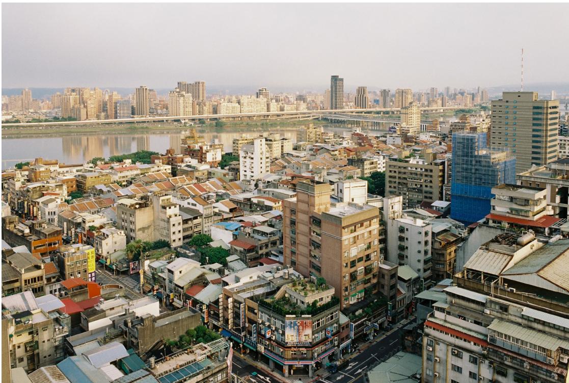
Fig. 1.2 Aerial view of Datong District facing Tamsui River. Early streethouses built during the Qing dynasty and Japanese colonial periods can be seen here by their clay tiles and arched rooftops.
