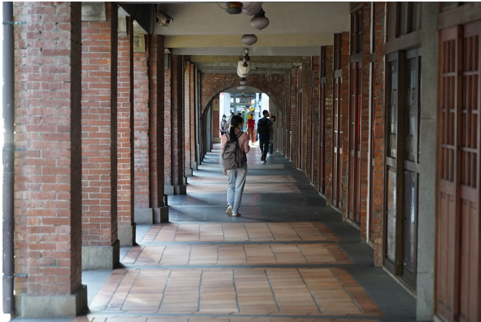
Fig. 2.7 View within the 'ding-a-ka' of preserved Minnan-style streethouses in the Bopiliao Historical Area lined with red brick and clay tiles.
