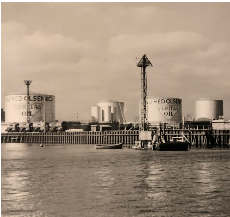
Fig. 1.13 1930's oil tanks on Petrol Island. Archival photograph from the 1930's, from the By og Havn archives.
