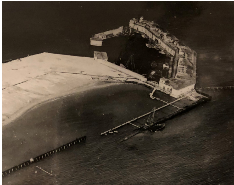
Fig. 1.11 1700's historic 'Prøvestenen' fortification with new surrounding soil infill in progress in the 1930's. Archival photograph of the construction of Petrol Island, from the By og Havn archives.
