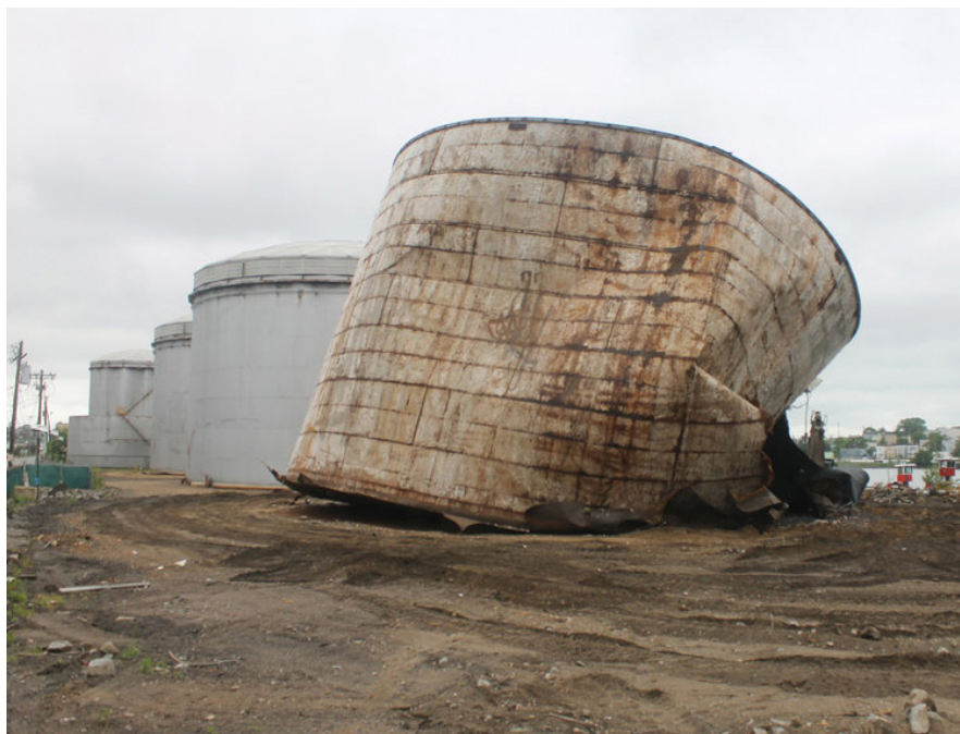
Fig. 3.11 'Tank Farm Demolition' by Landing Studio, Chelsea, Massachusetts. (Source: http://www.landing-studio.com/projects#/tank-farm-demolition/ )
