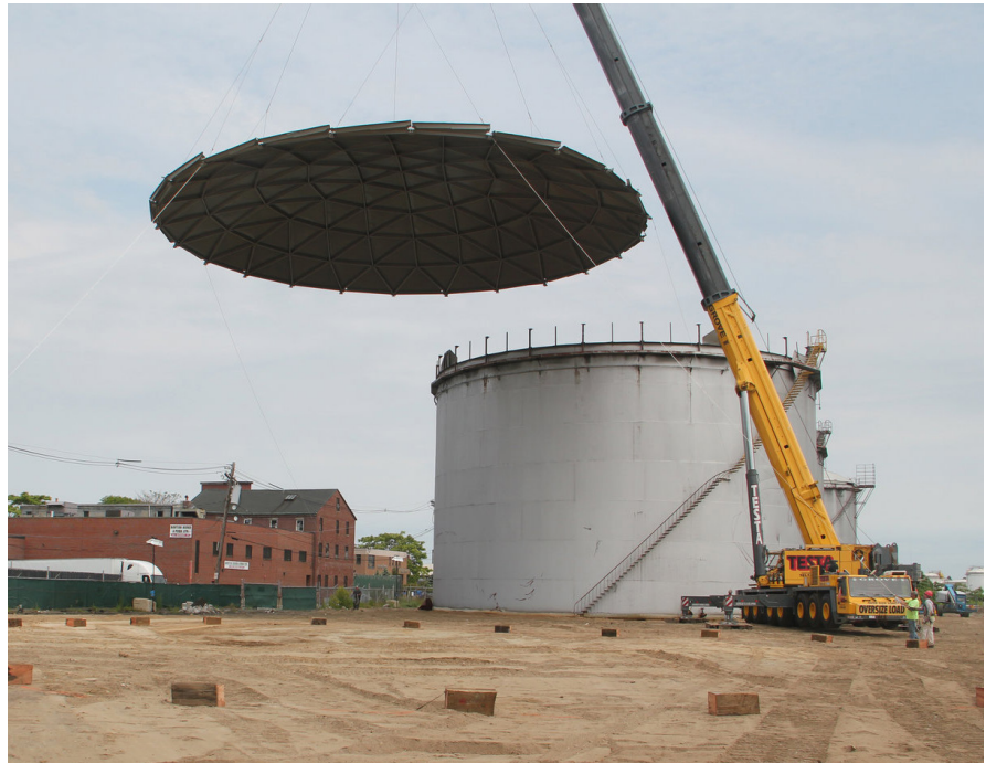
Fig. 3.12 'Tank Farm Demolition' by Landing Studio, Chelsea, Massachusetts. (Source: http:// www.landing-studio.com/projects/ tank-farm-demolition/ )
