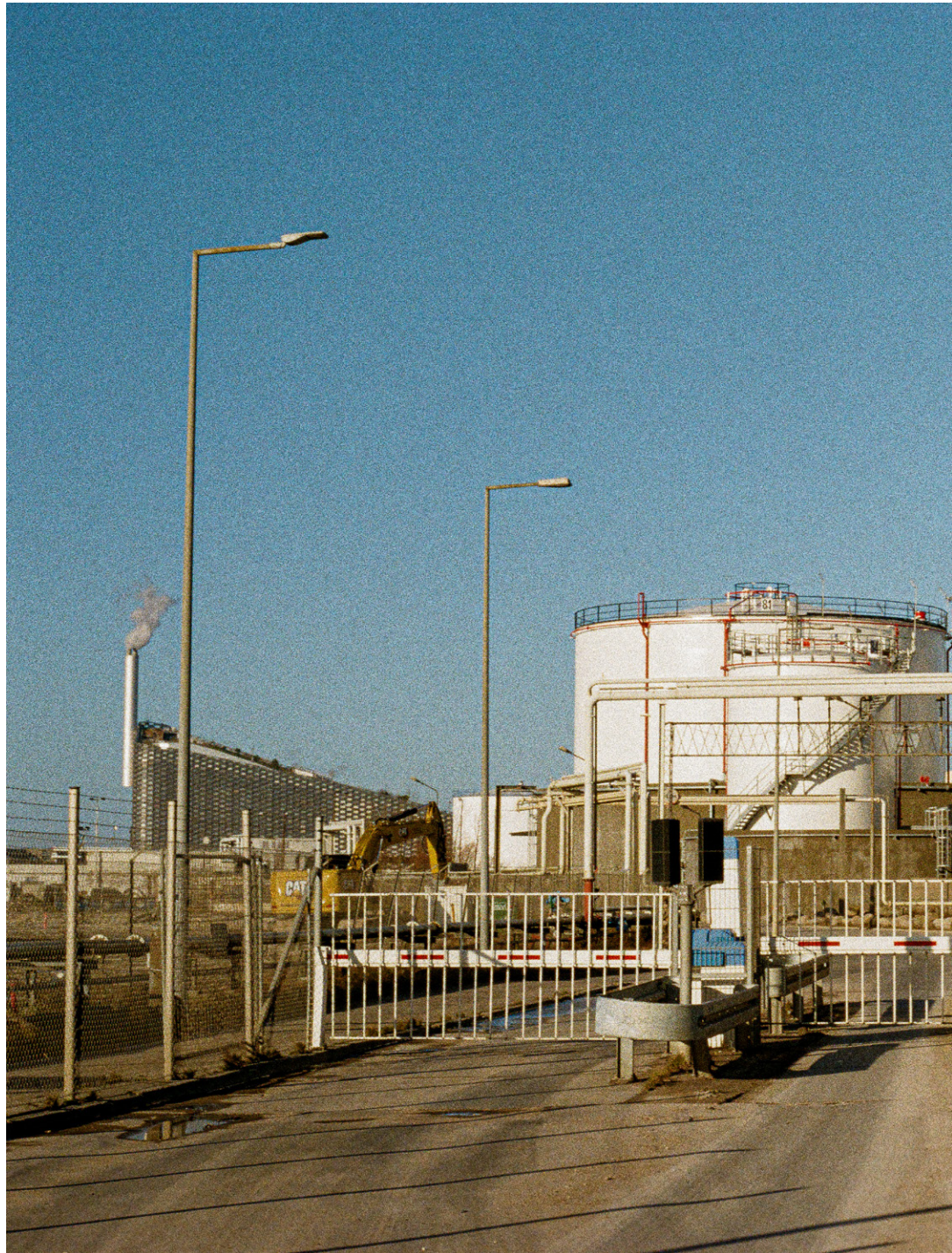
Fig. 3.3 Standing as close as one can get to the oil facilities on Petrol Island, outside the secured entrance gate. Amager Bakke, the waste-to-energy plant with rooftop 'CopenHill' can be seen in the bottom left background as the sloped roof with steam chimney. Photograph by author.
