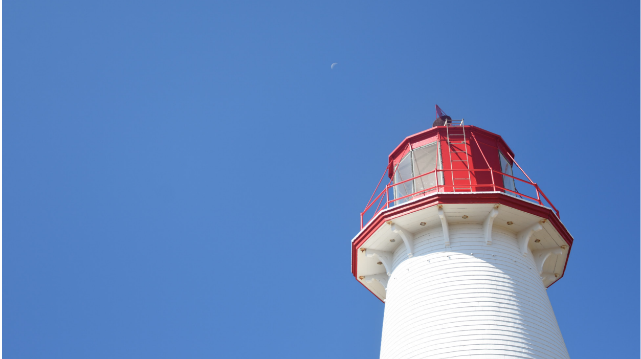
Figure 3.2 Photo of Canadian Coast Guard owned lantern room of Point Prim Lighthouse, Point Prim, PEI. 2022. Photo by Author.
