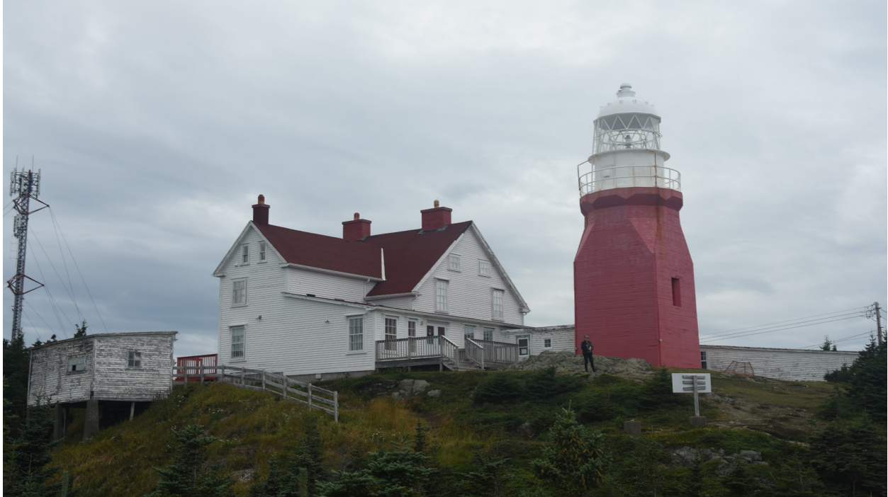
Figure 3.4 Photo depicting the weathering and state of deterioration of dwellings compared to well maintained state of Long Point Lighthouse, Crow Head, Newfoundland and Labrador. 2022. Photo by Author.
