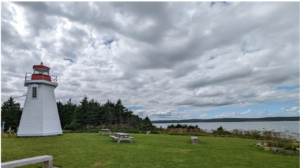
Figure 3.14 Old and new location of Gabarus Lighthouse, Gabarus, Nova Scotia. 2022. Photo by Author.
