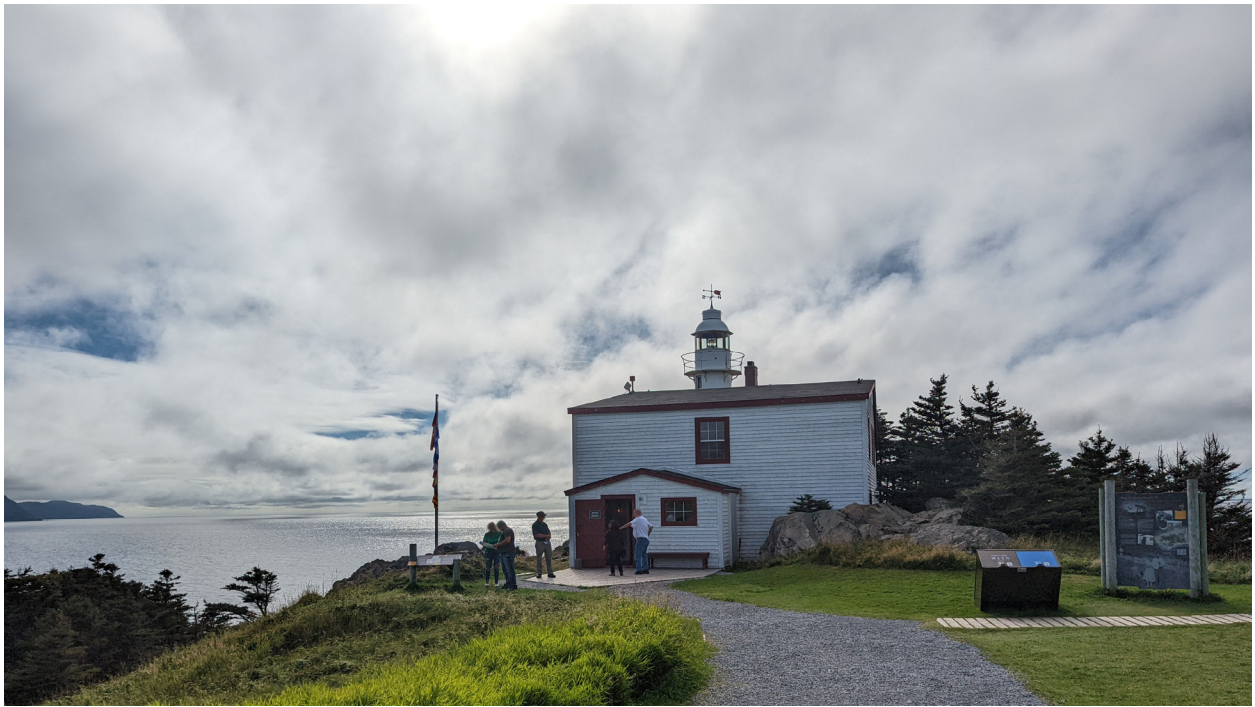
Figure 3.7 Lobster Cove Head Lighthouse in Gros Morne National Park with Parks Canada employees and signage, Rocky Harbour, Newfoundland and Labrador. 2022. Photo by Author.
