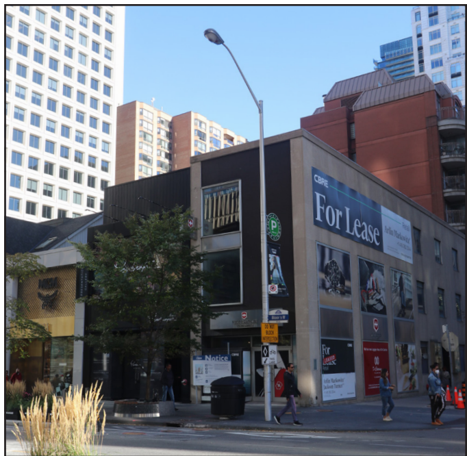
fig. 5.100 95 Bloor St West, photograph before construction
