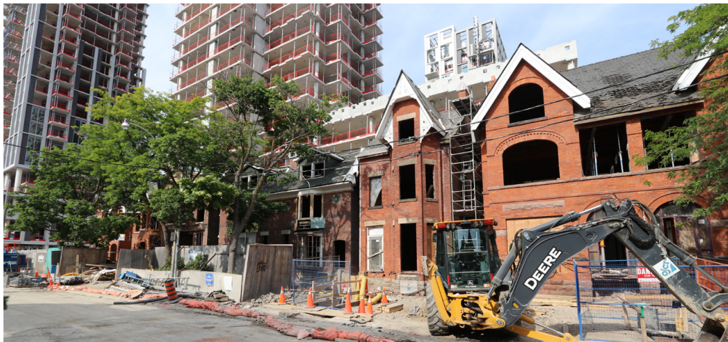
fig. 6.41 Photograph of heritage work during construction.
