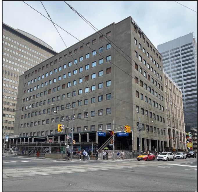
fig. 5.78 481 University Ave, photograph during construction
