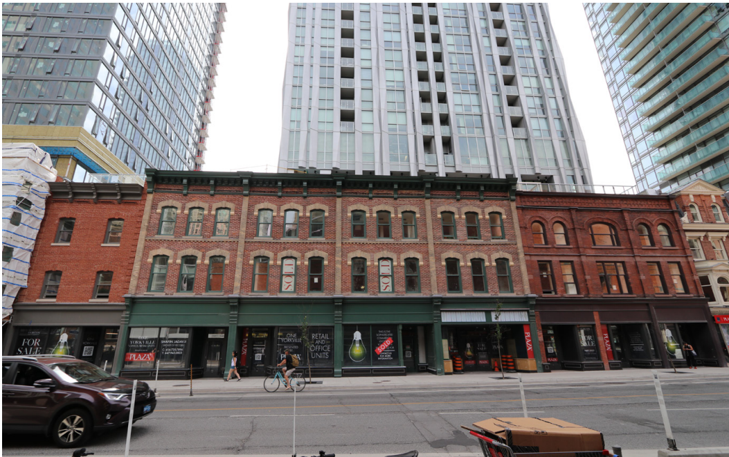
fig. 6.7 1 Yorkville nearly complete, 8 Cumberland can be seen neighbouring where the shelling continues
