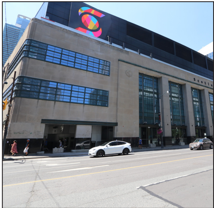
fig. 5.13 40 Bay St, photograph
