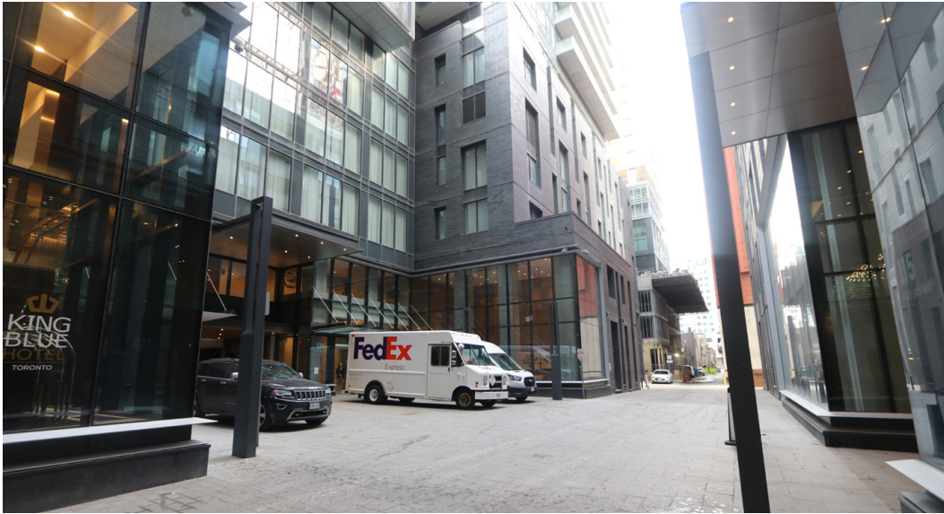
fig. 6.24 Photograph of porte cochere
