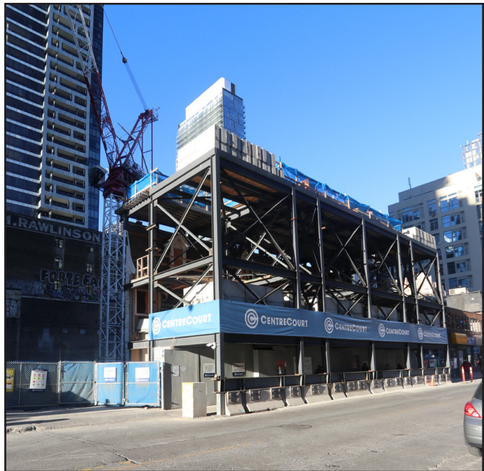
fig. 5.63 10 Wellesley St W, photograph during construction
