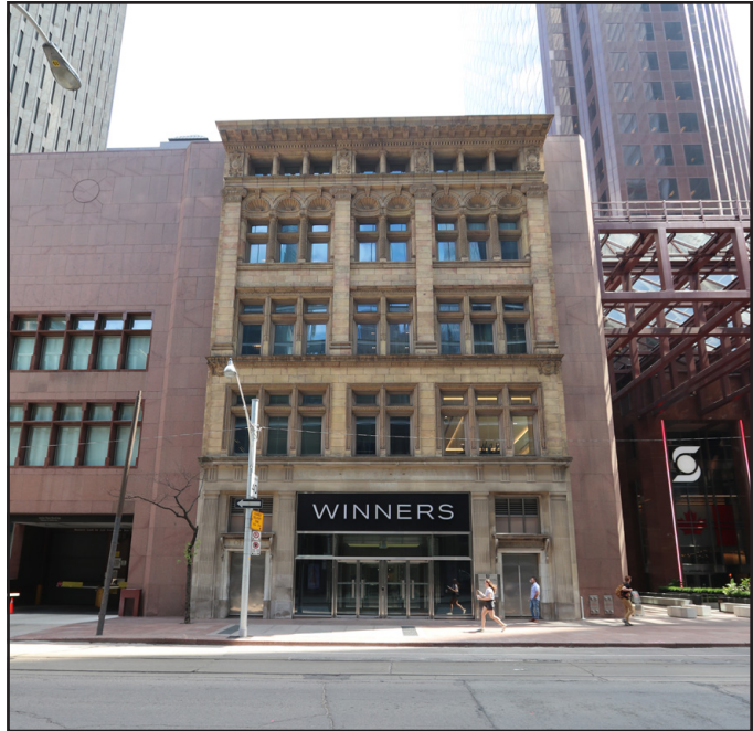
fig. 5.4 11 Adelaide St W, photograph
