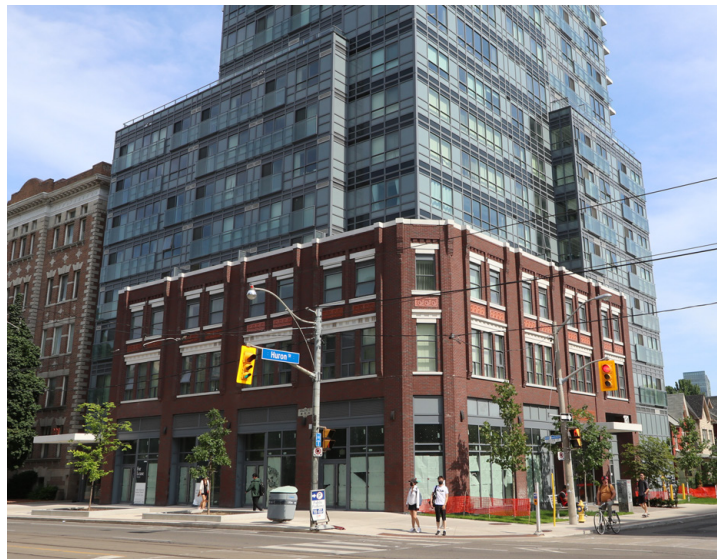
fig. 6.19 231 College St. The facade had to be rebuilt.
