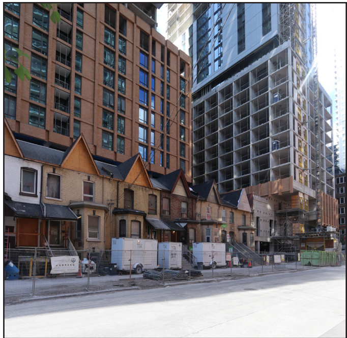
fig. 5.71 30 Widmer St, photograph during construction
