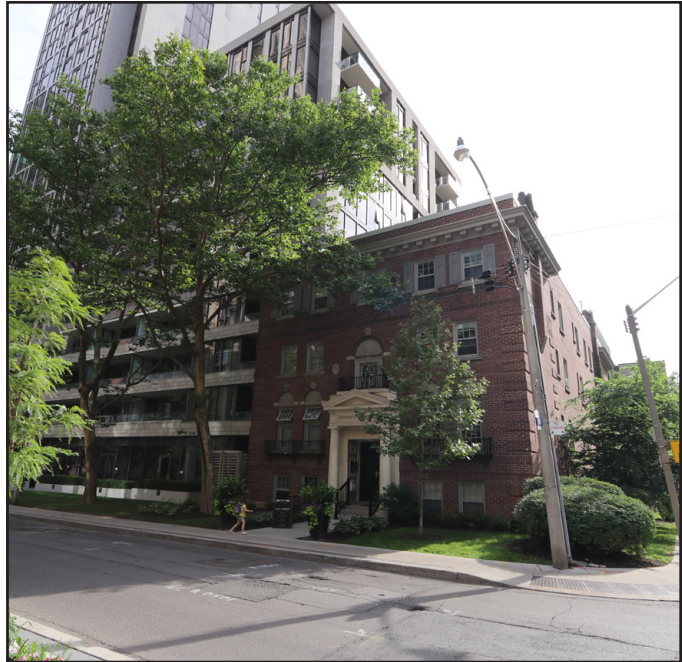
fig. 5.42 2 St. Thomas St, photograph
