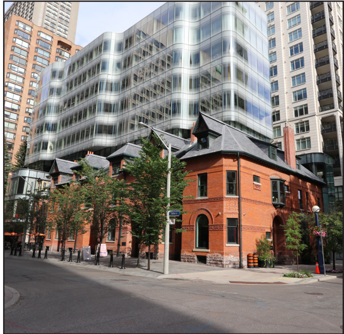
fig. 5.44 7 St. Thomas St, photograph
