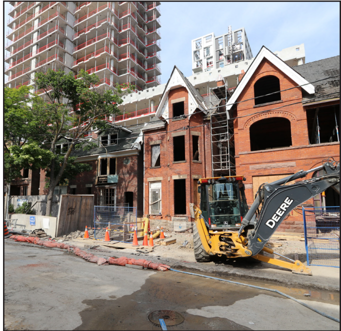
fig. 5.80 581 Bloor St W, photograph during construction
