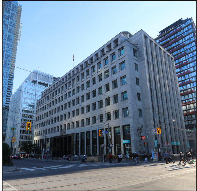
fig. 5.92 250 University Ave, photograph before construction
