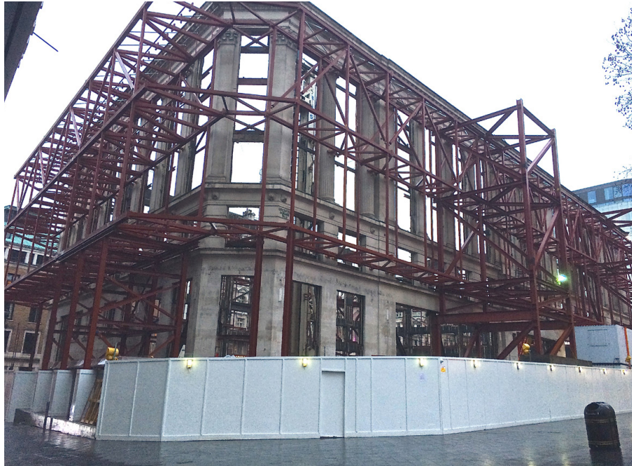
fig. 1.2 48 Leicester Square under construction, London, 2015
