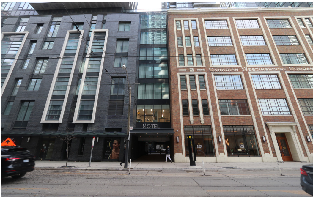
fig. 6.25 Looking at the street elevation of the podium; a pedestrian pathway cuts through where the heritage facade ends and the new podium material starts.
