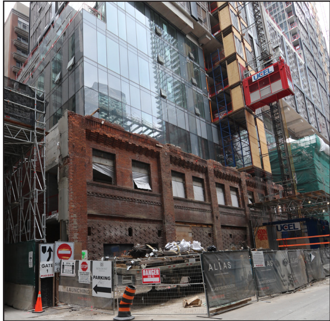
fig. 5.64 15 Mercer St, photograph during construction
