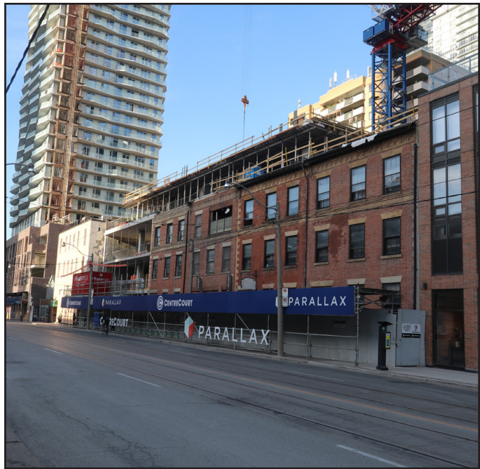
fig. 5.67 199 Church St, photograph during construction
