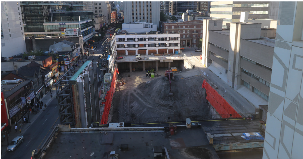
fig. 6.27 Photograph of the Concord Sky construction site
