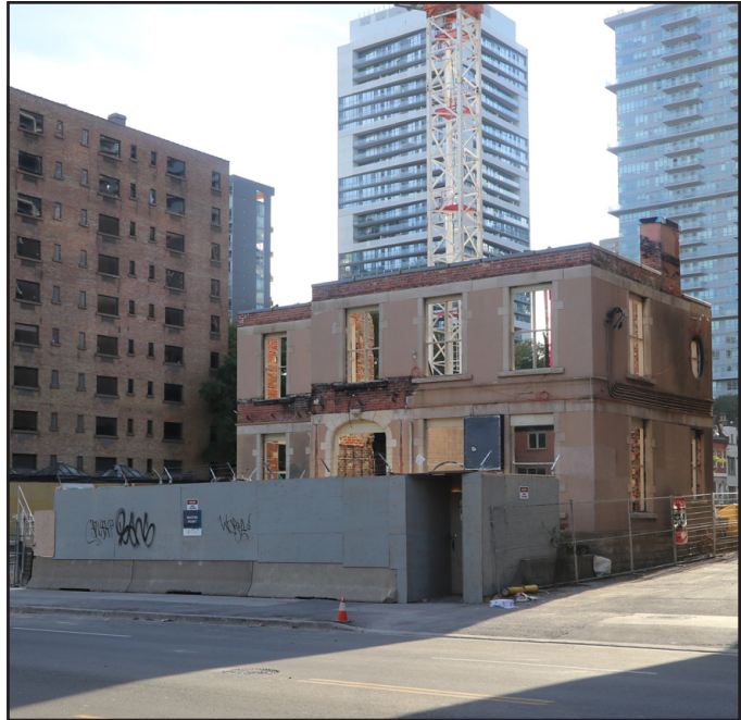
fig. 5.72 308 Jarvis St, photograph during construction
