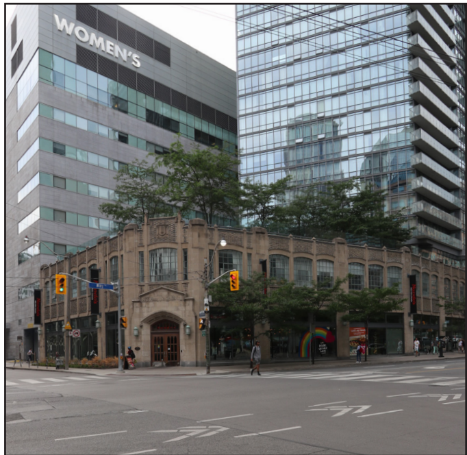
fig. 5.27 832 Bay St, photograph
