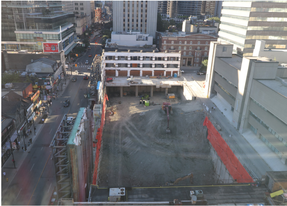
fig. 2.15 Facadism (construction site of Concord Sky)
