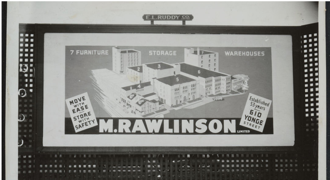
fig. 6.1 Rawlinson Limited Storage, 1937
