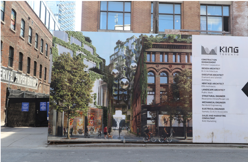
fig. 6.42 Photograph of rendering on construction hoarding.
