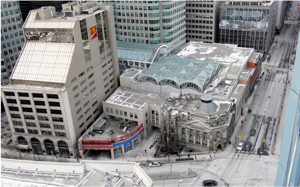
fig. 6.36 Aerial of BCE Place (Brookfield Place), 2015. Notice how the space is consolidated behind the facades, which are only fronts.
