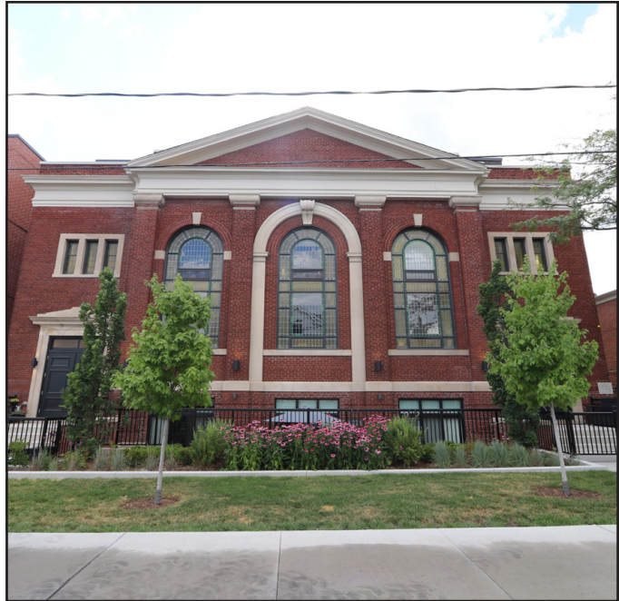
fig. 5.58 14 Dewhurst Blvd, photograph
