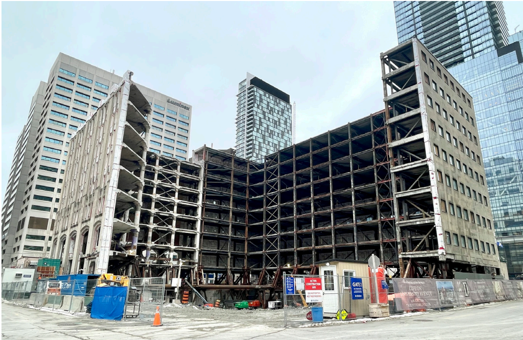
fig. 6.1 Construction site of 481 University Ave.
