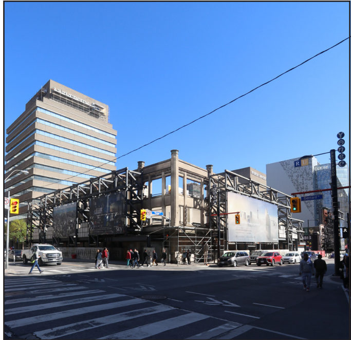
fig. 5.76 383 Yonge St, photograph during construction
