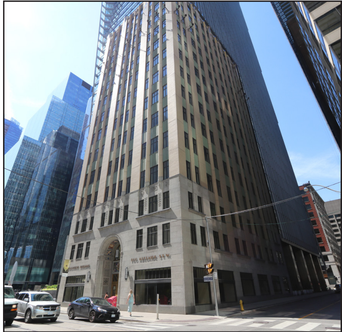
fig. 5.40 100 Adelaide St W, photograph
