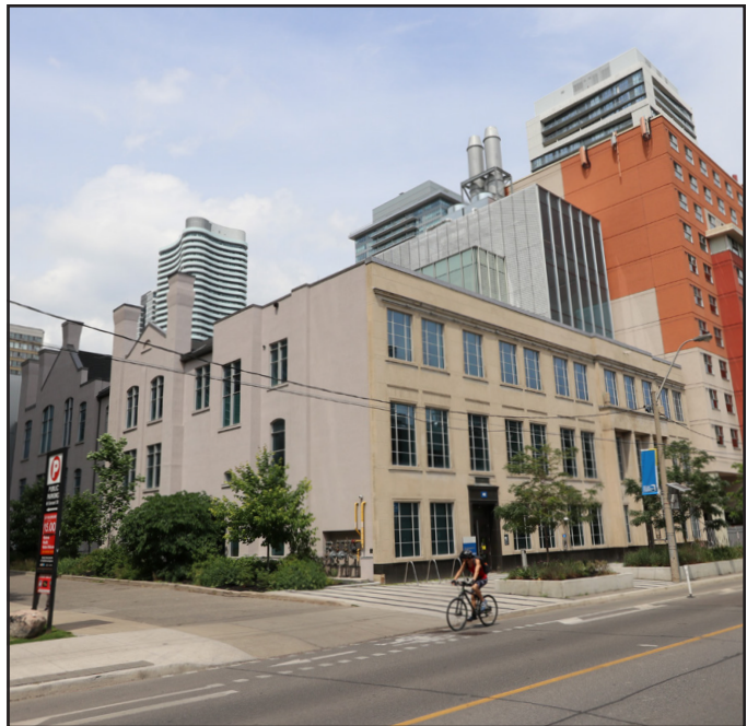
fig. 5.49 44 Gerrard St E, photograph
