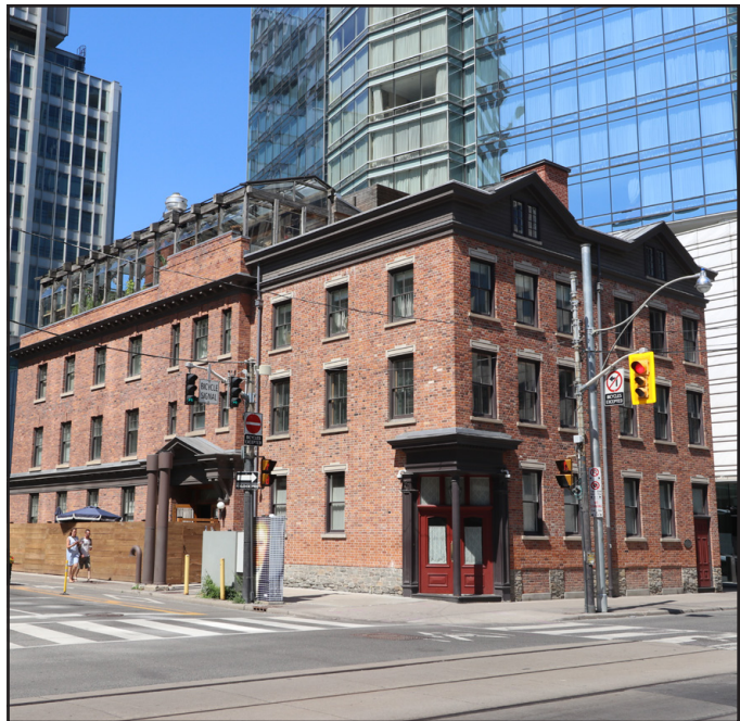
fig. 5.21 192 Adelaide St W, photograph
