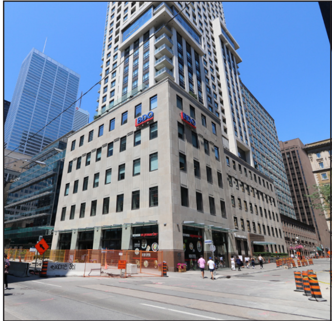
fig. 5.48 40 Scott St, photograph
