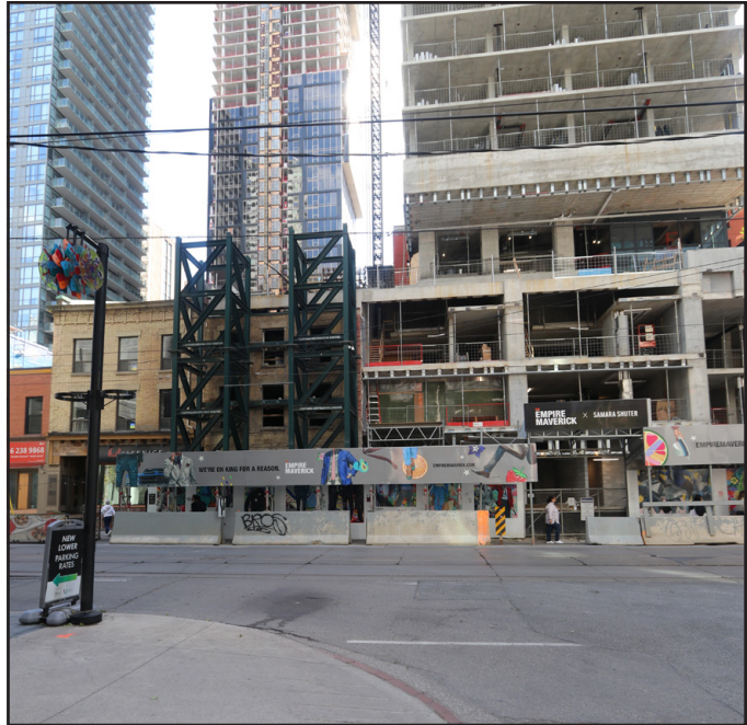
fig. 5.74 333 King St W, photograph during construction
