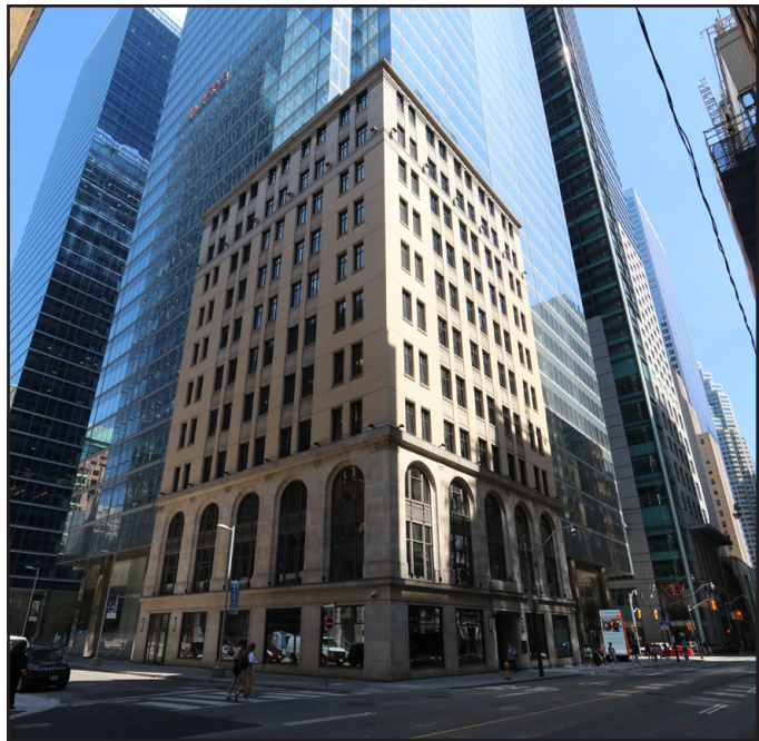
fig. 5.23 333 Bay St, photograph
