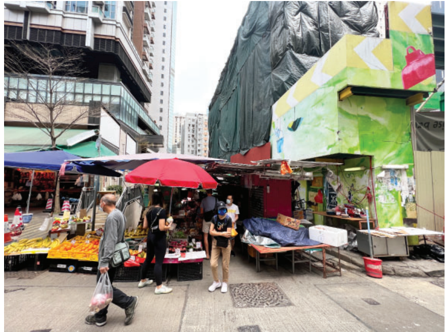
Fig.4.04 View of Graham Street Market entrance on Gage Street with towering construction surrounding the market.
