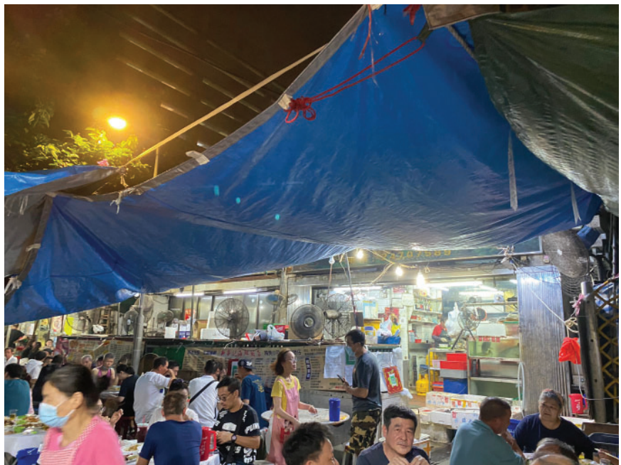
Yau San St. plastic tarp overhead awning extension from main structure.
