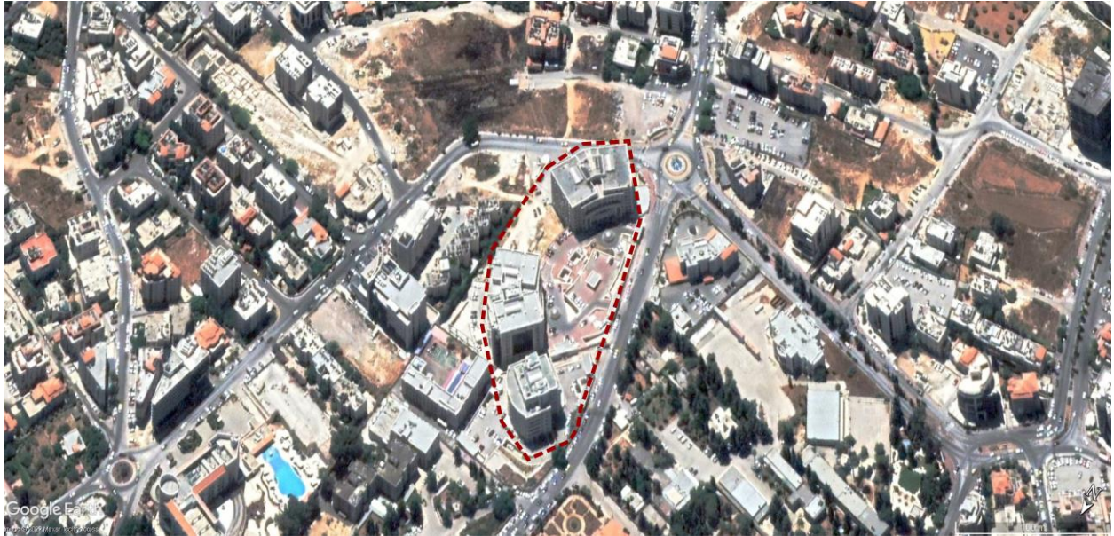
Figure 2.3: Ministerial Complex including large-scale buildings [Google Maps, author]
