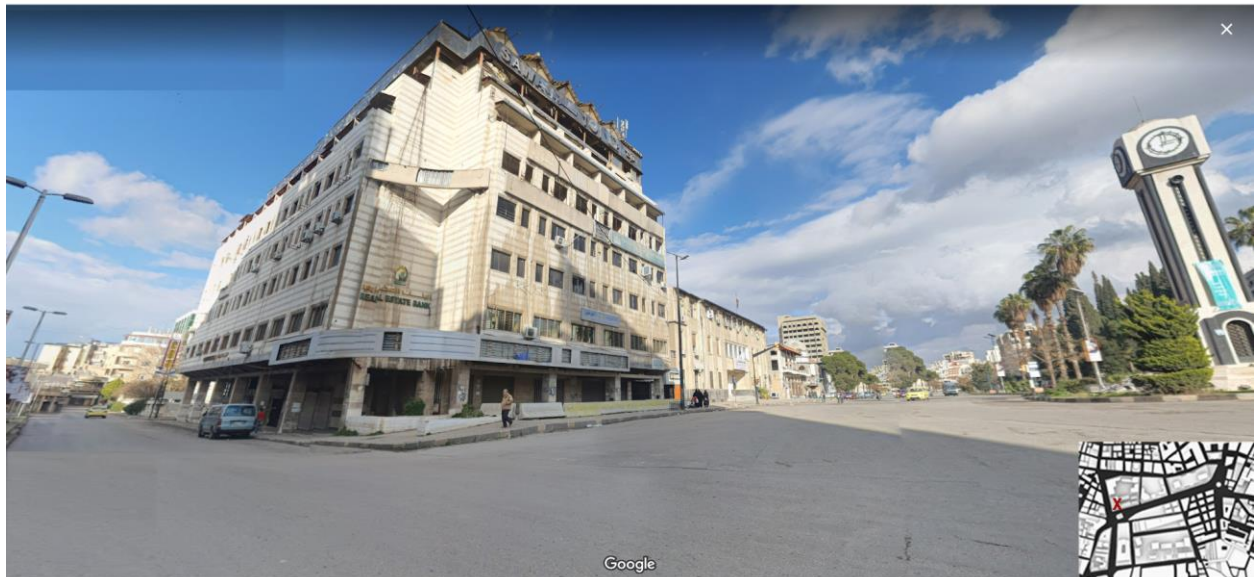
Figure 4.15: Teachers' union and Syrian real estate bank building [google maps street view]
