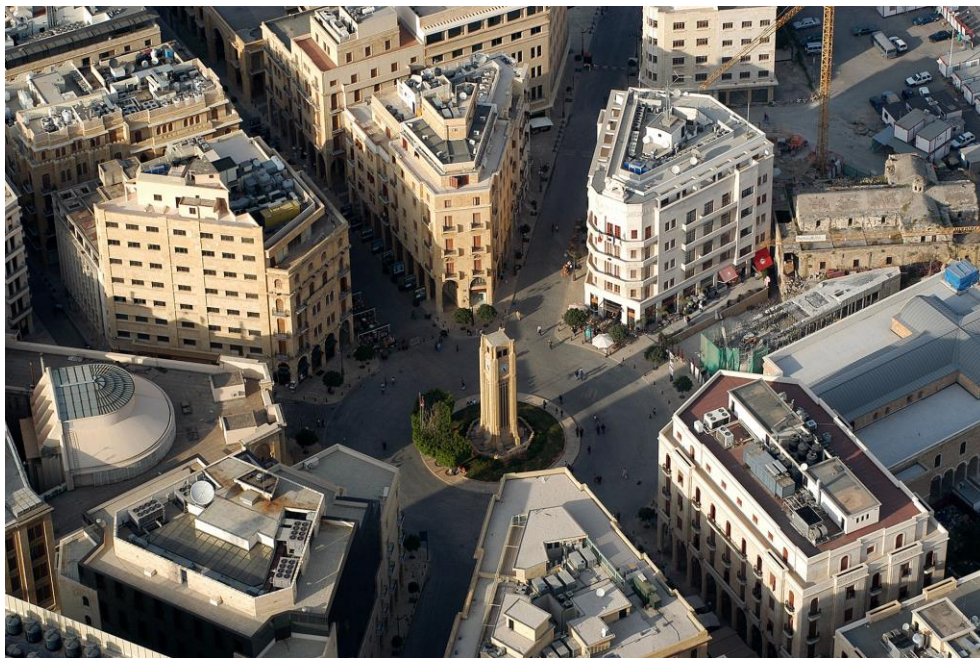
Figure 2.7: The main Square in Beirut downtown Najma Square, demonstrating a high-standard designed city center with immaculate public spaces and a homogeneous look [Solidere]
