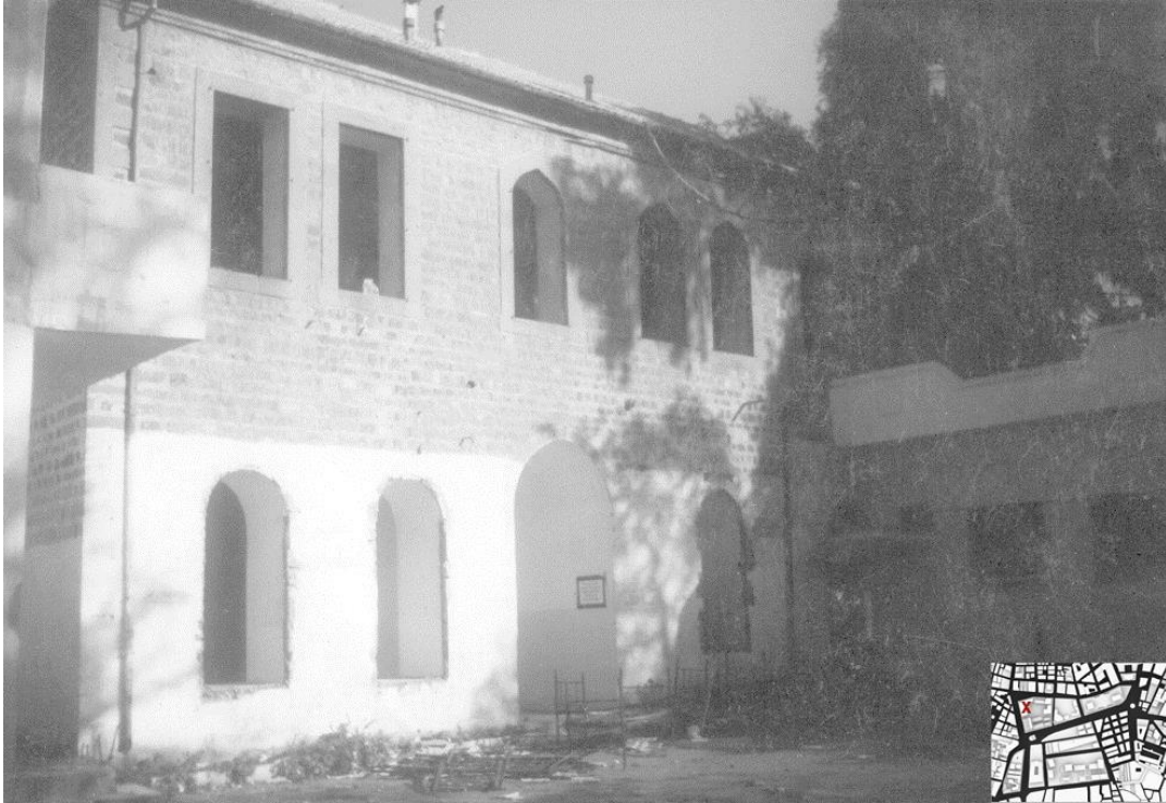
Figure 4.12: The Royal Charitable Office, constructed by the Ottomans in 1870 [Facebook.com/Museum of Old Pictures of Homs City]
