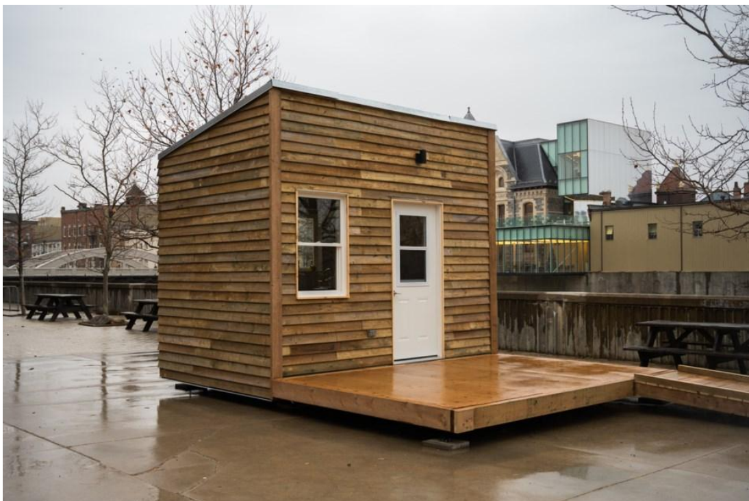
Fig. 28. v1 at its construction site at the University of Waterloo School of Architecture in Cambridge, ON. (Photo by Leilei Zhao for the design-build studio and the Tiny Homes Research Project).
