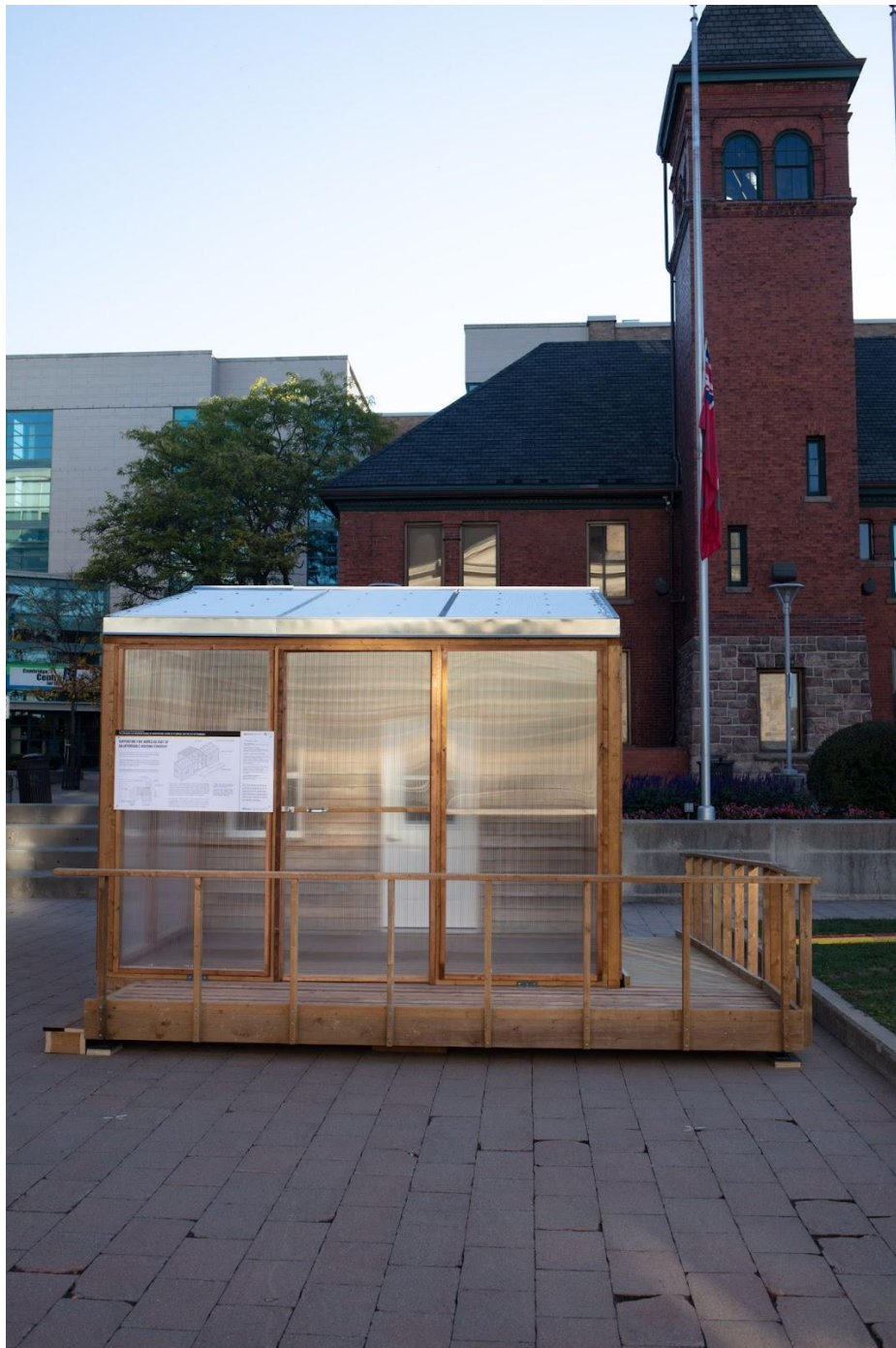
Fig. 33. The v1 prototype at City Hall, featuring the sunroom-porch, deck, and ramp. (Photo by Fred Hunsberger for the Tiny Homes Research Project).
