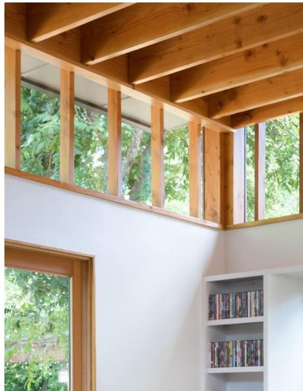
Fig. 112. A clerestory window in a home in Austin, TX. (Photo by Whit Preston, Design by Murray Legge Architecture, 2015, https://www.murraylegge.com/skyview )
