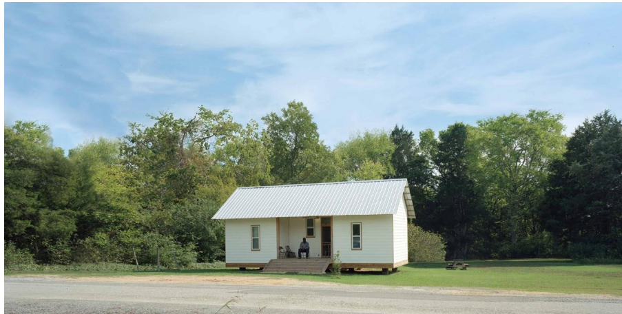
Fig. 25. "Mac's Home" in Alabama by Rural Studio. (Photo by Timothy Hursely, Design by Rural Studio, http://ruralstudio.org/front-porch/product-line-houses/ ).
