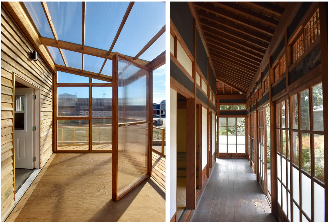
Fig. 74. The v1 polycarbonate panels are similar to the shoji screens used in Japanese architecture. (Photo on left by author, photo on right retrieved from: https://en.wikipedia.org/wiki/Shoji#/media/File:Yoshimatsu02.jpg ).
