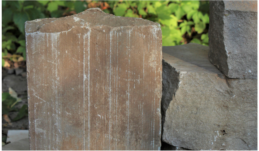
Fig. 2.21 Close-up of Queenston Limestone with saw marks, image by author.
