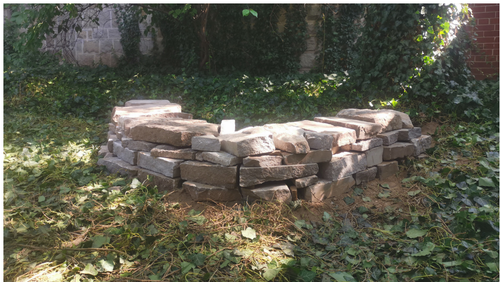
Fig. 2.1 Dry-stone stacked wall practice at Willowbank workshop, image by author.
