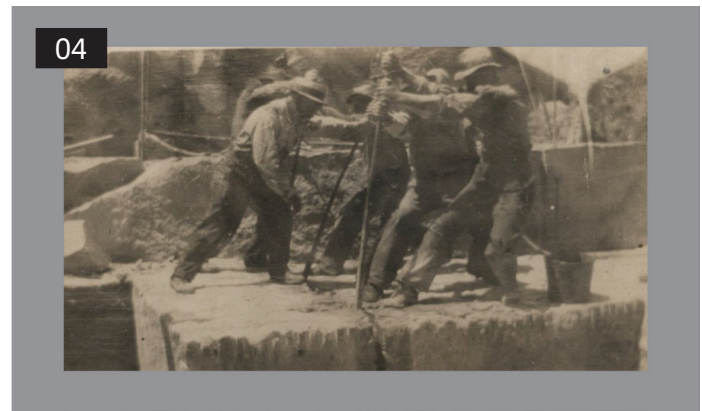
Fig. 1.13 Workers of the Queenston Quarry Company, workers splitting mill blocks with crow bars, Niagara-on-the-Lake Public Library, Collection of Alan Clifford, NOTLPL00227-03 to NOTLPL00227-11.
