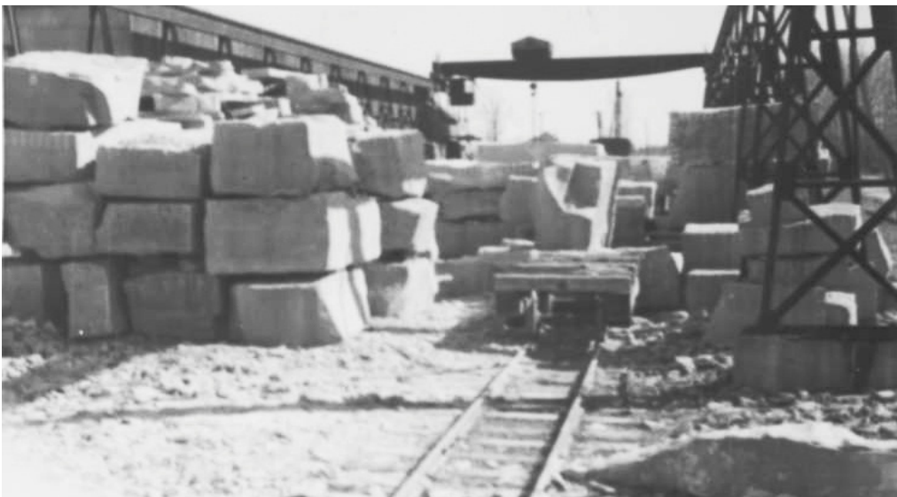
Fig. 1.21 Queenston Quarries, showing derricks transporting limestone to Queenston quarry stone yard, Gonder, Niagara-on-the-Lake Public Library Local History Collection, Francis J. Petrie Collection, D417697.
