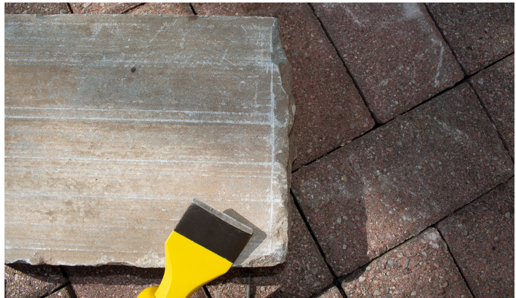
Fig. 2.19 Shaping stones with a stone chisel, image by author.
