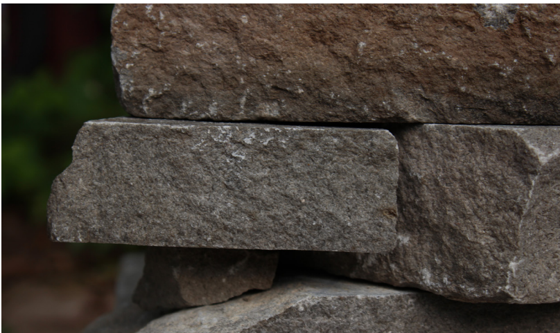
Fig. 2.17 & Fig. 2.18 Using rock shims as shims to support stones, image by author.
