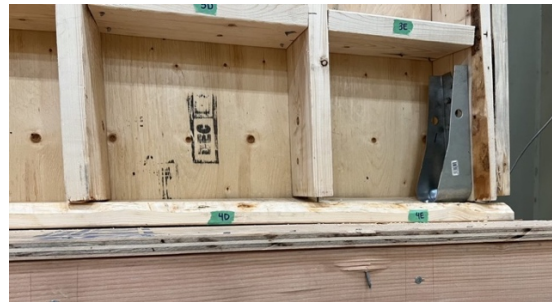
h) Stud nail withdrawal from bottom plate
