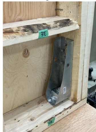
f) Right side hold down (no visible cracks in bottom plate)
