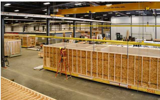
(a) NRB Modular Solutions Off-Site Construction
