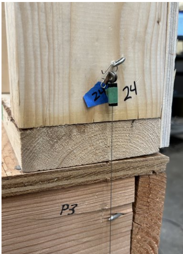
d) Right side hold down (no significant growth of crack from cyclic test 1)
