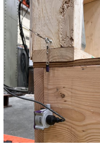
c) Left side hold down (near 4A) panel crushing base
