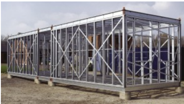
(a) Steel Framed Volumetric Module
