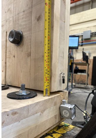
b) Right side connection uplift (note base crack)
