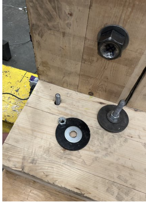
b) Left side connection (no visible damage around steel bracket/bolts), upgraded washers were sufficient for test)
