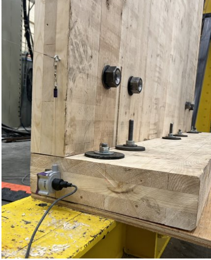
a) Left side connection (no visible damage)
