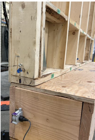
d) Left side hold down (note crack in bottom plate)
