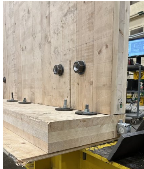
d) Right side connection (no visible damage)
