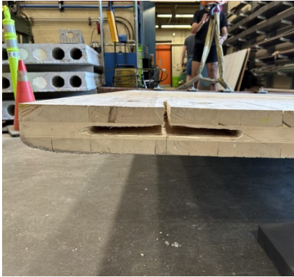
a) Left side connection slot (no visible damage)
