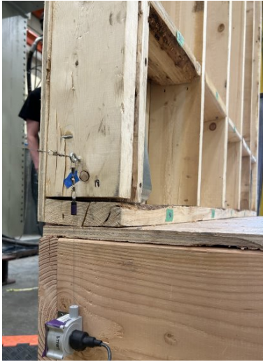
a) Left side hold down (stud lifting & crack in bottom plate worsening)
