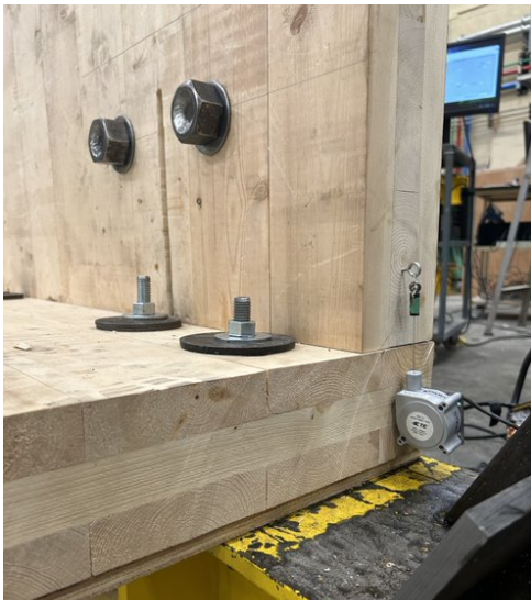
c) Right side connection (no visible damage)
