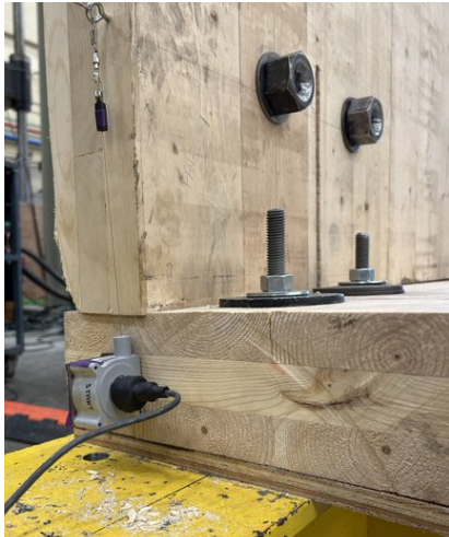
d) Left side connection (note slight crushing on base under panel)
