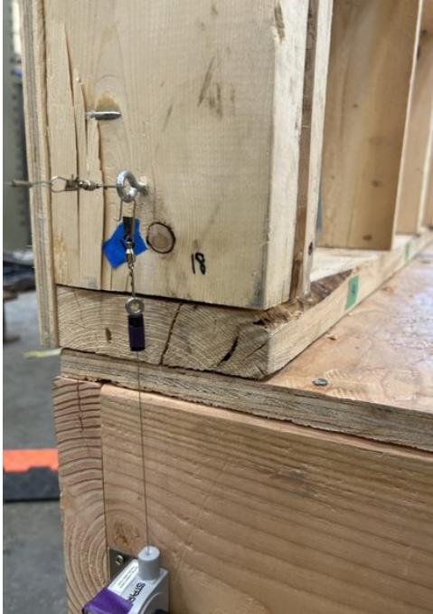
a) Right side hold down (no significant additional damage since previous cyclic test)
