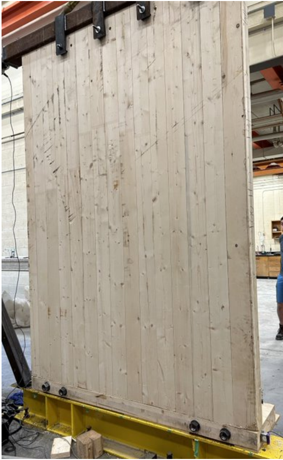
b) Back of panel (no visible damage except crushing along bottom edge/corners)
