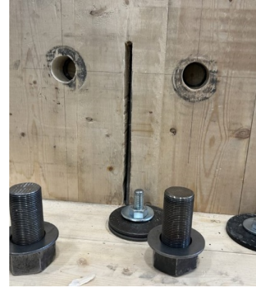
c) Right side connection with bolts removed
