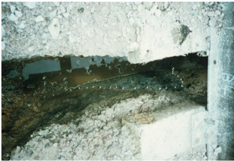
Figure 1.3: Failure mechanisms of railway subgrades: (a) Progressive shear failure in railway foundation [141, 142], (b) Subgrade attrition with mud pumping [194, 262], and (c) Excessive Plastic Deformation [139]
