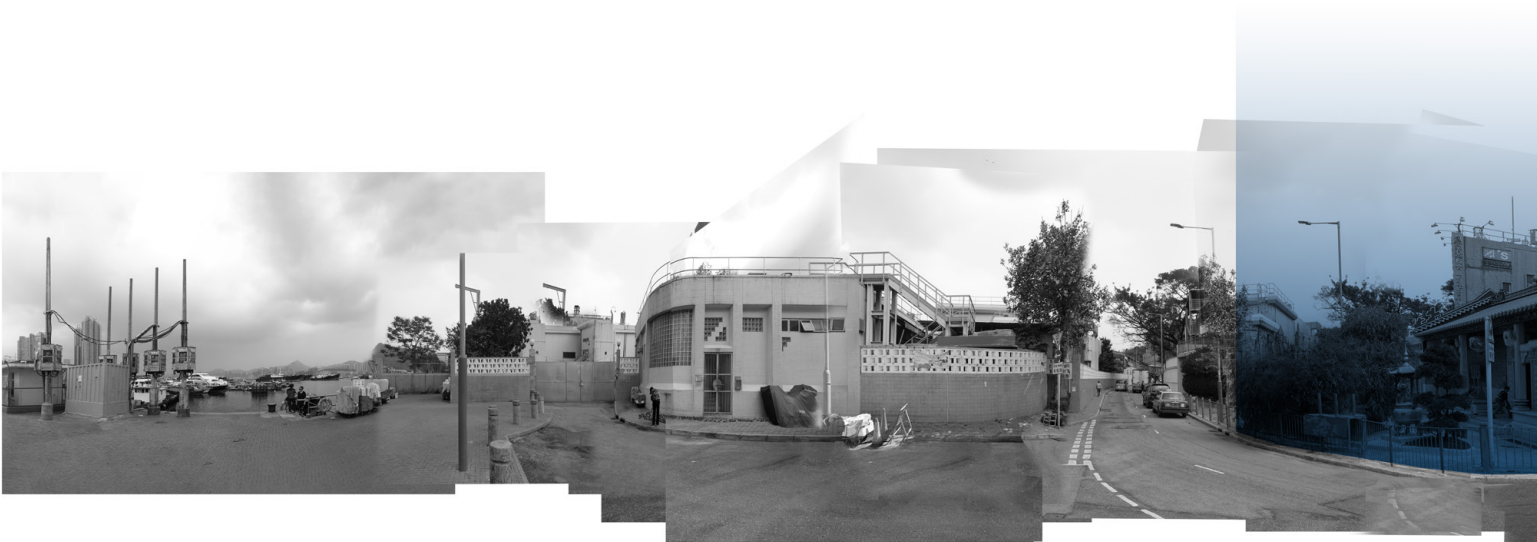
Fig. 6.71 Site 3 Elevation during Off-Season
