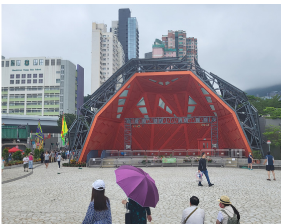
Fig. 5.34 Adjacent Eastern District Cultural Square
