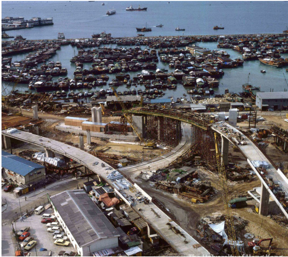
Fig. 4.12 Island Eastern Corridor Under Construction, 1980s
