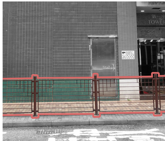
Fig. 6.29 Special Fences along parts of Shau Kei Wan Main Street East
