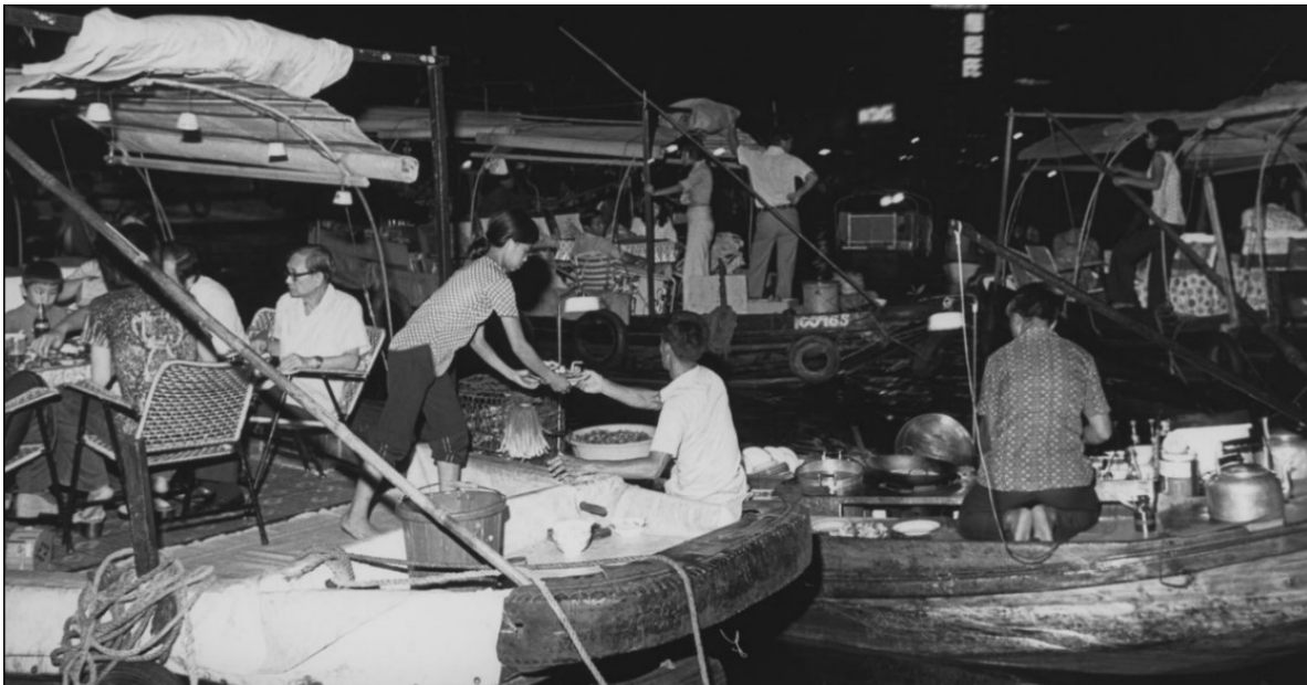
Fig. 2.5 Floating Kitchen in Causeway Bay Typhoon Shelter, 1974
