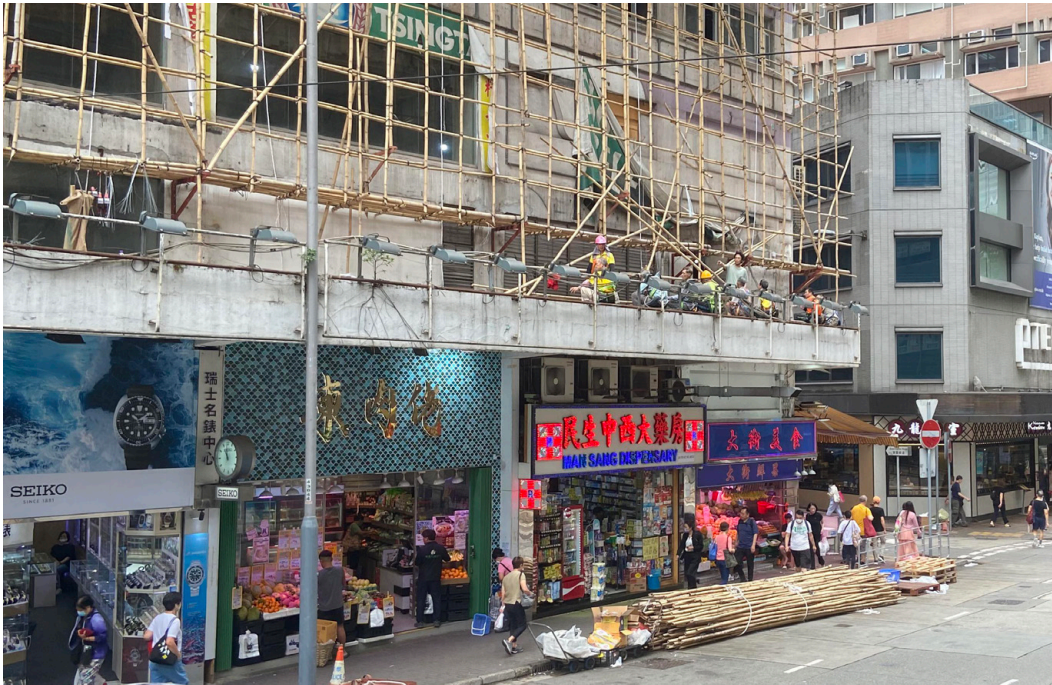
Fig. 3.12 Setting up Bamboo Scaffolding in Hong Kong, 2023
