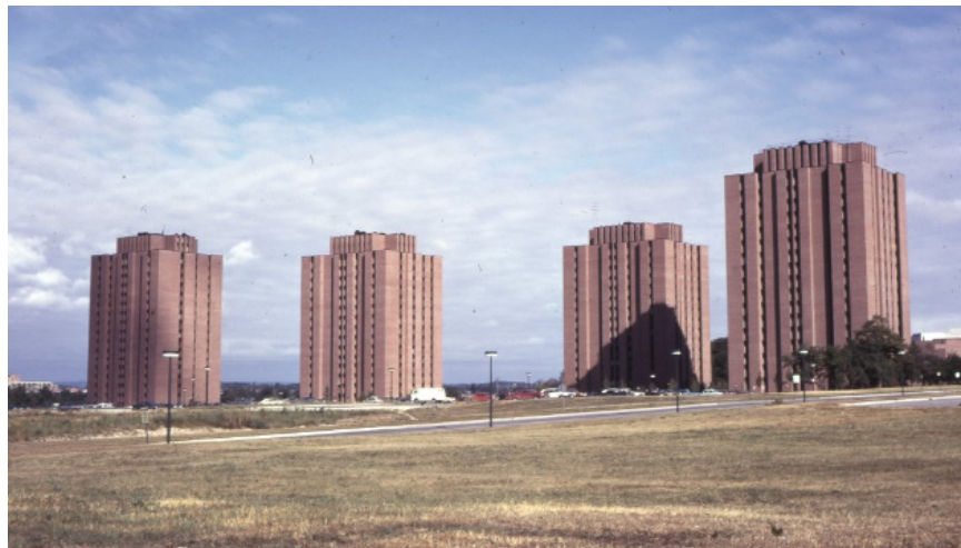
Fig. 1.2 York University Graduate houses. Examples of large-capacity student residences in the 1960s.
