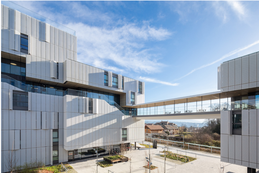
Fig. 1.35 View of the promenade and bridge.
