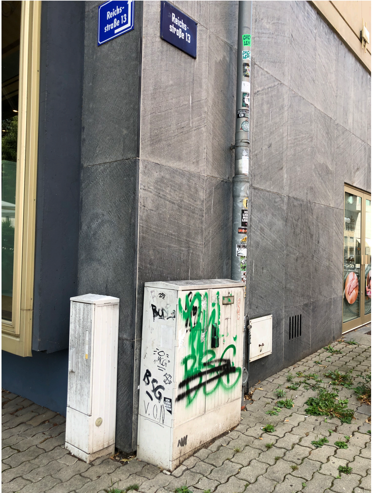
Figure 20. Drain pipe and power box with Chemie.
