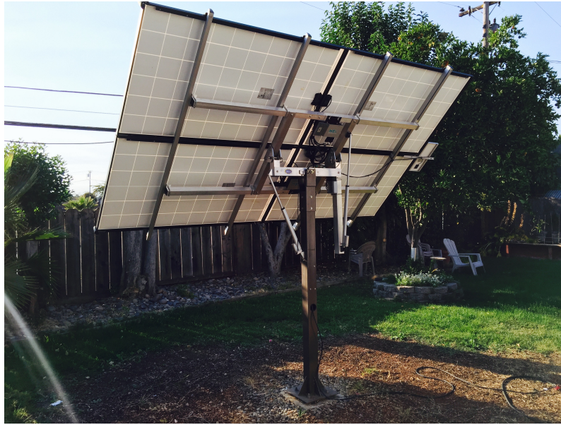
Figure 2.2: Pole mounted solar panel with dual-axis solar tracking capabilities. (© 2016 Adsala, original shared under CC BY-SA 4.0 )
