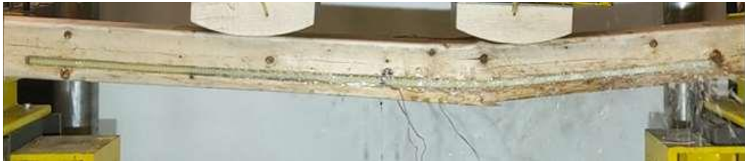
(c) FRP resin failure
