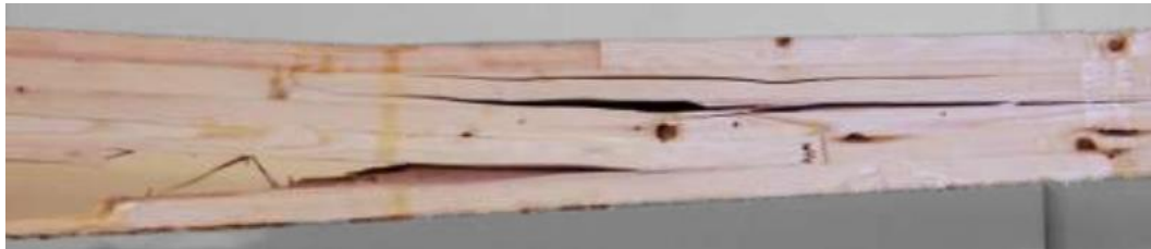
(c) Crack detail (front view)
