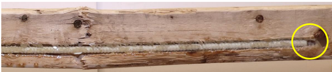
(e) Crack and slip detail (front view)
