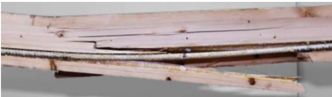
(e) Crack detail (front view)
