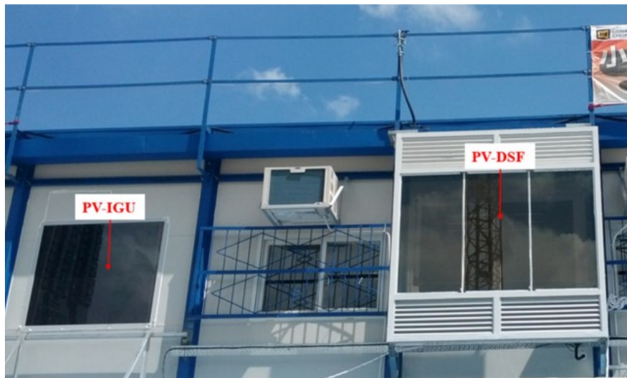
Figure 43 Test bed on the south facing facade in Hong Kong for the PV-DSF and the PV-IGU various performance comparison [48].
