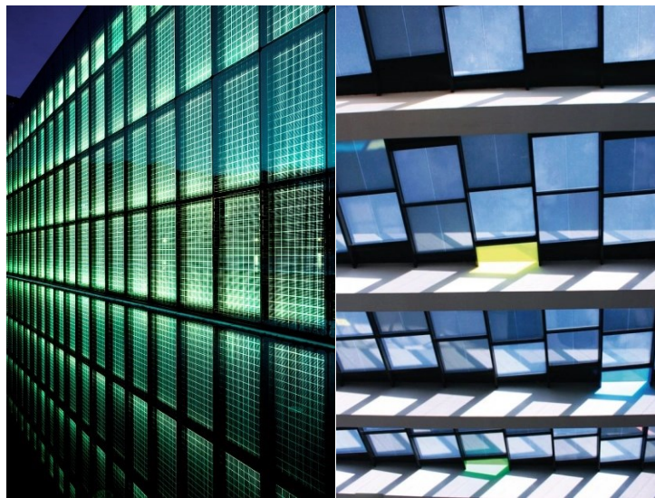
Figure 6 c-Si based BIPV curtain wall (left, Source: Ertex Solar); a-Si thin film BIPV (Right, Source: Onyx Solar)
