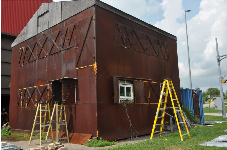
Figure 3.1: External view of the burn house structure.
