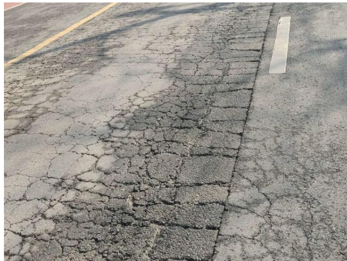
Figure 2. Alligator Cracking
