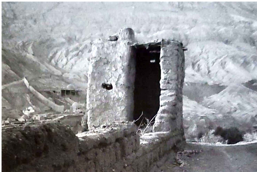
Fig.3-1-29 Dry toilet on roof. 72
