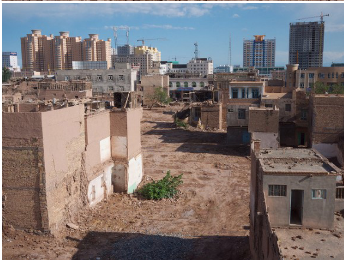
Fig.4-3-8 Old City of Kashgar under demolition in 2014. In the distance, concrete high-rises are under construction. Photograph by Far West China. 7
