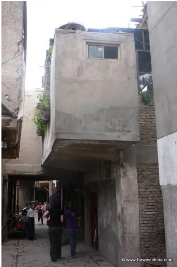
Fig.3-1-31 Overhung structures built over street, known as “cross-street-houses” in the Old City of Kashgar. 82
