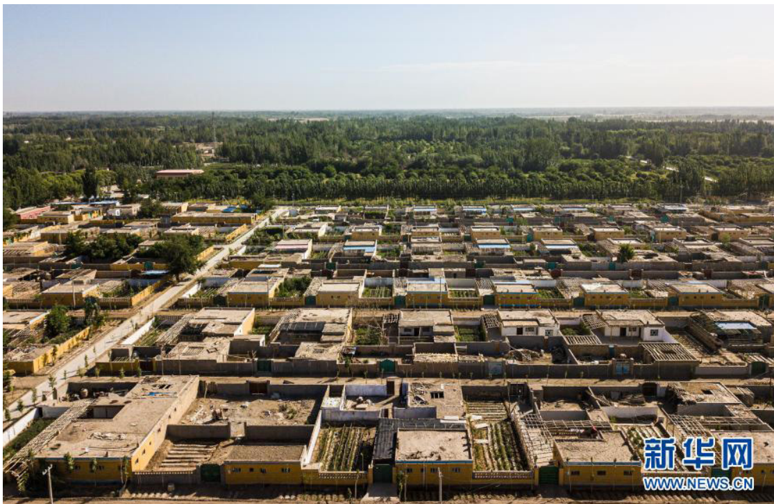
Fig.4-2-12 Fu Min An Ju Housing in Kuotandun Village, Ishkuli Township, Shache County (莎车县伊什库力乡阔坦墩村), Xinjiang. Drone photograph by Wang Fei on May 22, 2020. 31
