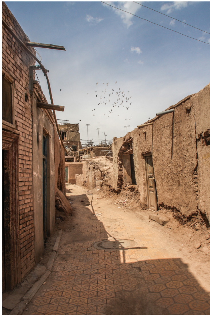
Fig.4-3-9 The Old City of Kashgar in various stages of demolition in summer of 2014. Photograph by Silvia. 9
