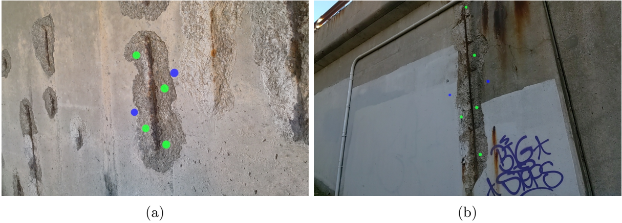
Figure 3.11: Seed points selected on SA in (a) and SB in (b): The points inside and outside spalling regions indicate positive and negative seed points, respectively. These images were captured on the HoloLens 2.
