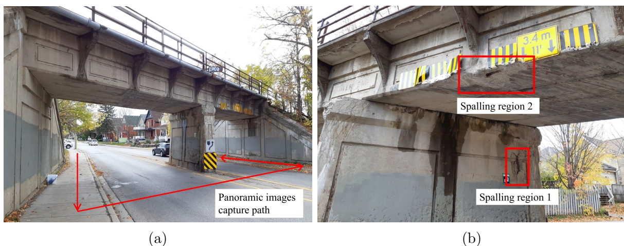
Figure 5.5: Test bridge structure: (a) a path for collecting panoramic images and (b) two spalling regions at the side and top of the bridge abutment.
