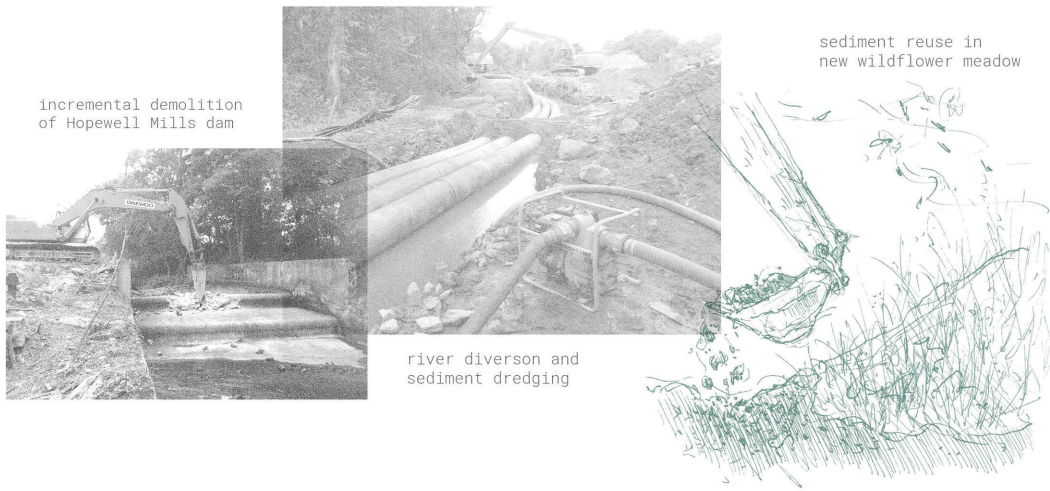
Fig. 4.25 Dam removal process at the Hopewell Mills site.
