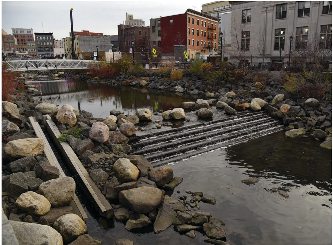
Fig. 4.8 An eel and fish ladder provides connectivity at a small weir along the Saw Mill River in Yonkers, New York. Photograph by Nathan Kensinger, 2016.
