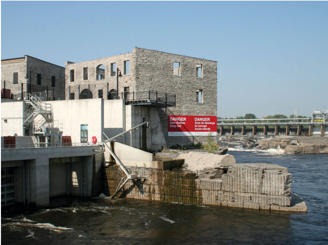
Fig. 4.16 One of the eel ladder intakes mounted to Generating Station #5 with steel supports, August 2023.
