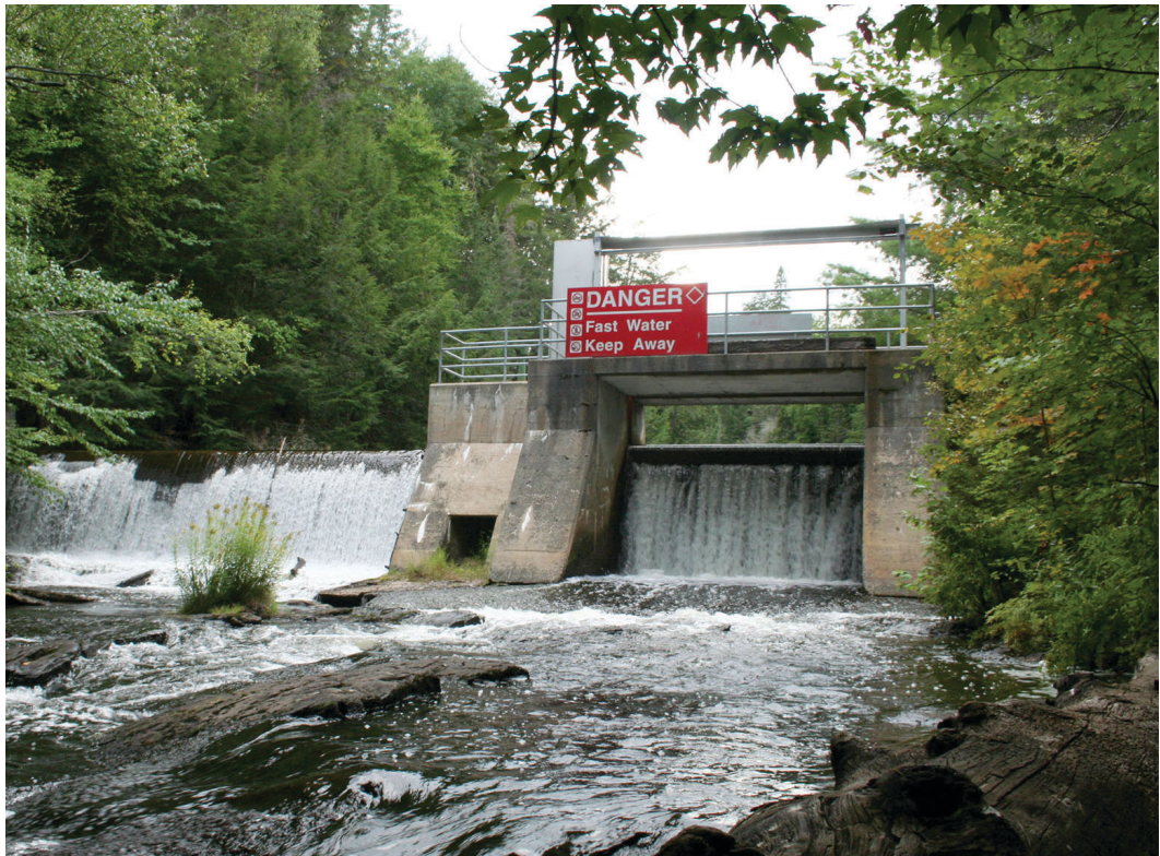
Fig. 4.4 The current concrete stoplog dam at Cache Lake, August 2023. Repairs to the dam's spillover weir are visible to the left of the view.
