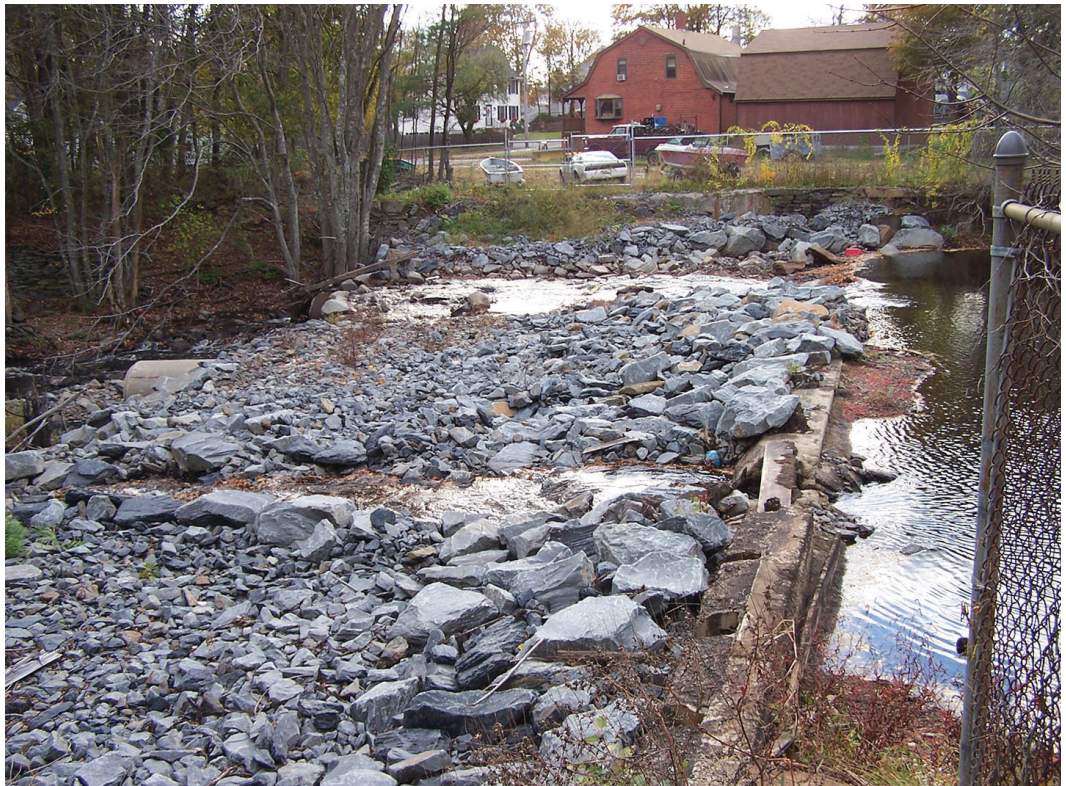
Fig. 4.23 Boulders piled against the aged Whittenton dam after its near failure to prevent collapse. Photograph by the Massachusetts Division of Ecological Restoration, 2010.
