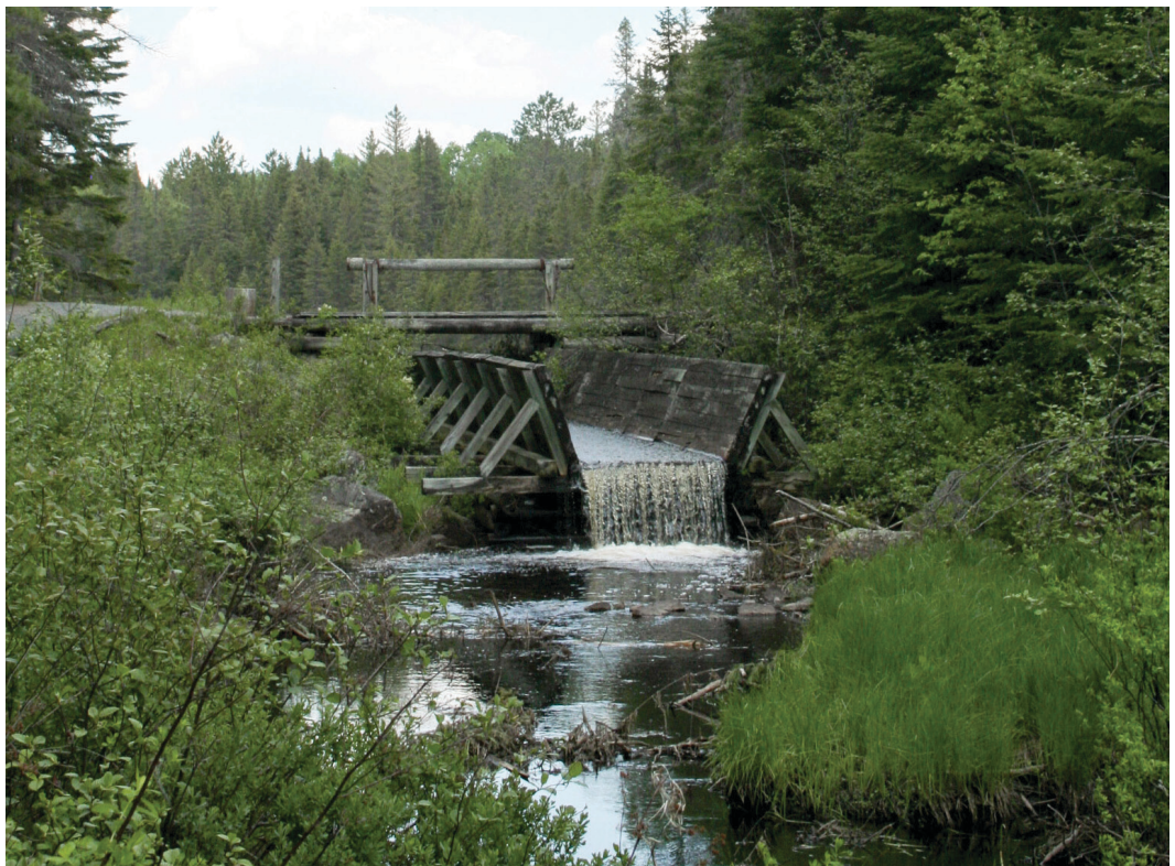
Fig. 2.4 A display wooden logging dam and chute at the Logging Museum's outdoor exhibit, May 2023.
