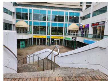
Fig. 3.7 2024 photo of Chinatown Centre Mall. Glass walls and modern style.
