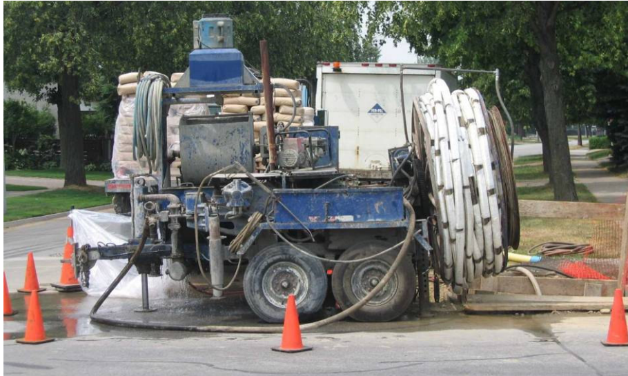
Figure 2-4: Pumping machine where mortar is mixed and pumped into the watermain.
