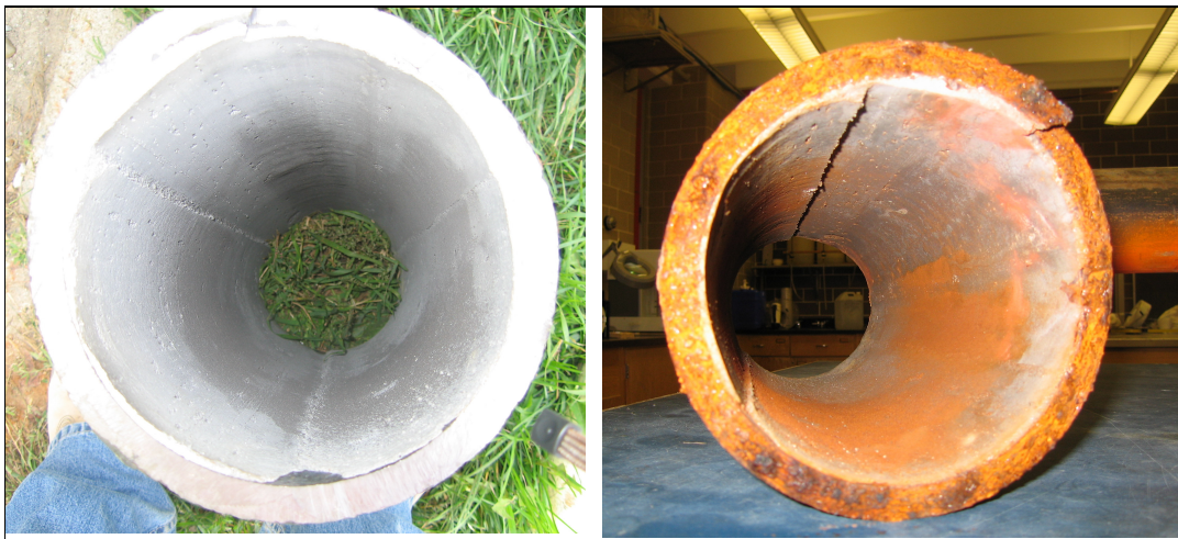
Figure 4-7: Pipe section #1 at collection (left) and prior to testing.
