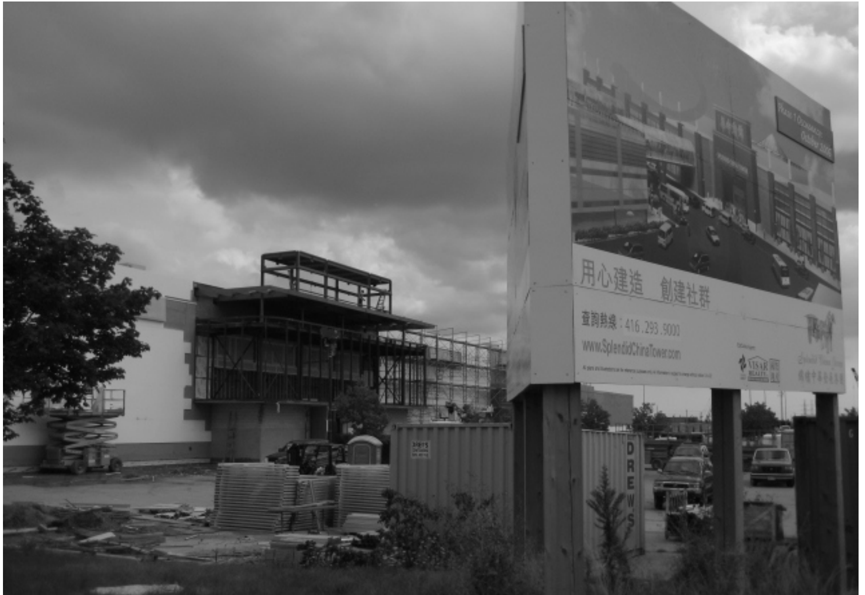
Fig. 5.103: Construction Site of Splendid China Tower Over Former Canadian Tire Store
