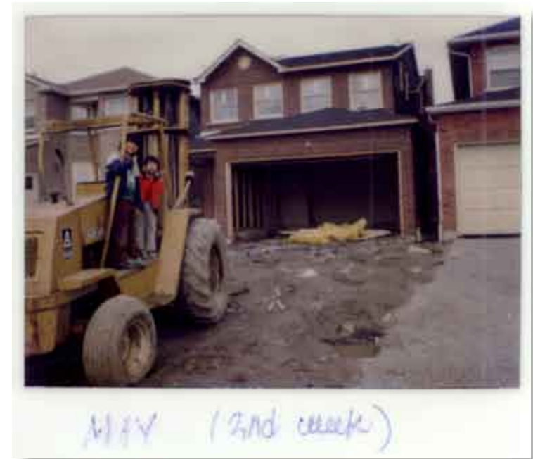
Fig.5.78: Photo of Sanvictores family home in second week of construction
