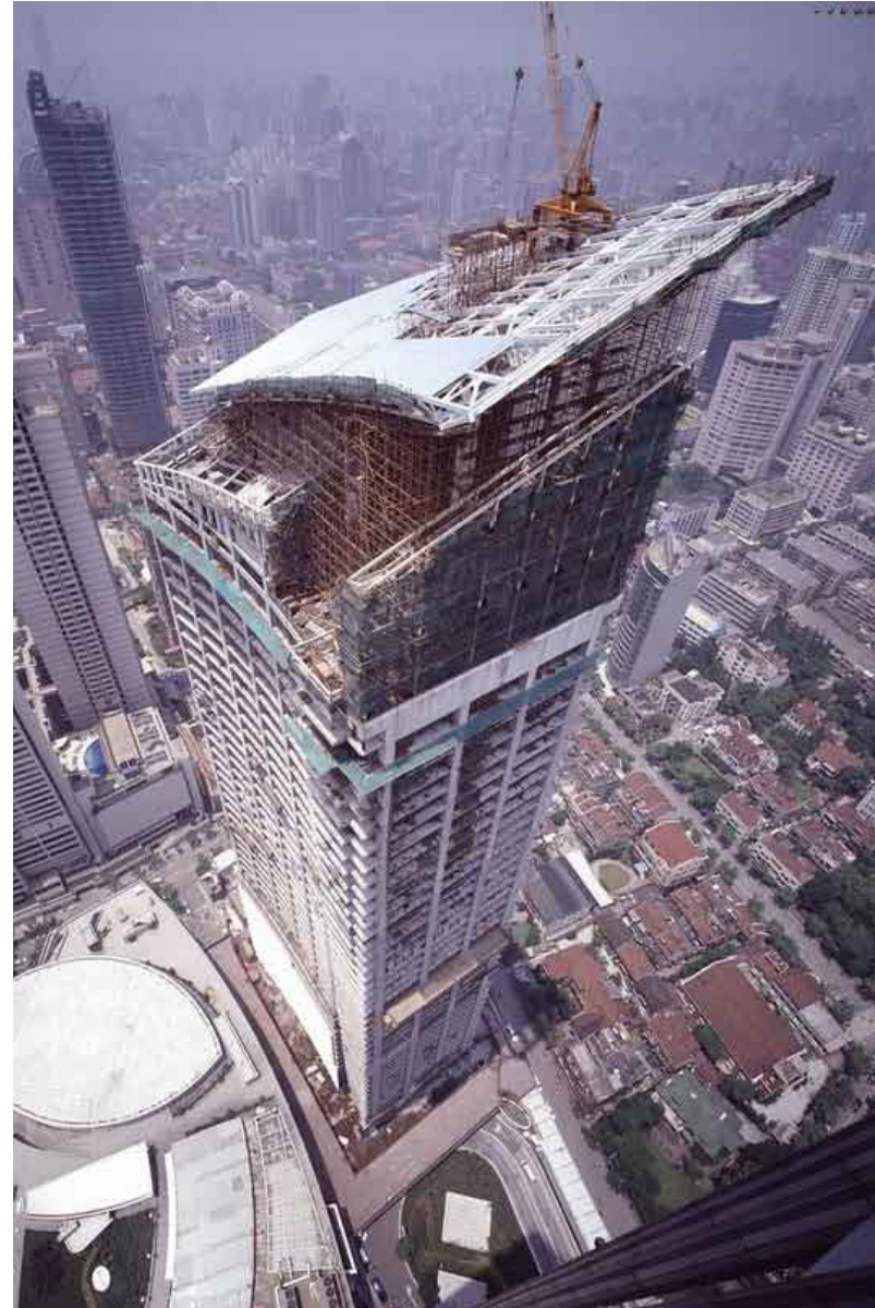
Fig. 3.19: Construction Photo of Plaza 66 Phase 2 Tower, Source: www.skyscrapercity.com
