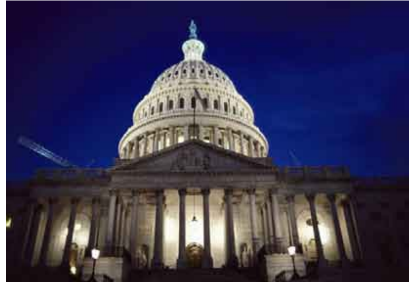
Fig. 3.38: U.S. Capitol Building, Washington DC
