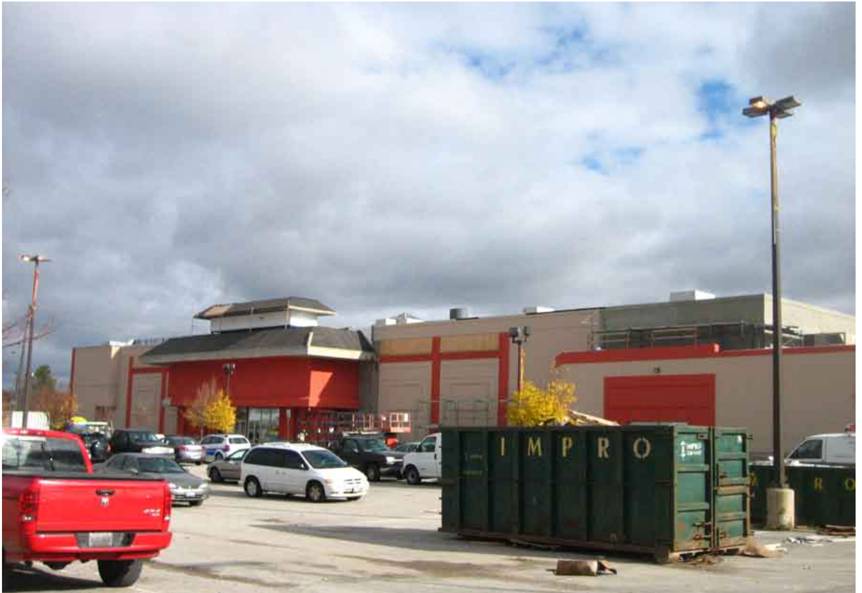
Fig. 6.85: View of Splendid China Tower in Final Stages of Construction, November 2006
