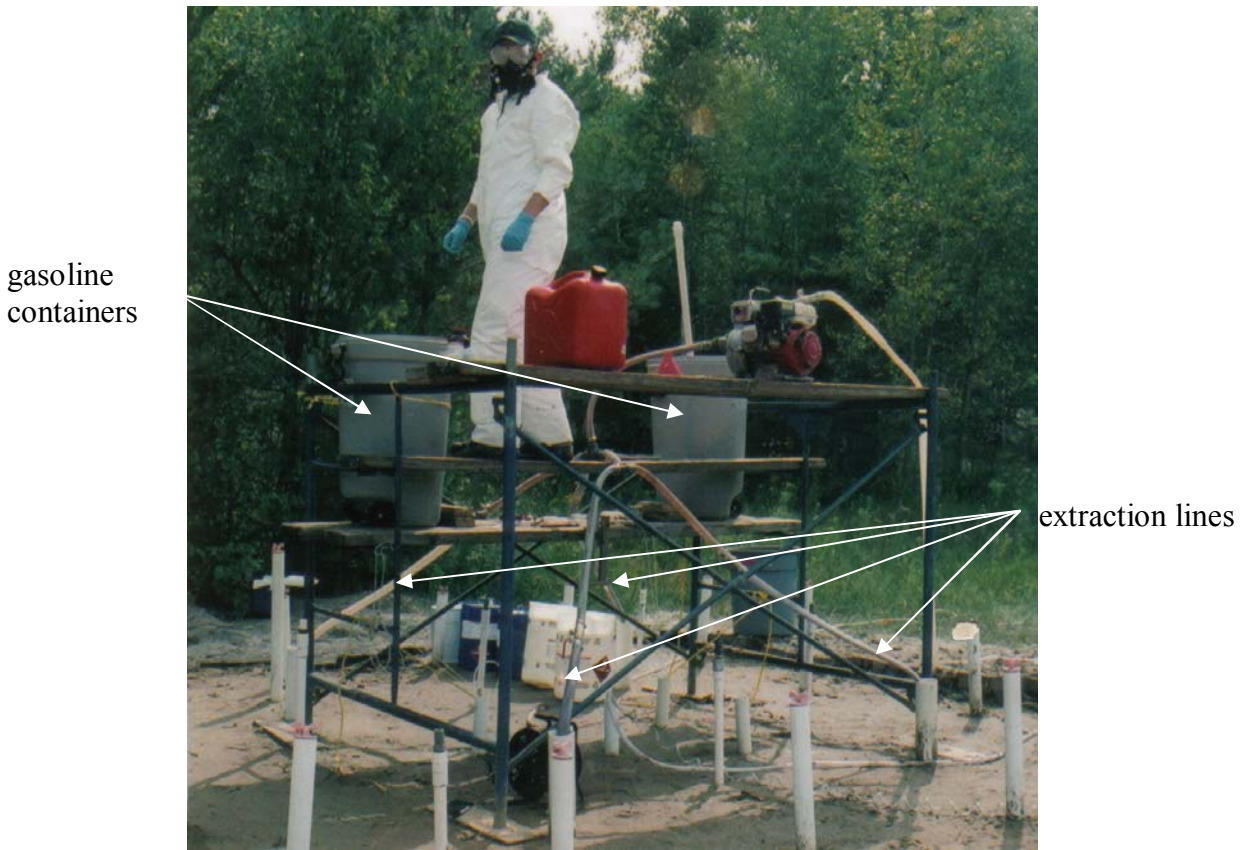
Figure 2.12. Photograph of injection infrastructure, showing both the contaminant injection system and the groundwater extraction system.
