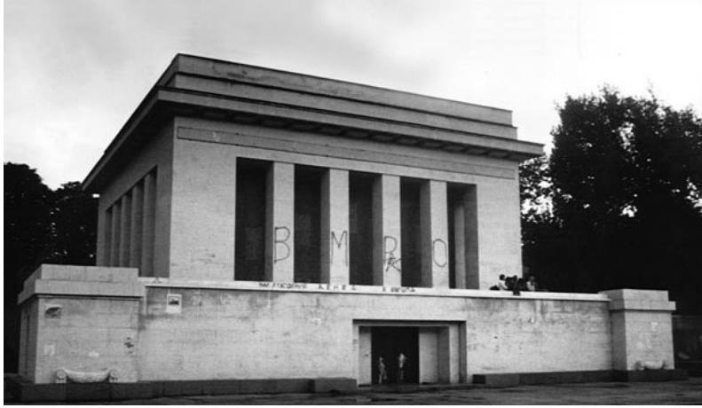
Fig.2.28. In the post-communist years, the building was left empty and neglected. However, while discussion raged about the future of the monumental structure, it changed appearance several times. In 1997, it was covered with dozens of black spots for a promotion of Walt Disney's film "101 Dalmatians." Later that year, it was turned into an Egyptian pyramid for an open-air staging of Giuseppe Verdi's opera "Aida." After the production's success, the National Opera began staging open-air productions in the square in front of the mausoleum.
