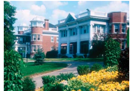
4.38: HHC Existing Western Elevation
