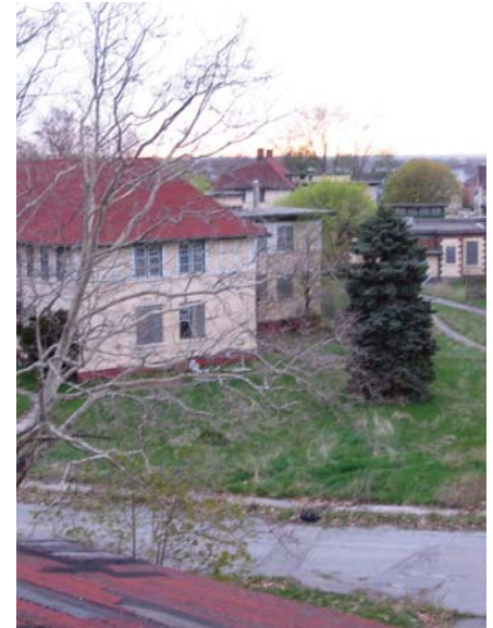
4.14: The Former WMHC, Before Redevelopment.
