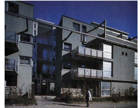
4.84: UHousing Rear Facades
