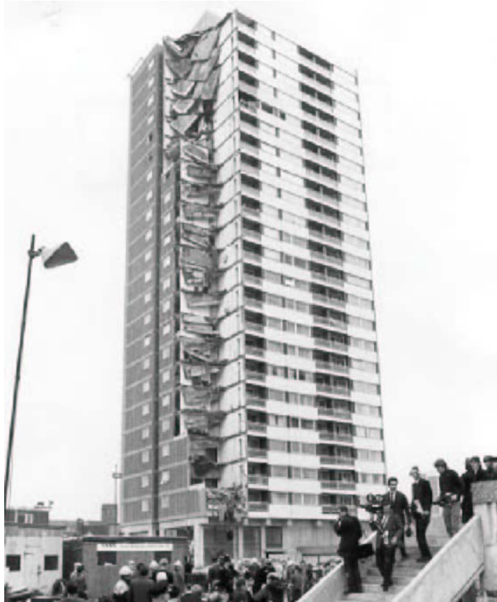
Figure 1.3 Progressive collapse of Ronan Point Flats, UK (Griffiths et al., 1968)
