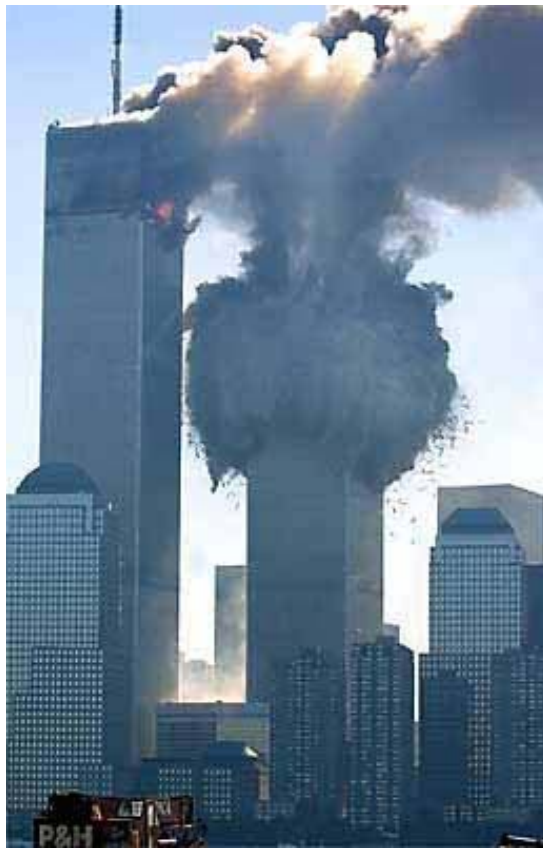
Figure 1.6 Progressive collapse of World Trade Centre tower, New York (FEMA , 2002)
