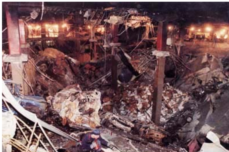
Figure 1.4 Local damage of World Trade Centre building, New York (Bureau of ATF, 1993)
