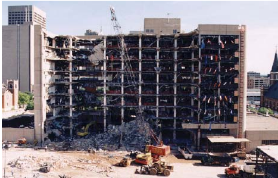
Figure 1.5 Progressive collapse of Murrah Office Building, Oklahoma (Hinman, 1997)
