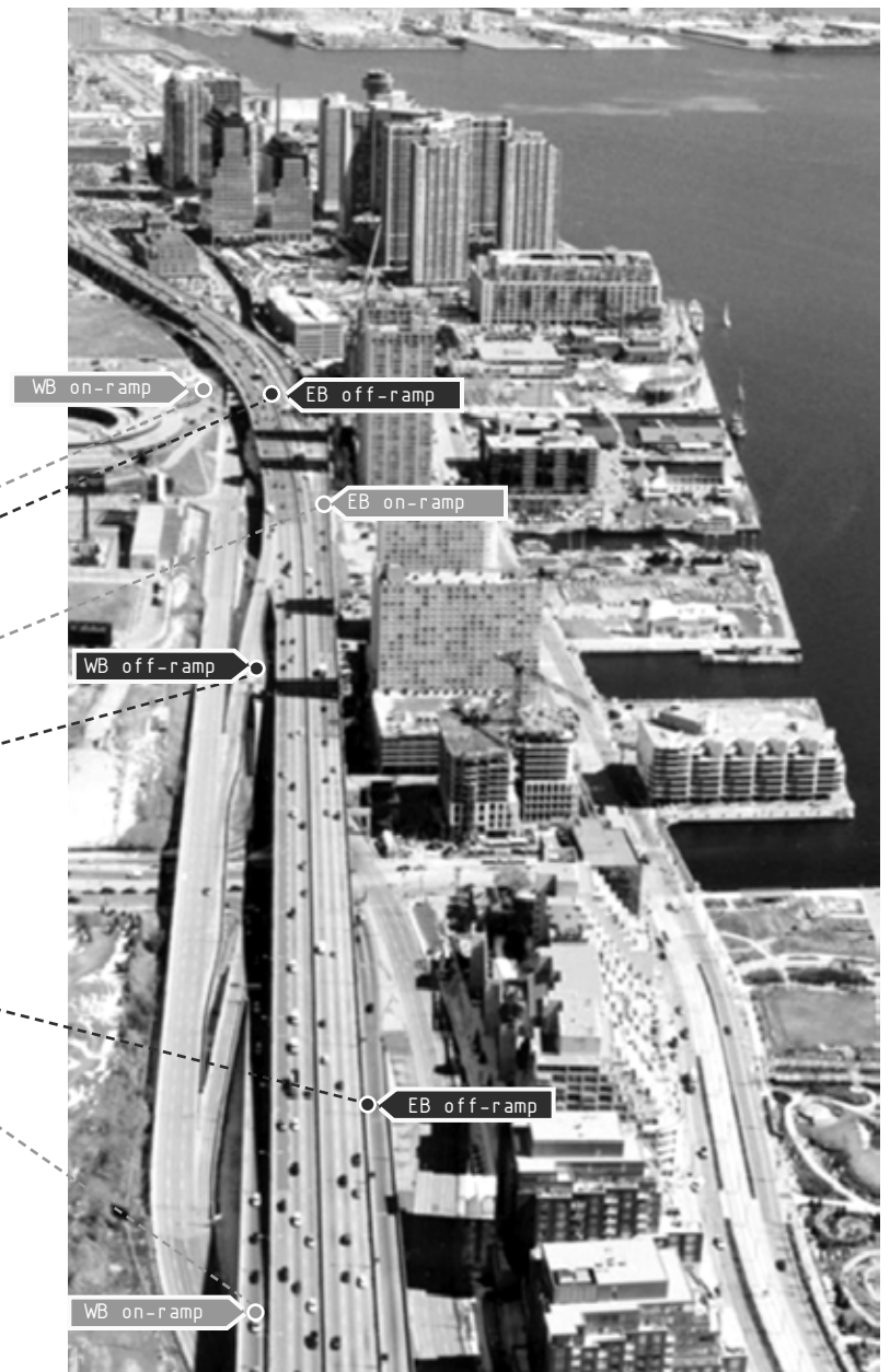
Figure 17 left - Gardiner Expressway on and off ramps
