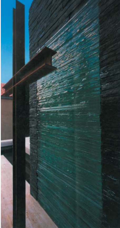
fig 3.30 An example of the use of stacked glass in the Mausoleum in Murcia.
