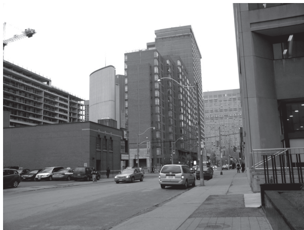
existing site condition (from top) Dundas Street, looking South-West; Dundas Street, looking North-East; Chestnut Street, looking North
