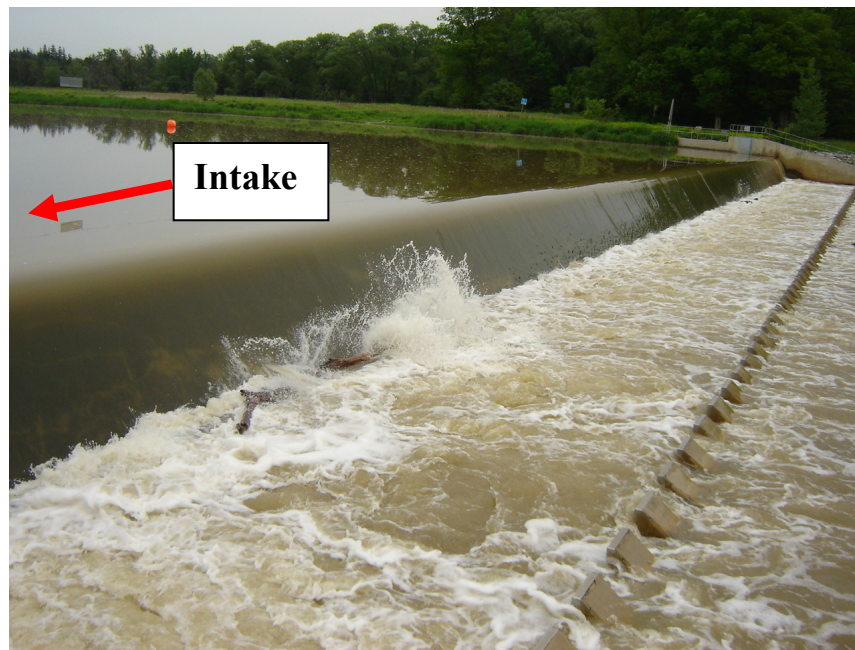
Figure 3-1: Dam on the Grand River at the Mannheim intake
