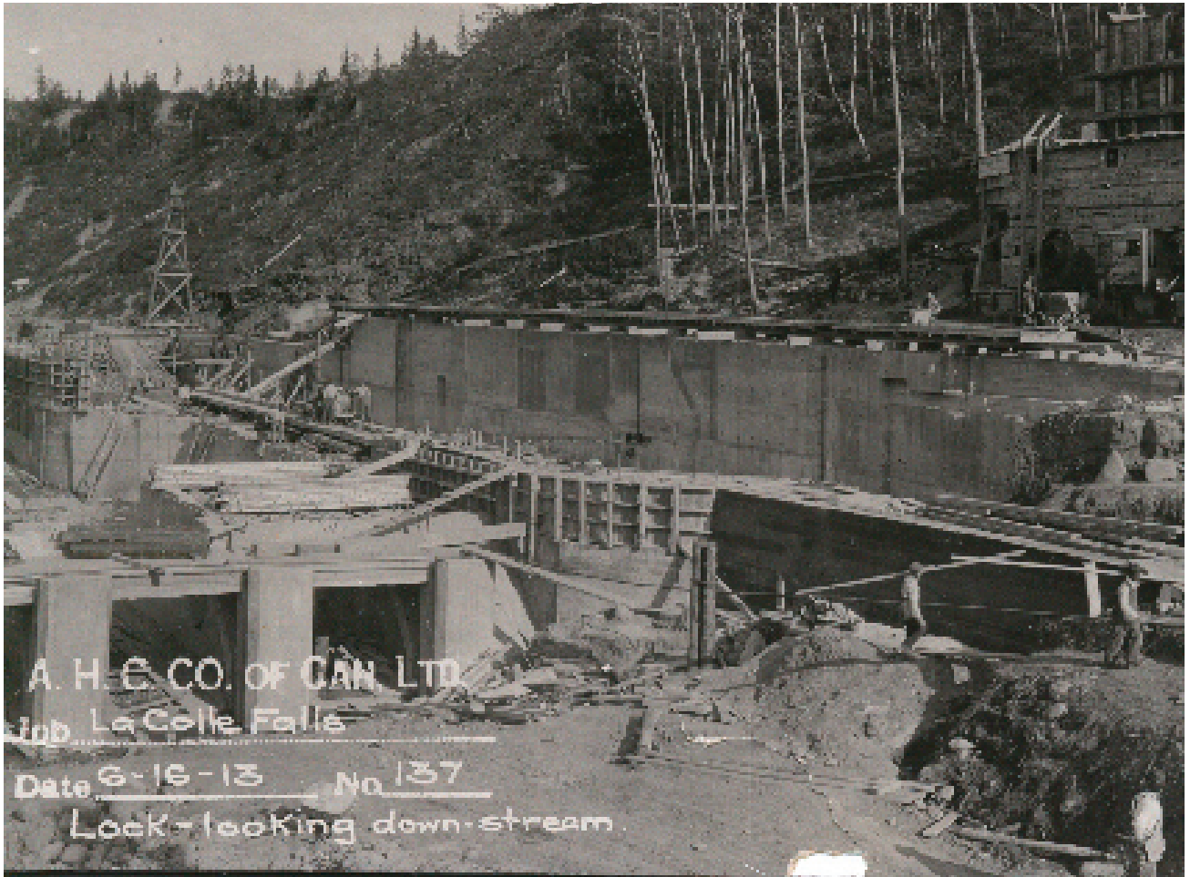
107 Construction Photograph #137 - Lock Looking Down-Stream, the Shipping Lock South Wall is Visible on the Right - Note the Extend of Foliage Cleared on the Ravine Bank
