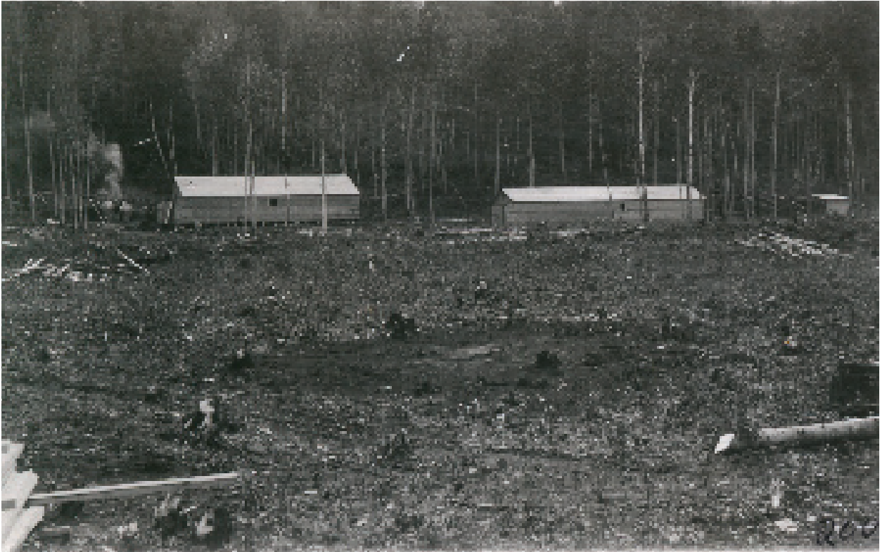
150(Above) Construction Photograph - View of Worker's Camp
