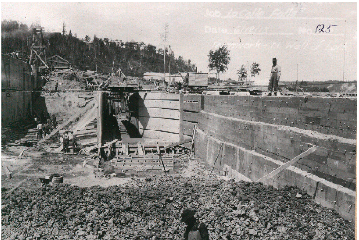
98(Above) Construction Photograph #124 - Cofferdam Connection to the Concrete Ribs of the Weir
