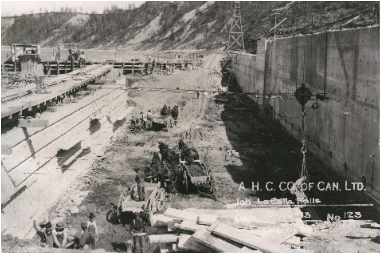
96(Above) Construction Photograph #123A - Using the Cable Pulley System to Move Formwork for the Weir
