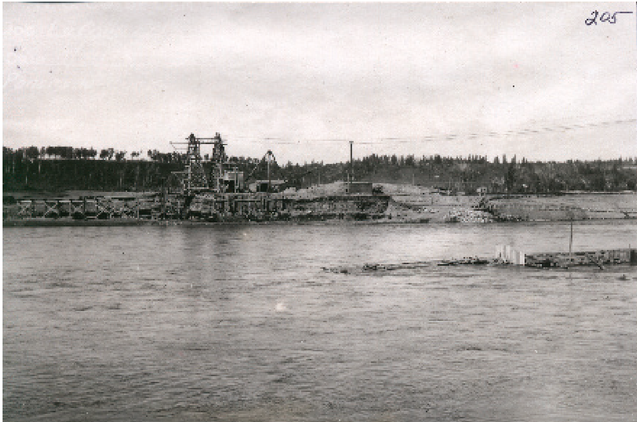
152(Above) Construction Photograph #205
