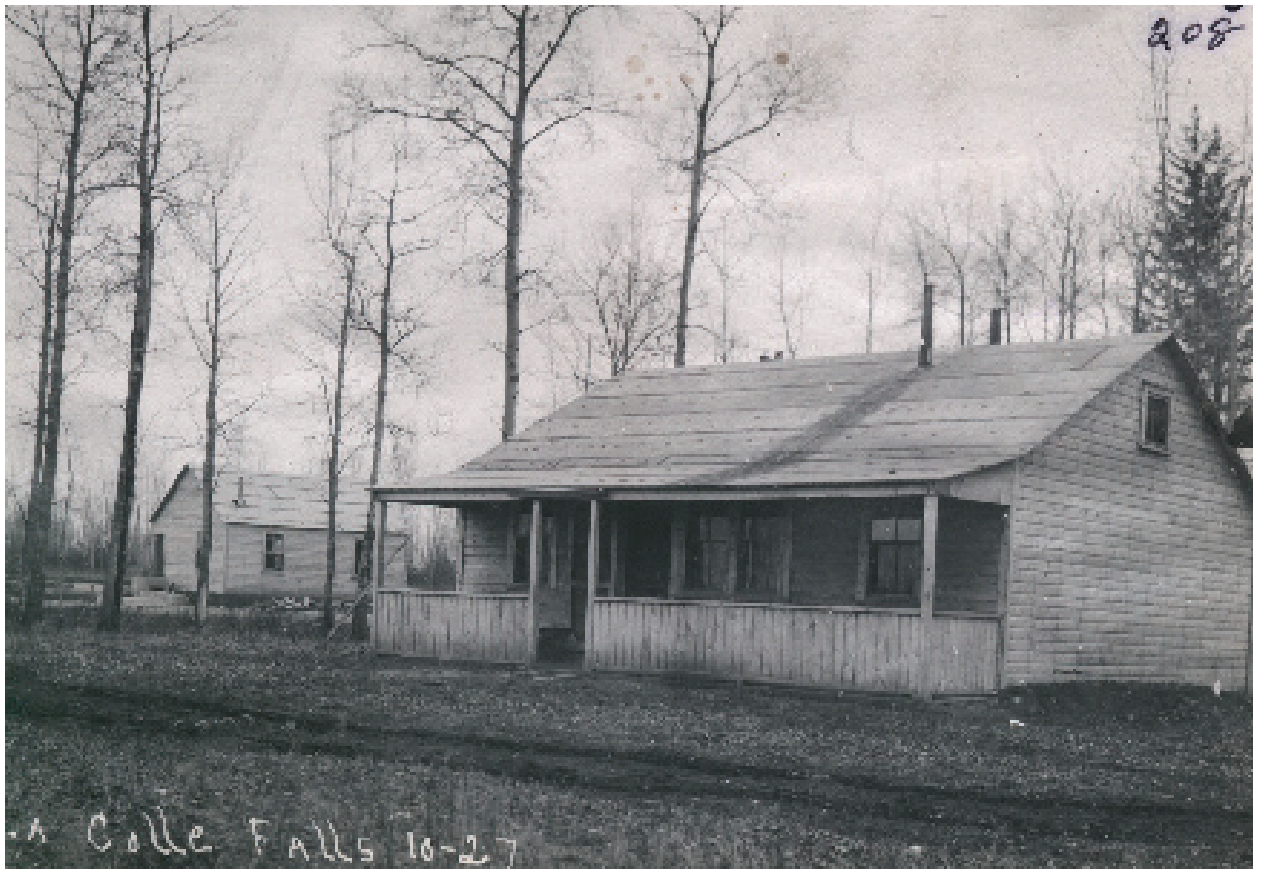
154(Above) Construction Photograph #208 - View of Worker's Camp Showing Wooden Buildings
