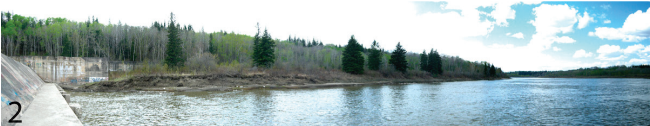
2 12 View Up-River from Dam
