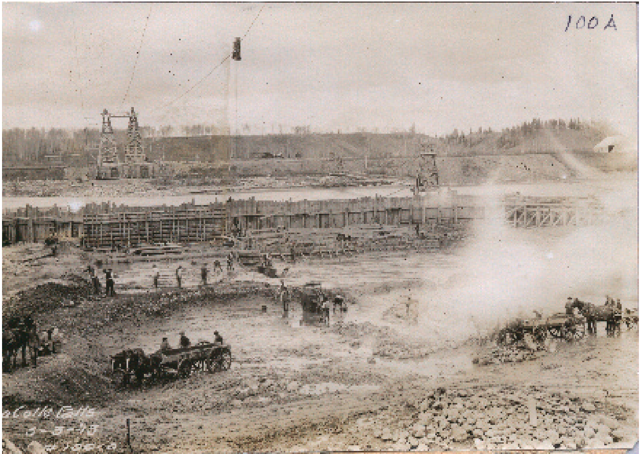
79(Above) Construction Photograph #100 - The Area Inside the Wooden Cofferdam in the River is Drained, and Debris is Removed
