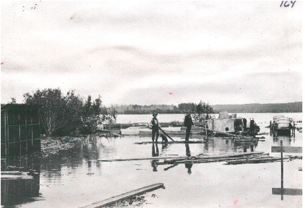
129(Above) Construction Photograph #169 - Filling the Tail Race (Power Canal) with River Water
