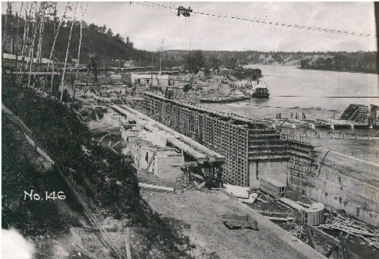
114 Construction Photograph - Panorama - #146 and #145 - Looking Upstream - View Showing the Construction Site at Peak Activity, the Shipping Lock is Visible on the Left Side and the Partially Completed Weir Reaches Across the River, Note - the Weir was Constructed with a Curved Design to Allow Debris to be Easily Carried Over the Dam During Times of Flood and High water
