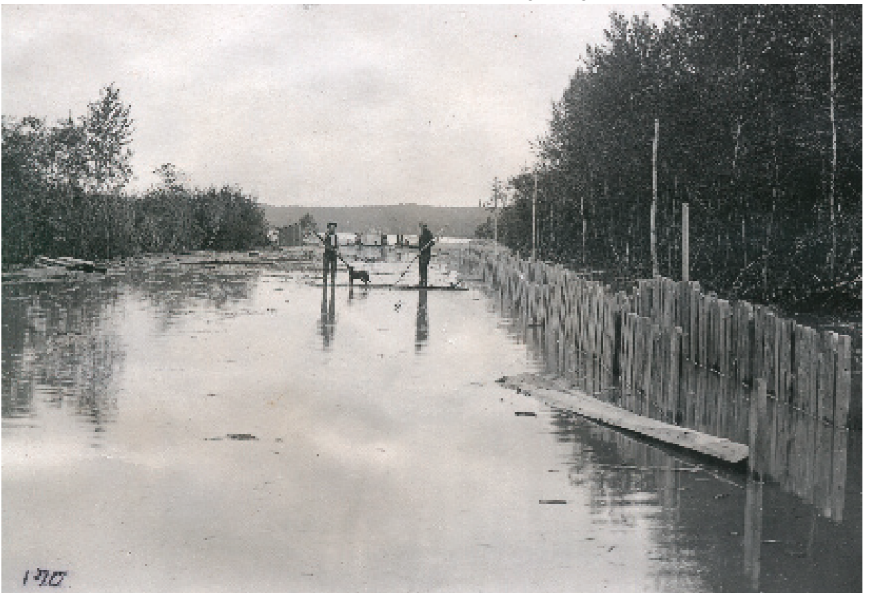
129(Above) Construction Photograph #169 - Filling the Tail Race (Power Canal) with River Water
