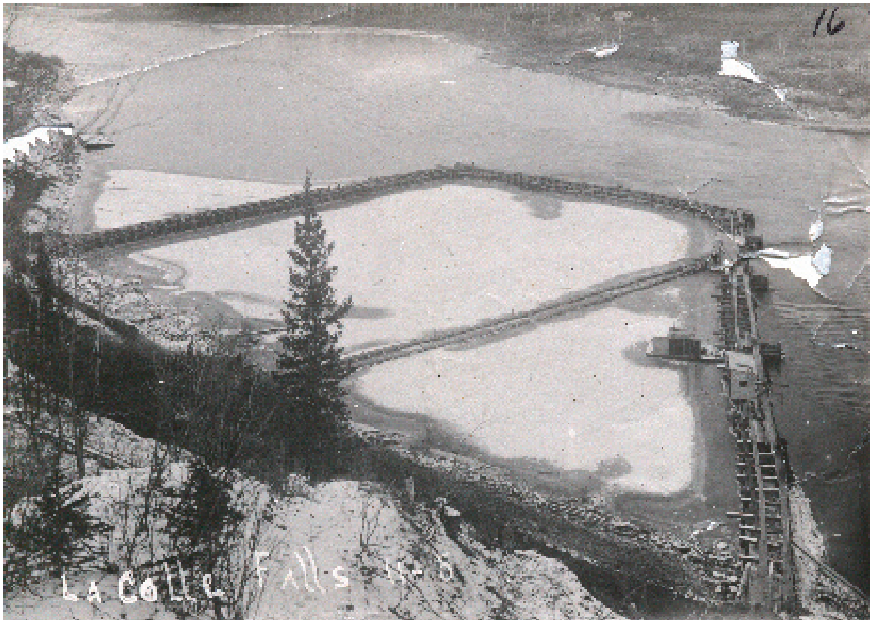
75(Above) Construction Photograph - A Wooden Cofferdam Was Constructed in the River to Hold Back the Water on the Construction Site
