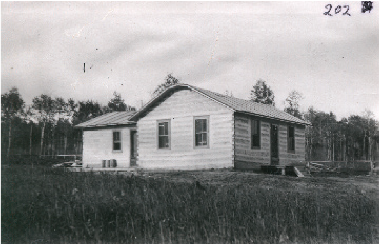
151(Below) Construction Photograph #202 - View of Worker's Camp Showing Log Building
