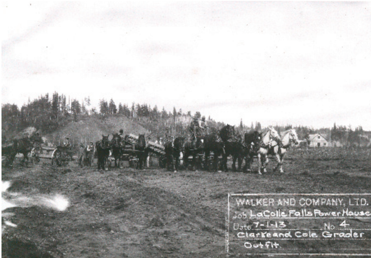
77(Above) Construction Photograph #4 - The Team of Horses Beginning the Excavation for the Powerhouse
