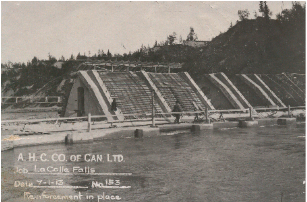
117 Construction Photograph #153 - Reinforcement in Place for the Crest of the Weir
