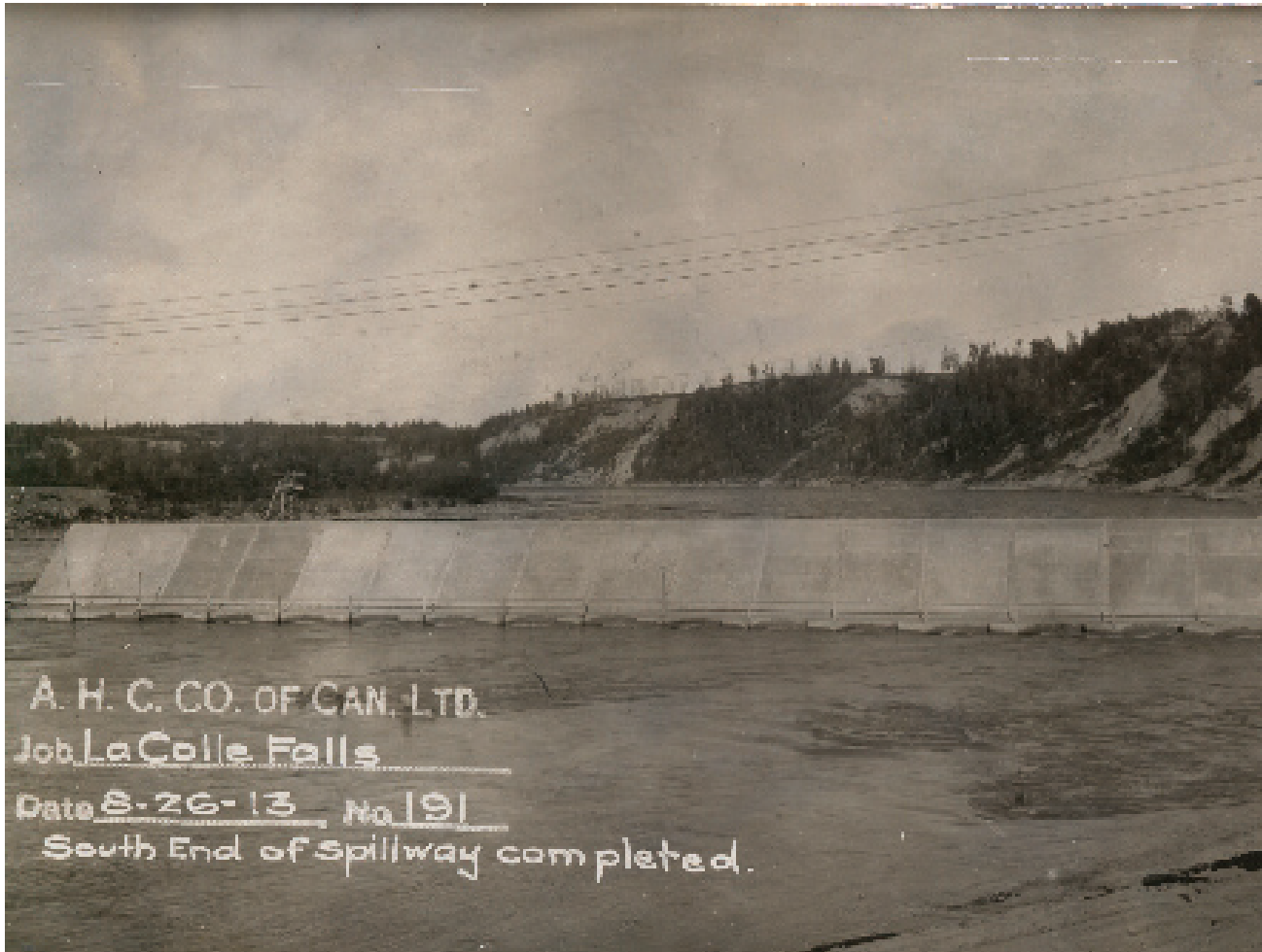
143 Construction Photograph - Panorama - #191, and #192 - View Showing Weir at South End of Spillway Completed and Shipping Lock Nearly Completed (at Right)
