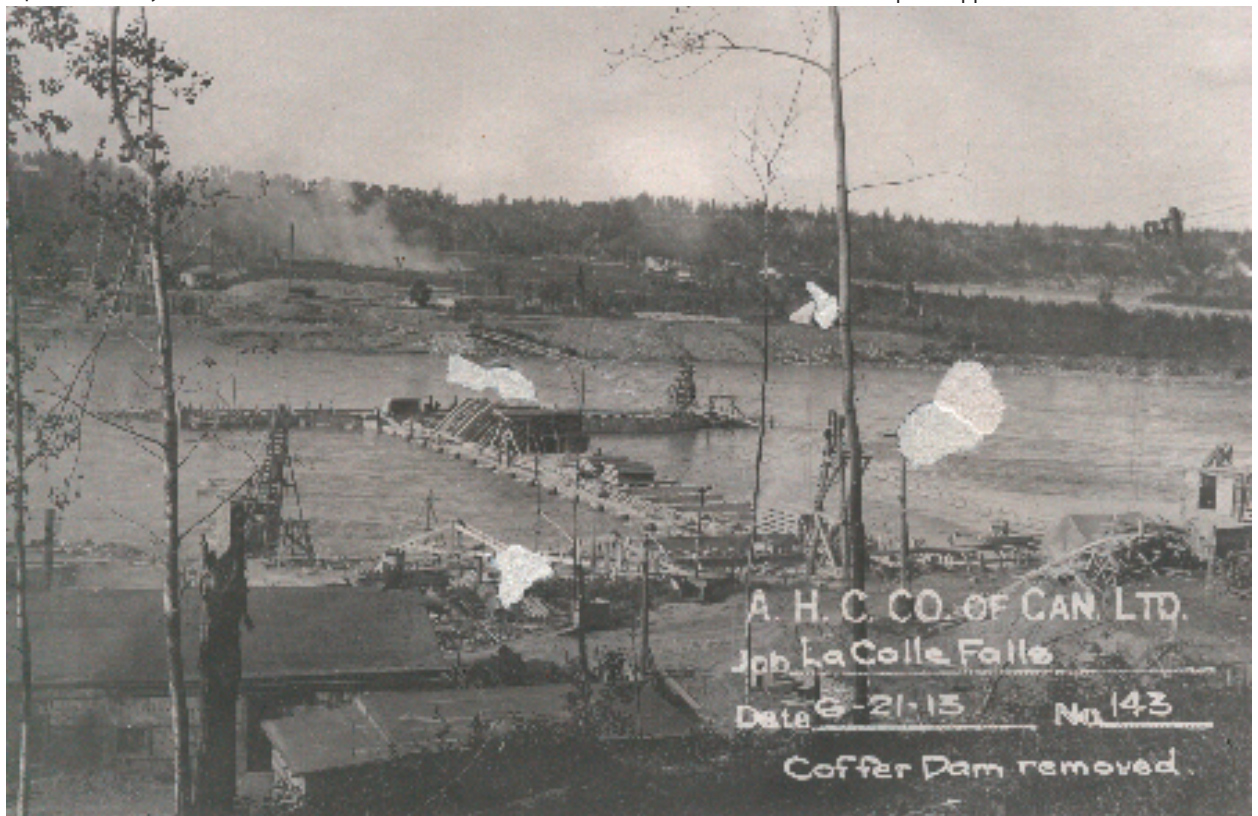
110(Above) Construction Photograph #142 - Blowing Out Coffe-Dam - After Allowing Water to Enter, the Coffe Dam was Exploded with Dynamite
