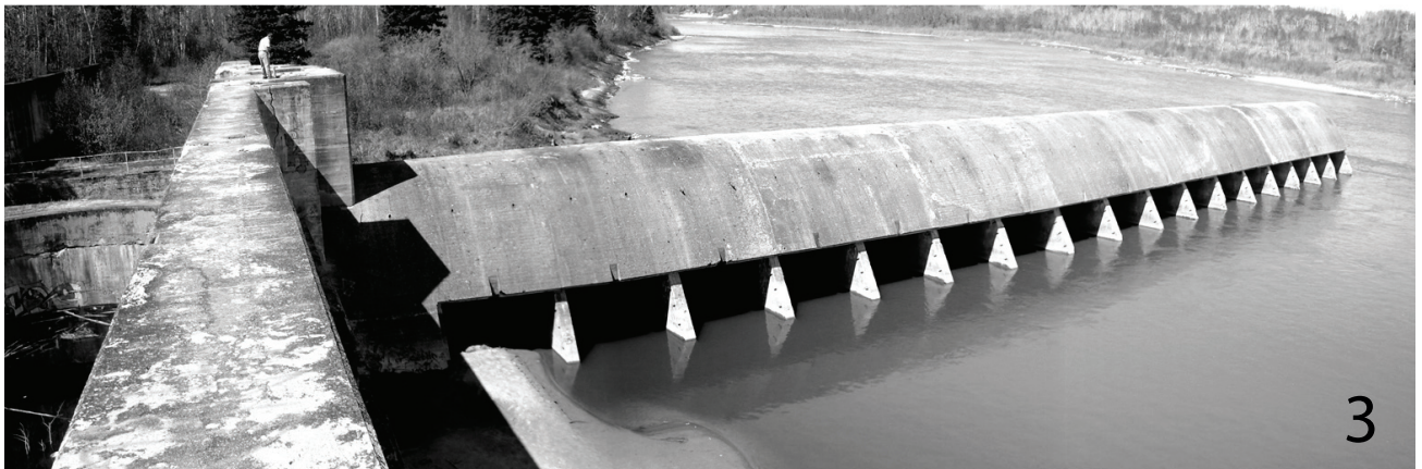
25 View of the Weir in the River Looking Upstream
