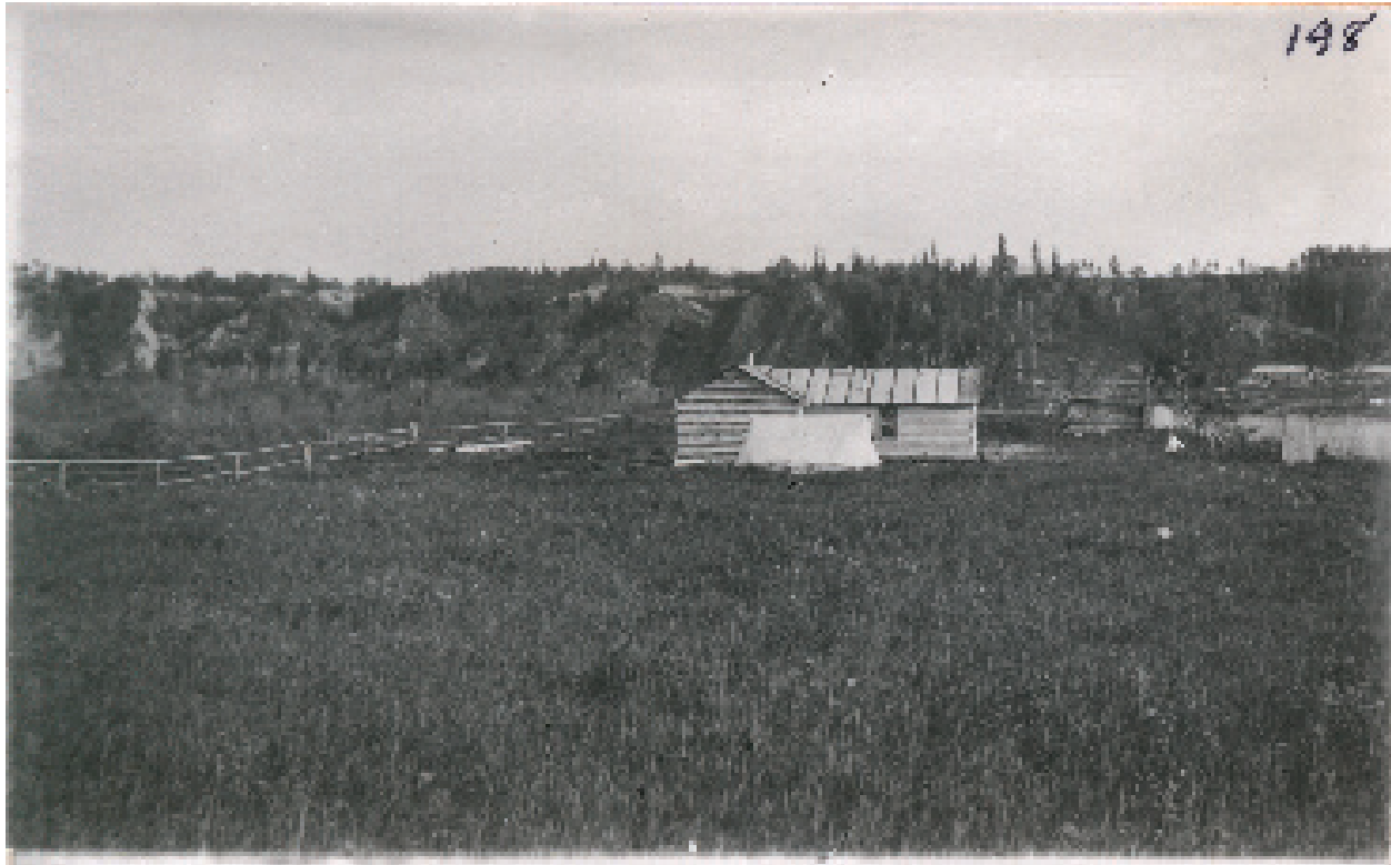
148(Above) Construction Photograph #198 - View of Worker's Camp at Top of South River Bank Showing Log Building
