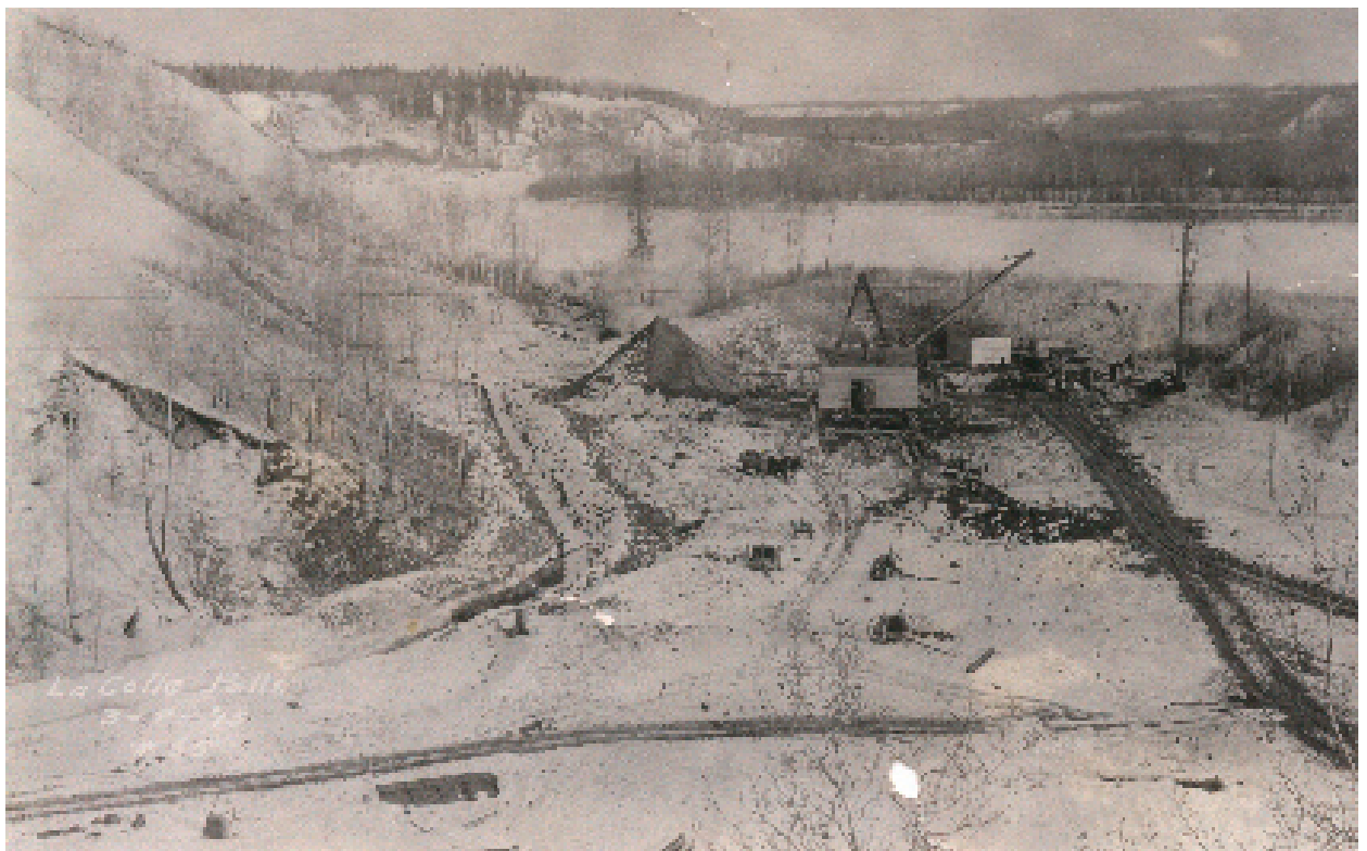
75(Above) Construction Photograph - A Wooden Cofferdam Was Constructed in the River to Hold Back the Water on the Construction Site
