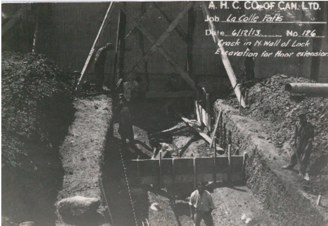
100(Above) Construction Photograph #126 - Crack in North Wall of Shipping Lock Excavation for Floor Extension
