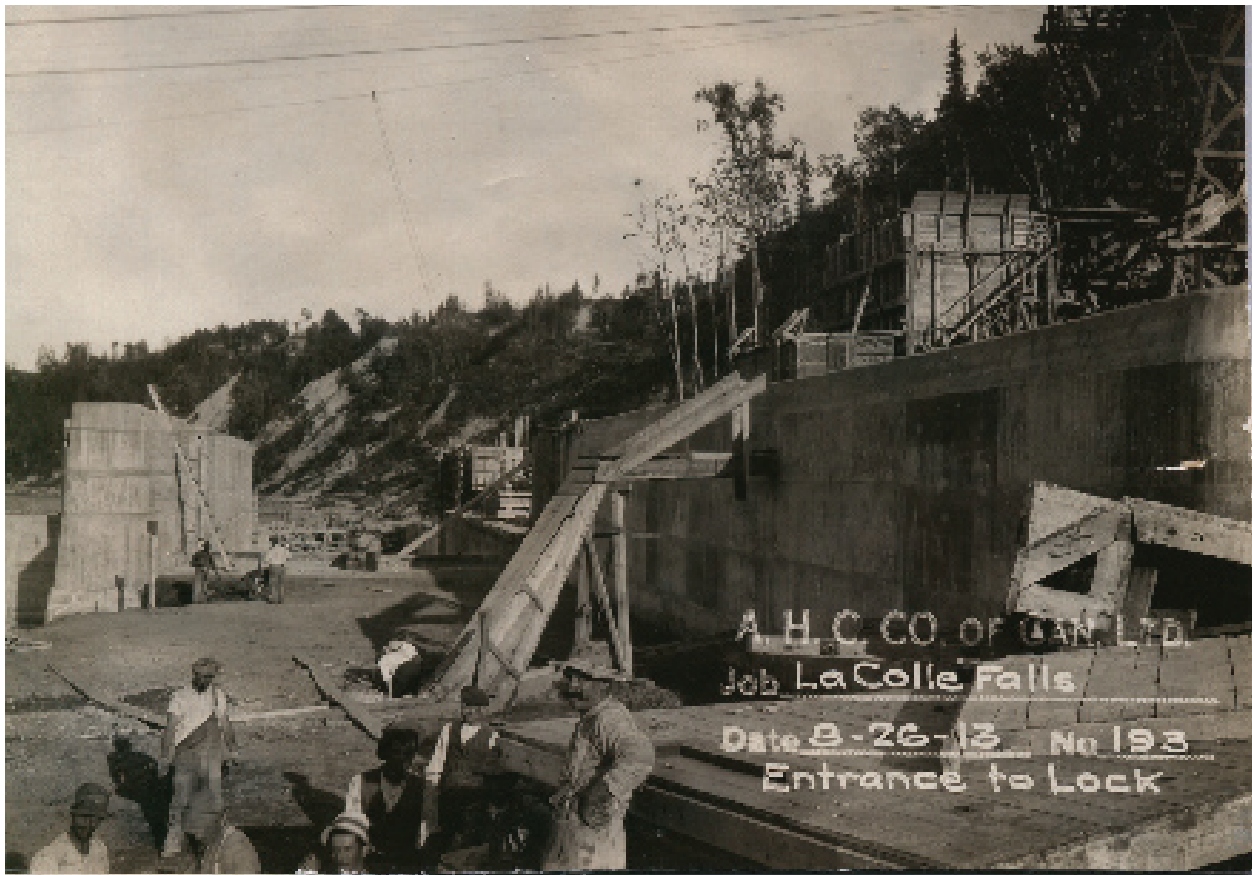
144(Above) Construction Photograph #193 - View of Nearly Completed Entrance to Shipping Lock
