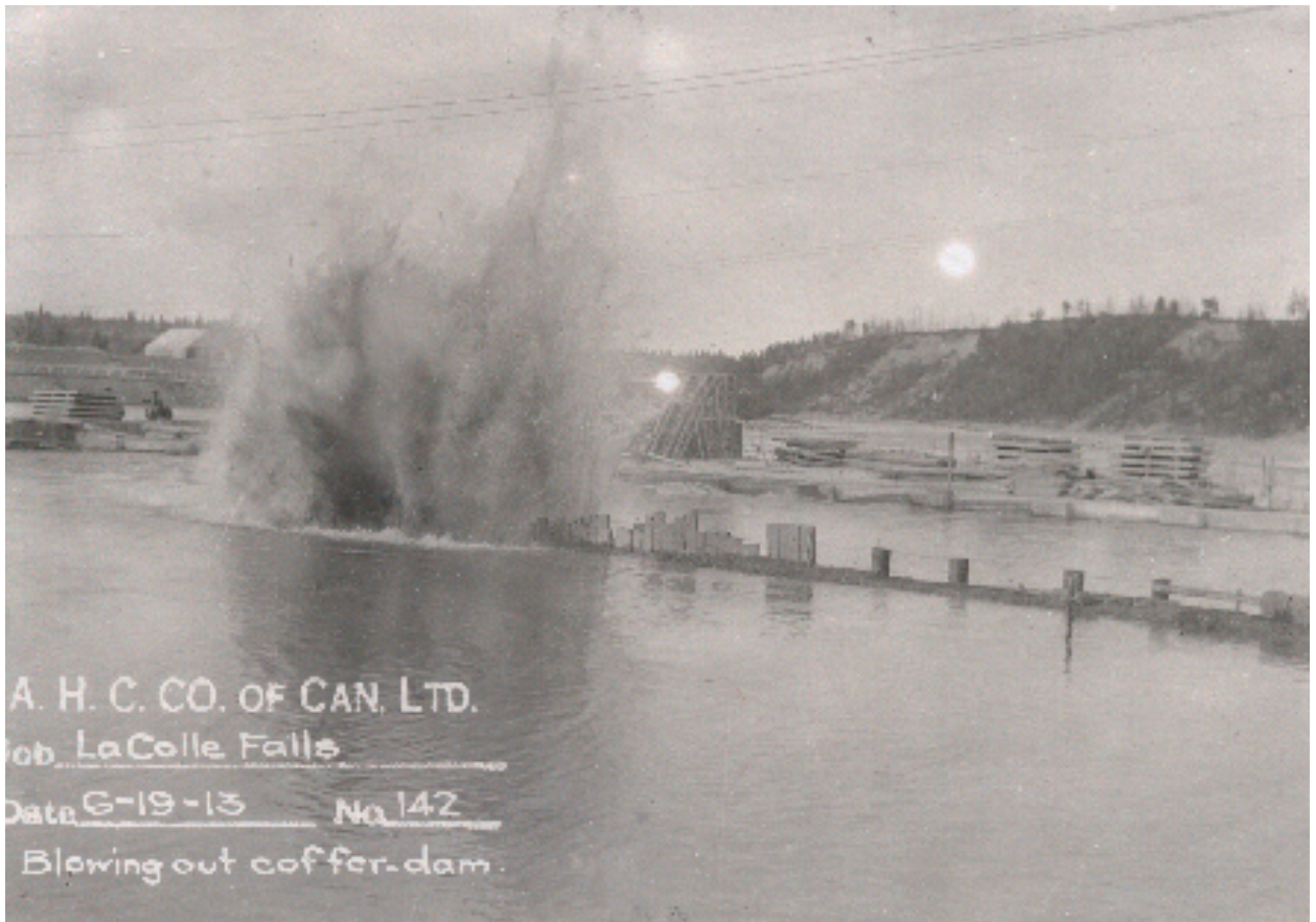
110(Above) Construction Photograph #142 - Blowing Out Coffe-Dam - After Allowing Water to Enter, the Coffe Dam was Exploded with Dynamite
