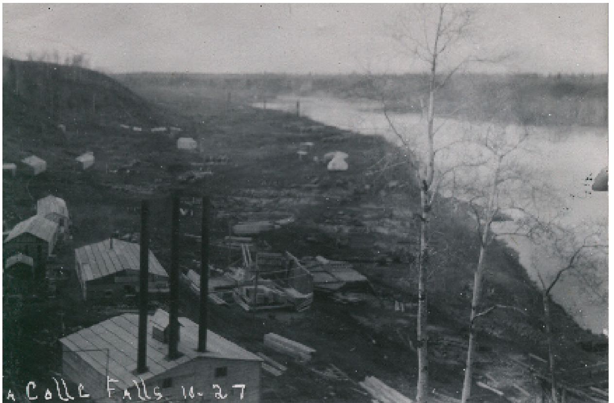
155(Below) Construction Photograph - View of the Supplies and Workshop Buildings on the River Flat, South Bank
