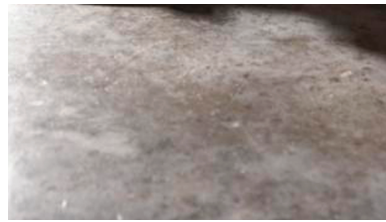
Polished Concrete Floor
