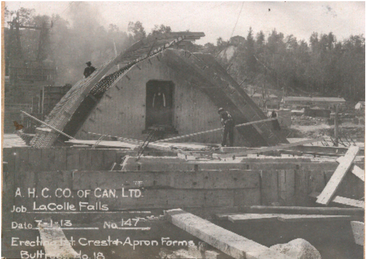
113 Construction Photograph #147 - Erecting 1st Crest & Apron Forms Buttress No. 18 of the Weir, Note the Curved Construction of the Weir to Allow Debris to be Easily Carried Over the Dam During Times of High Water
