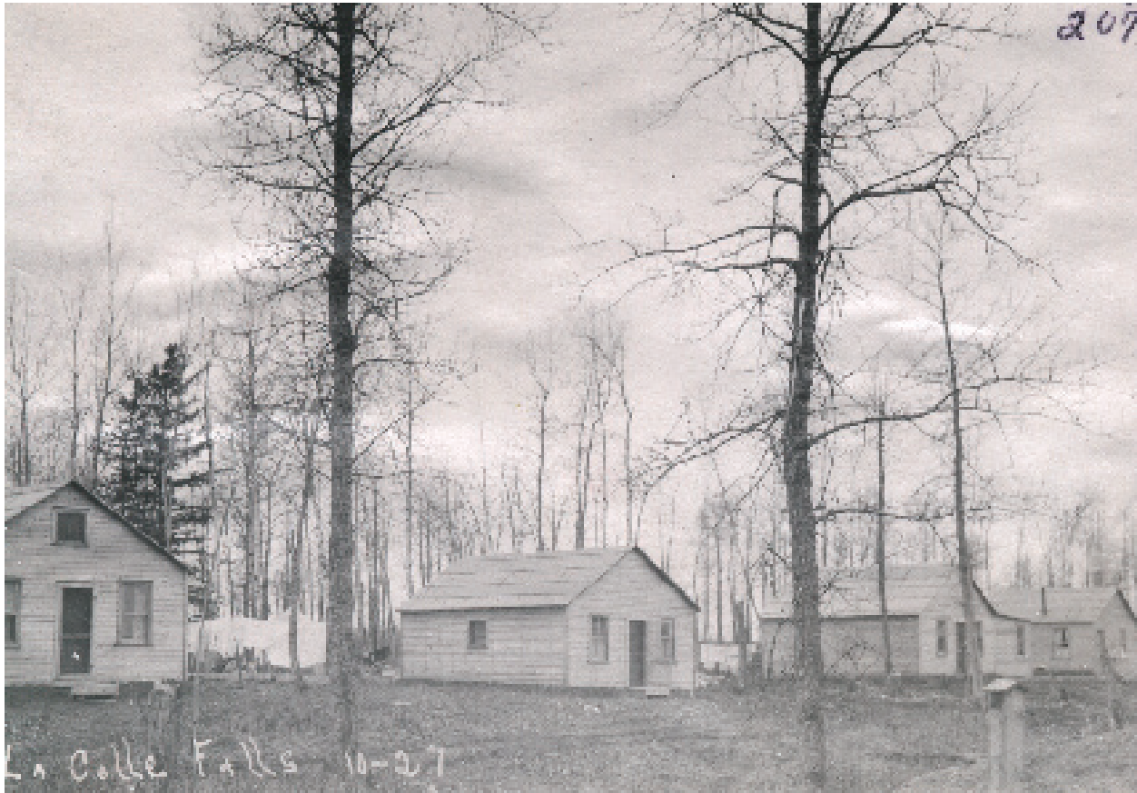
153(Below) Construction Photograph #207 - View of Worker's Camp Showing Wooden Buildings
