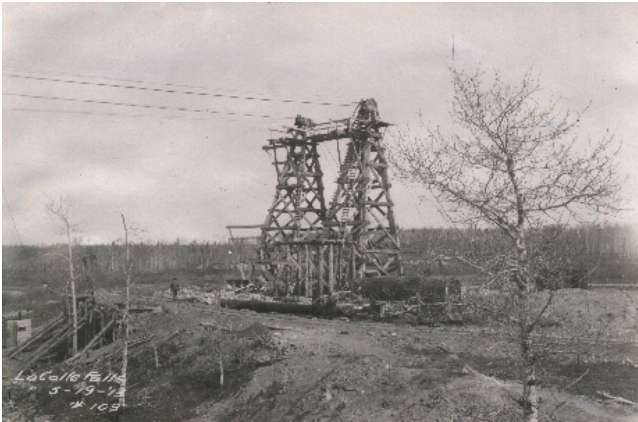
85(Above) Construction Photograph #108 - Using the Cable Pulley System to Move a Steel Boiler Across the River
