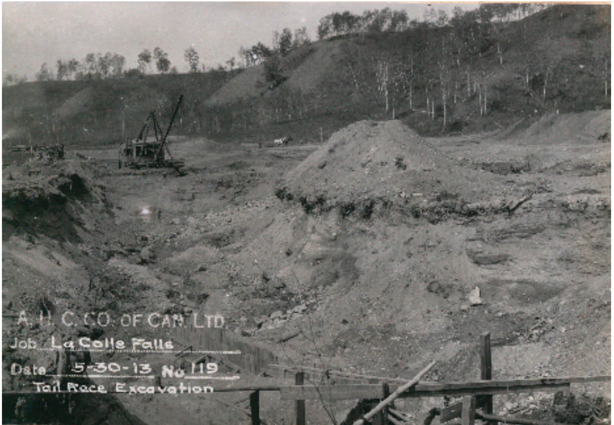
93(Above) Construction Photograph #119 - Tail Race (Power Canal) Excavation with Grading Machine
