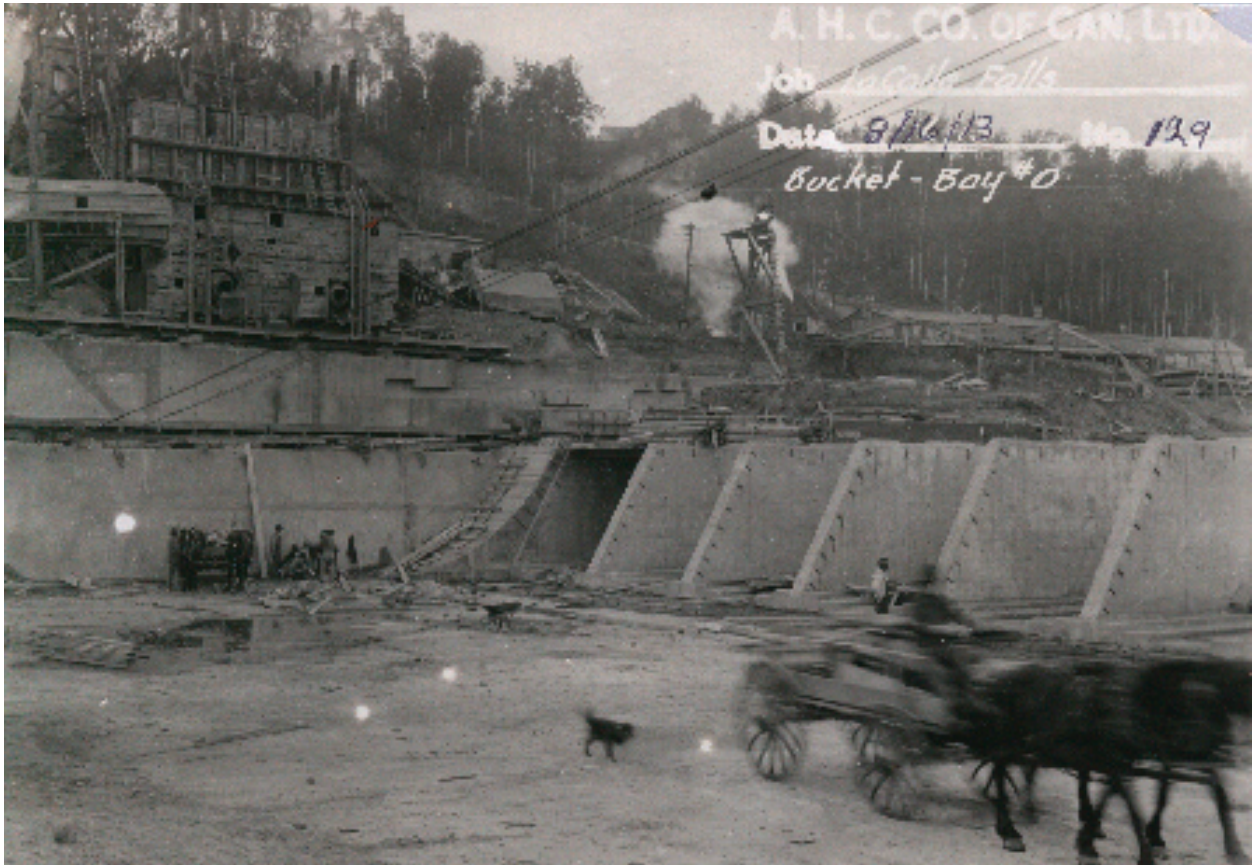
102(Above) Construction Photograph #129 - Ribs of Weir with Spouts of Concrete Chute Visible in the Background Above Shipping Lock
