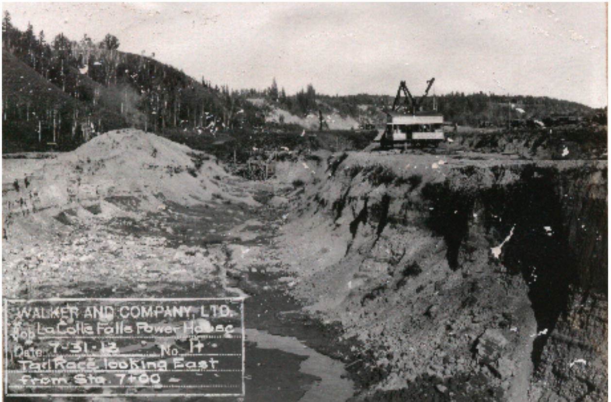
93(Above) Construction Photograph #119 - Tail Race (Power Canal) Excavation with Grading Machine
