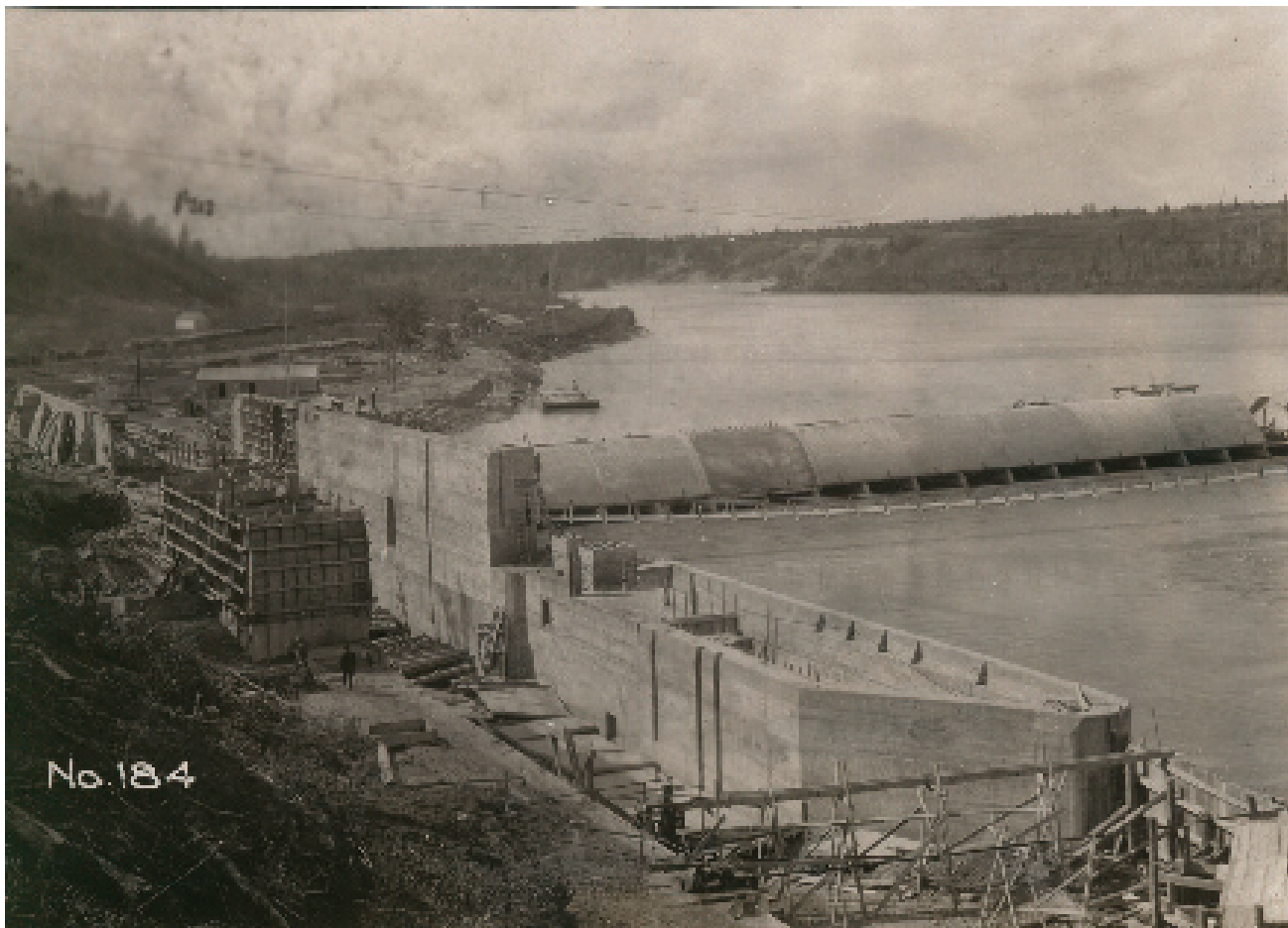
138 Construction Photograph - Panorama - #184, and #185 - View Looking Upstream Showing the Nearly Complete Shipping Lock and Weir
