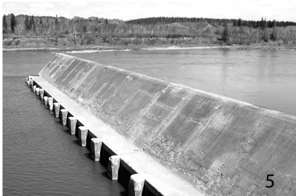
27 View of the Weir Ledge
