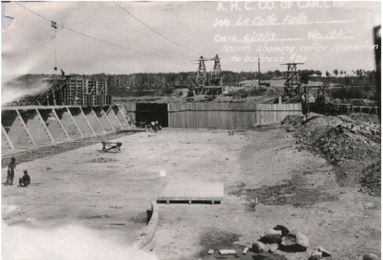
98(Above) Construction Photograph #124 - Cofferdam Connection to the Concrete Ribs of the Weir
