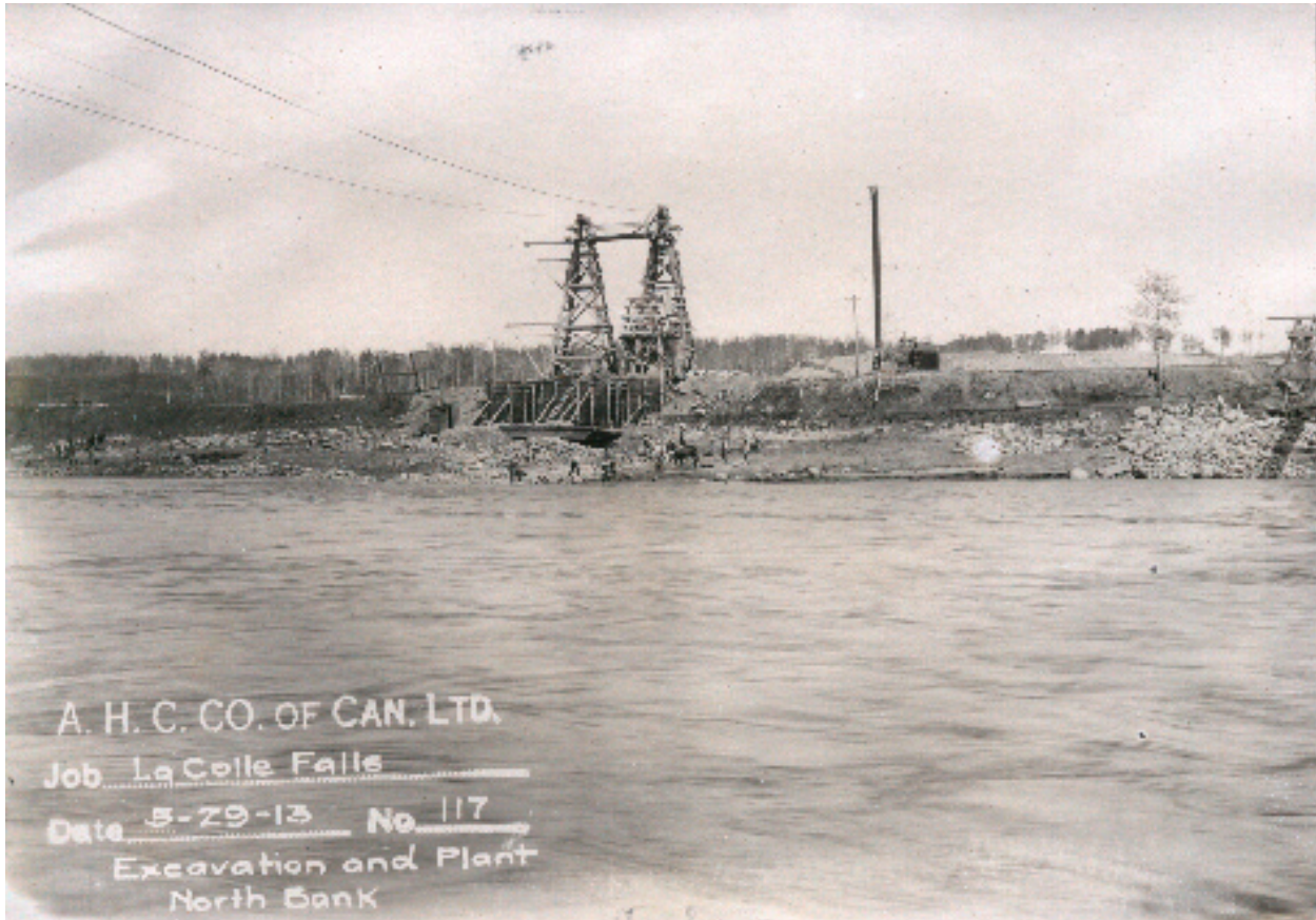
91(Above) Construction Photograph #117 - Excavation and Plant North Bank - View Showing the Towers for the Cable Pulley System
