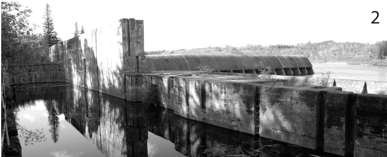
23 View of the Shipping Lock Pool and Weir Beyond Looking Upstream
