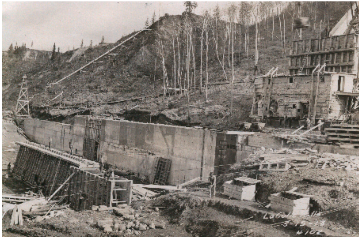
79(Above) Construction Photograph #100 - The Area Inside the Wooden Cofferdam in the River is Drained, and Debris is Removed
