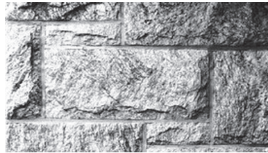
Cut Native Granite Masonry
