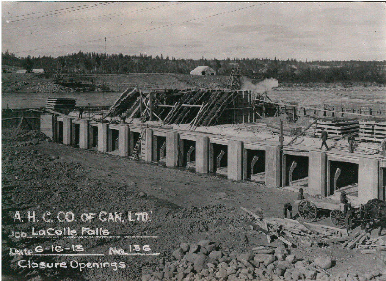
106 Construction Photograph #136 - View Showing Weir Closure Openings, the River Water Would Have Passed Through the Openings, In Times of Low Water, Doors Would Have Been Closed to Raise the Water Level
