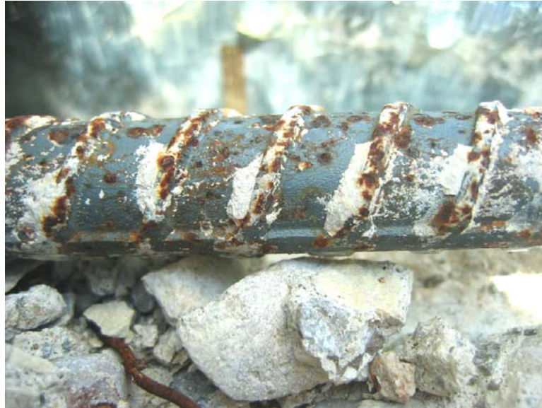
Figure 4.7 Condensed crushed concrete in front of the steel bar lugs for wrapped beams
