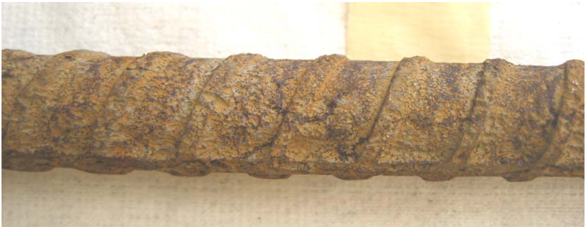
Figure 3.1: Uniform corrosion for steel bars corroded for 50 days
