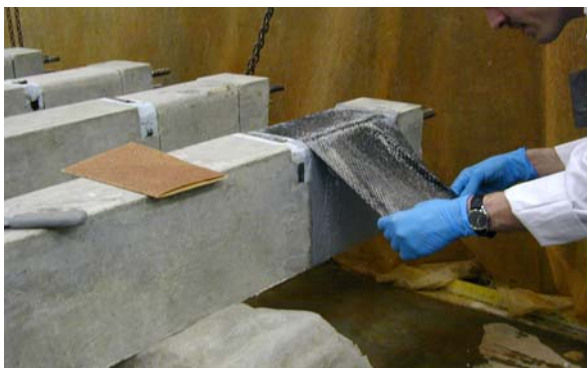
c) CFRP sheet application
