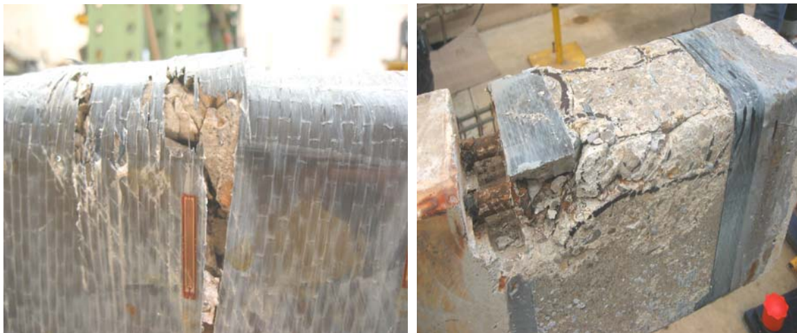
a) Rupture of CFRP sheets
