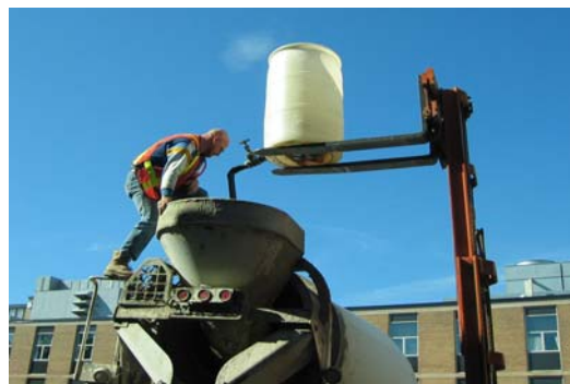
Figure 2.8: Salted and unsalted water added to the ready-mix concrete
