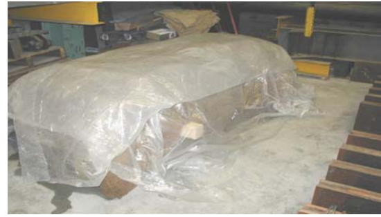
b) Beams Curing
