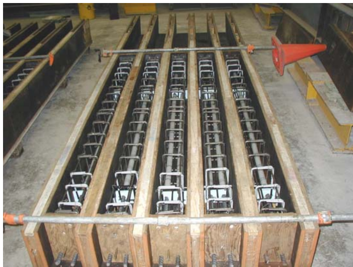
Figure 2.7: General view of the cages in the formwork before casting
