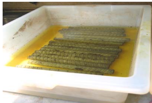
b) Chemical cleaning process
