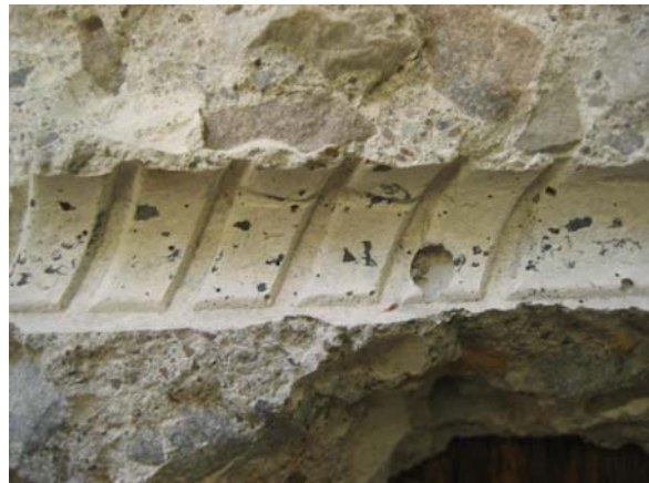
b) Concrete below steel bar (bottom cover)
