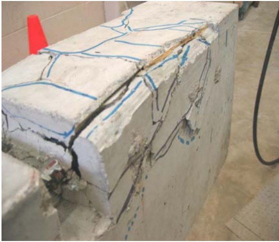
a) Concrete splitting for uncorroded beams
