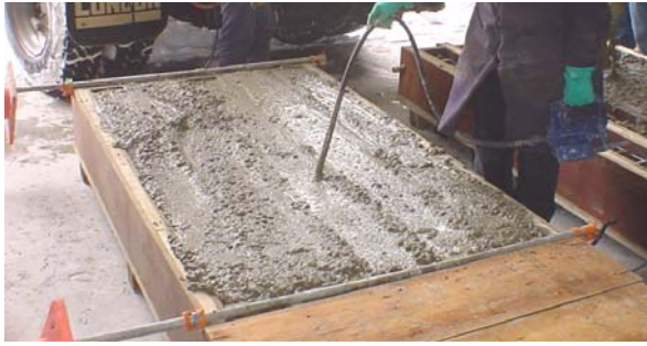
a) Concrete vibration
