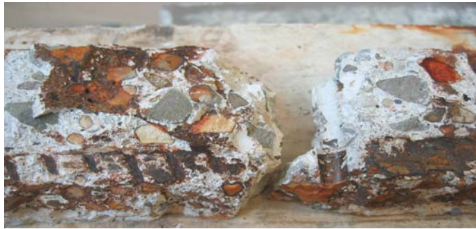
Figure 3.11 Failure plane for unwrapped corroded beams
