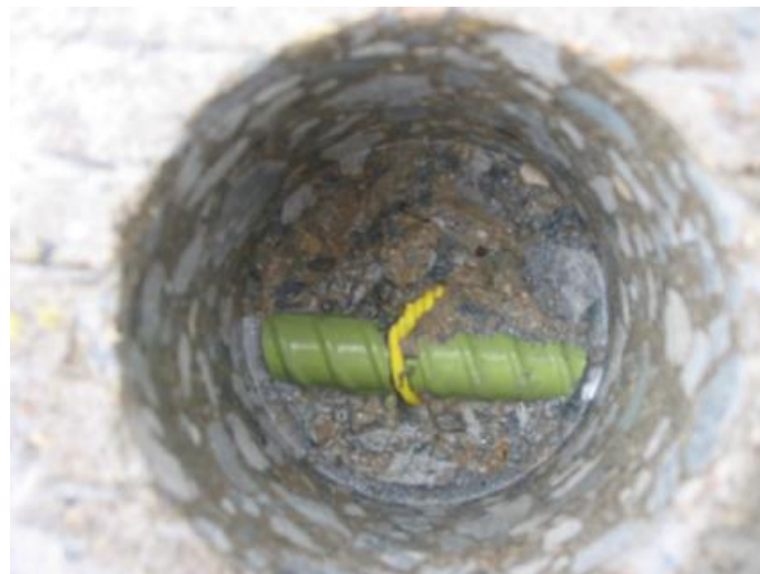
Figure 3. 24. Epoxy coated steel bar used in the deck of the bridge at the University of Waterloo.
