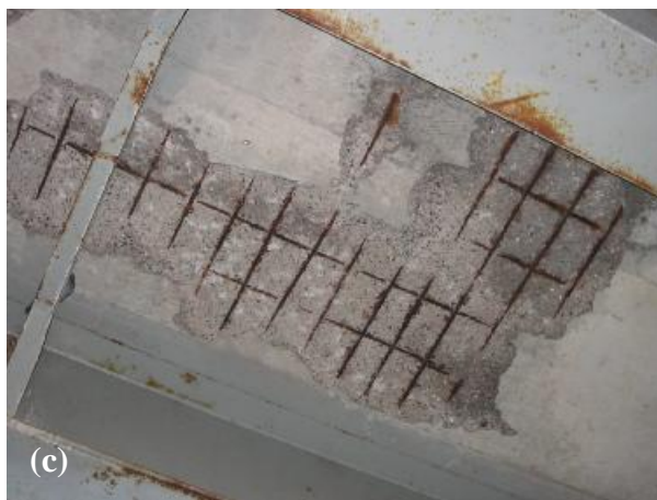
Figure 3. 30. Photograph from Island Park Bridge, Ottawa, Ontario (a) corrosion of the steel bars of one of the approaches of the bridge, (b) repaired areas of the bridge, (c) corrosion underneath the bridge deck and (d) severely corroded spot on one of the approaches.
