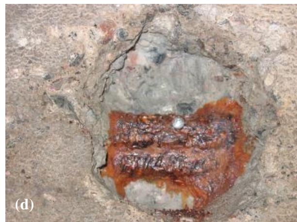
Figure 3. 30. Photograph from Island Park Bridge, Ottawa, Ontario (a) corrosion of the steel bars of one of the approaches of the bridge, (b) repaired areas of the bridge, (c) corrosion underneath the bridge deck and (d) severely corroded spot on one of the approaches.
