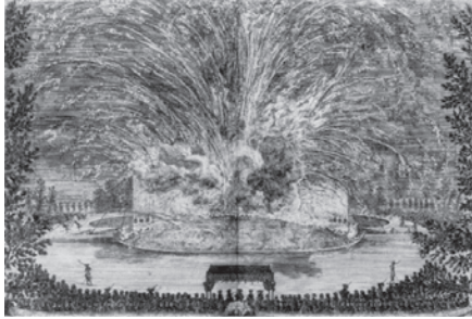
2-7 Fireworks, and the destruction of Alcine's Palace.
