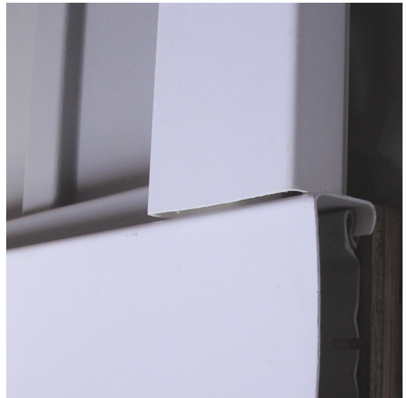
Top Left: 2.261 Drywall installed. Top Right: 2.262 White vinyl fascia installed below the brown shingles and above the white soffit and the grey siding. Above Left: 2.263 Installing the vinyl soffit beneath the carport. Above Right: 2.264 The vertical joint cover overhanging the shallower profile of five-inch-wide window surround trim. Left: 2.265 Drywall taped.
