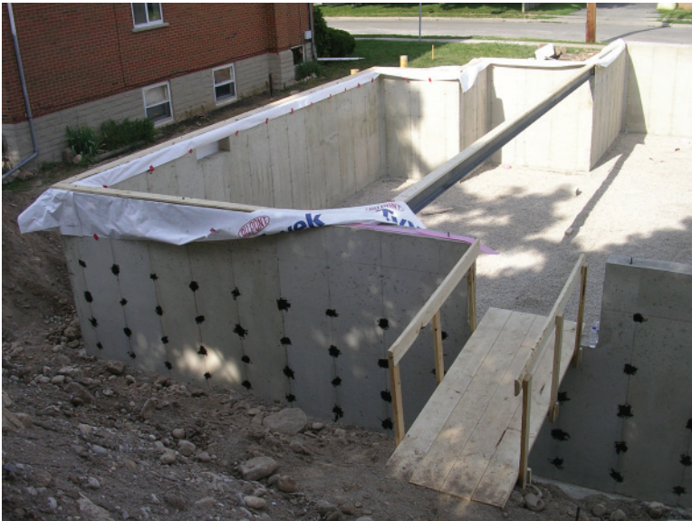
Above Left: 2.169 Installing sill gasket along the top of the foundation wall.
