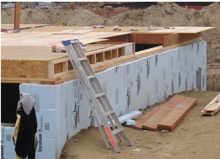
Above Left: 1.15 An erected kitchen wall panel. Above: 1.16 An erected party wall panel complete with gypsum board for fire separation. Left: 1.17 Additional framing is needed to make up the difference between the width of the foundation and the width of the floor panels.
