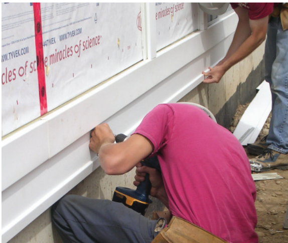
Above Left: 2.270 Installing the starter pieces for the horizontal band of siding.
