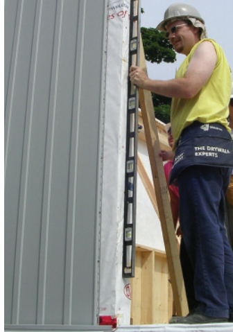
Facing Page Top: 2.191-2.193 Erecting the first wall of exterior wall panels.
