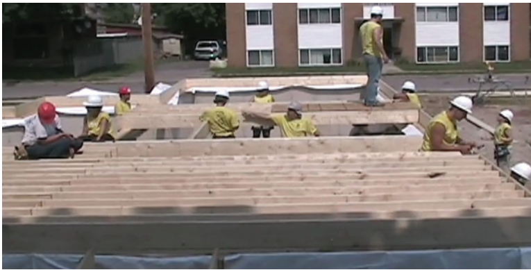
Above Left: 2.172 Installing rim boards.
