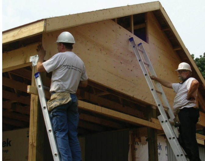
Above: 2.240 Driving a nail at the corner of a sheet of OSB roof sheathing to secure it in place.
