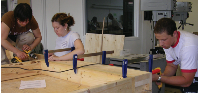
Left: 2.110 Using clamps to help install a lintel.
