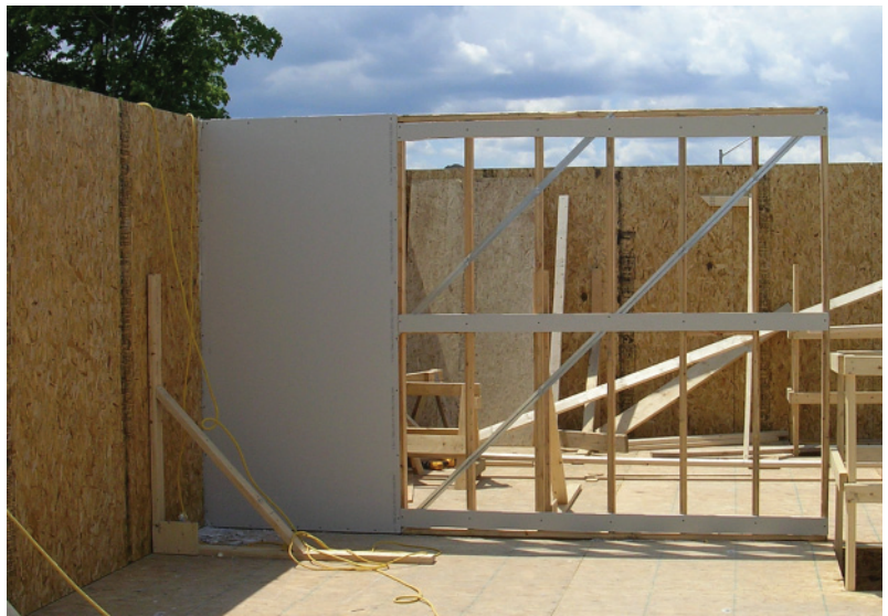
Above Left: 1.15 An erected kitchen wall panel. Above: 1.16 An erected party wall panel complete with gypsum board for fire separation. Left: 1.17 Additional framing is needed to make up the difference between the width of the foundation and the width of the floor panels.
