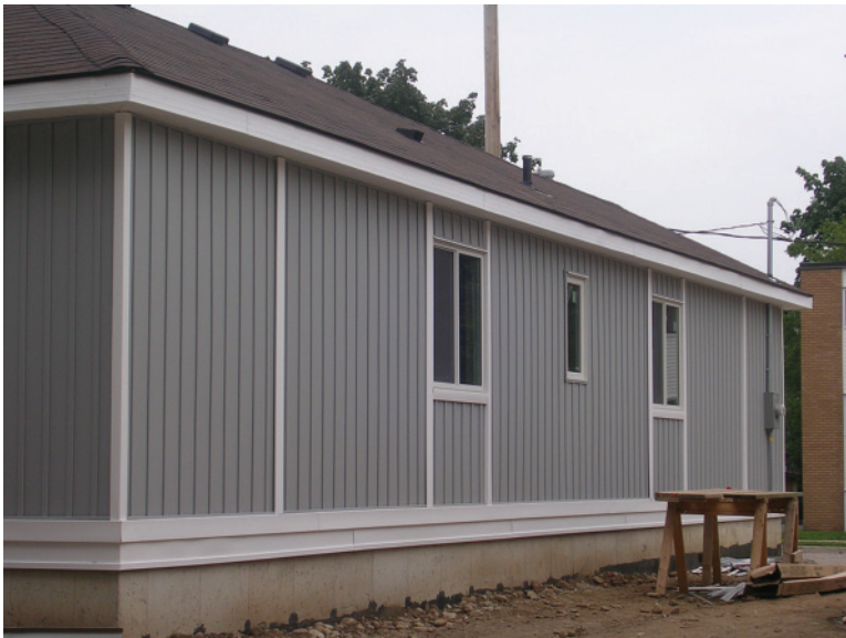
Top Left: 2.280 Installing board and batten siding panels above a window.
