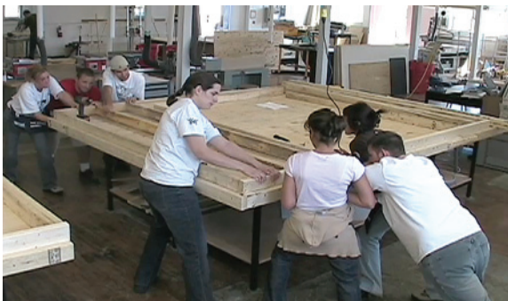
Left: 2.69 Pushing and pulling to force the wood into place. Below Left: 2.70 A small interior wall panel. Below: 2.71 A very small interior wall panel.
