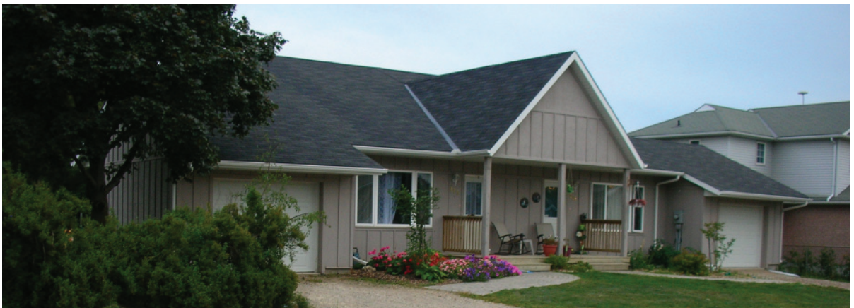
Above: 2.18 Plywood and batten clad Habitat for Humanity house in Elora.
