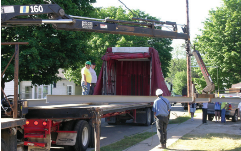
Above: 2.164 Unloading a steel beam.
