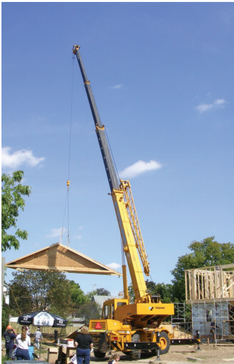
Above Left: 1.27 Lifting a framework of joists and rim boards on top of the first floor walls.
