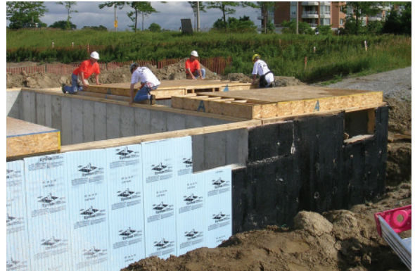
Above Left: 1.7 A floor section is placed where the boom can reach.
