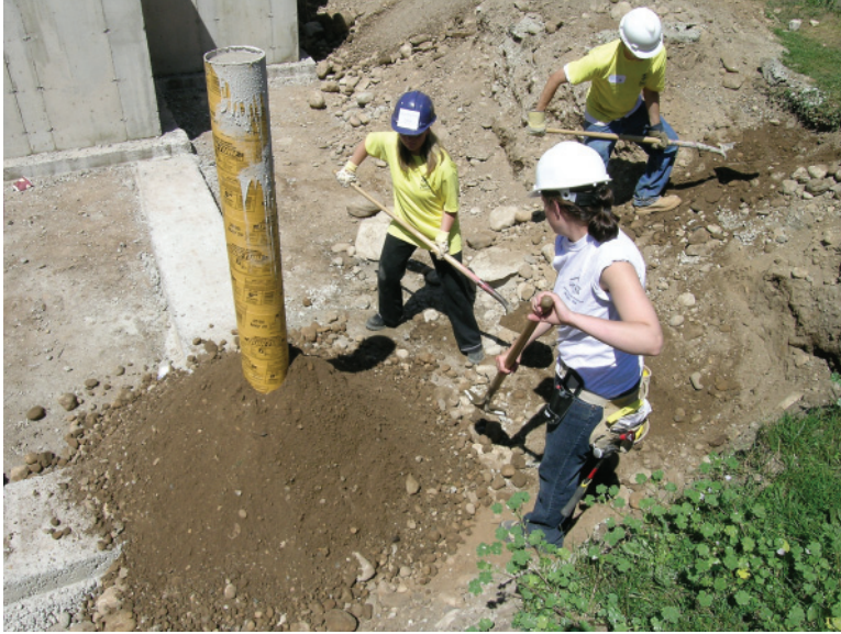
Left: 2.157 Packing dirt around a concrete pier to stabilize it. Below: 2.158 The footings.
