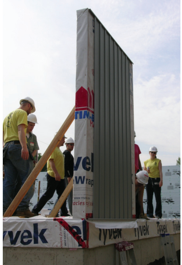
Below: 2.190 The first erected wall panel.
