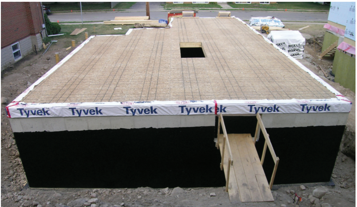
Below: 2.180 The completed floor deck.
