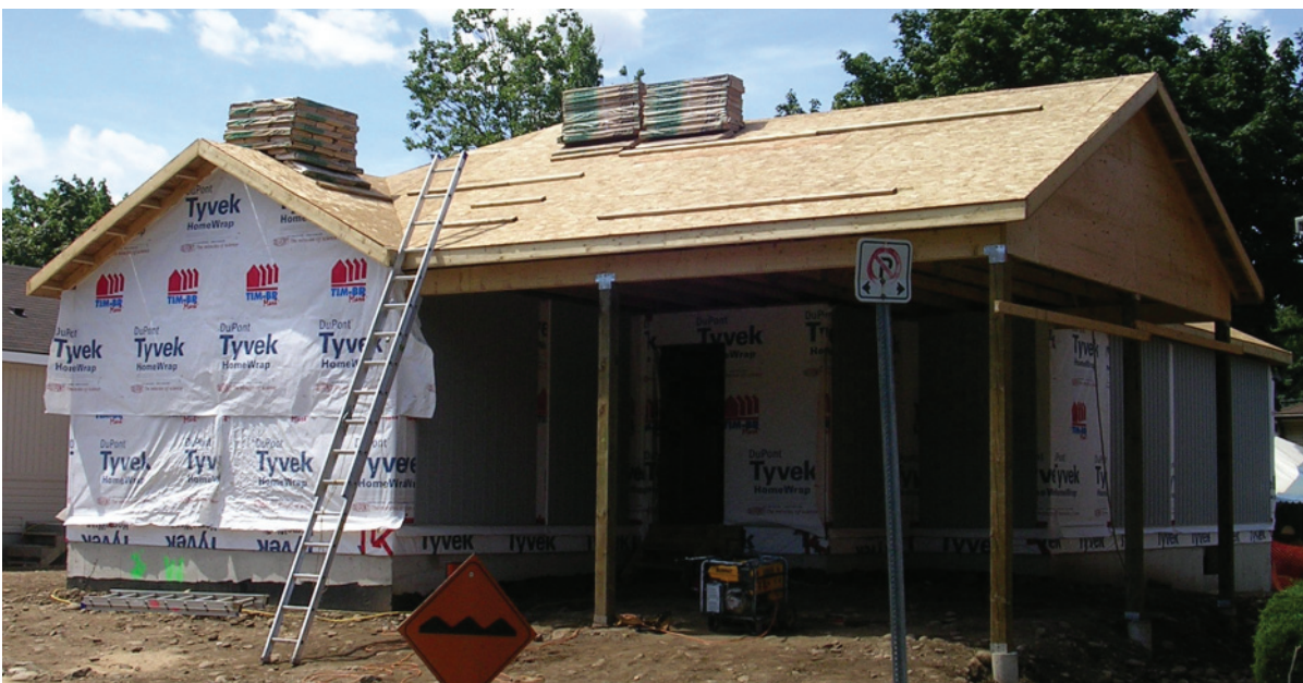
Below: 2.243 Bundles of shingles on top of the complete roof sheathing.
