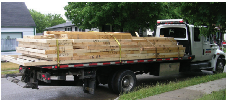
Above Left: 2.149 Storing unloaded exterior wall panels at the back of the site.
