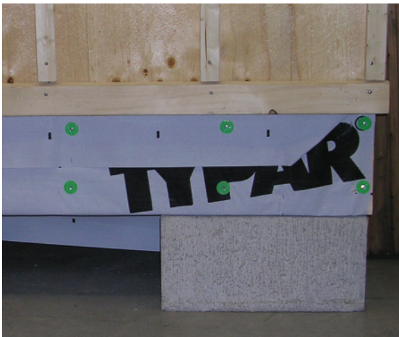
Above Left: 2.21 A nail with a plastic washer.
