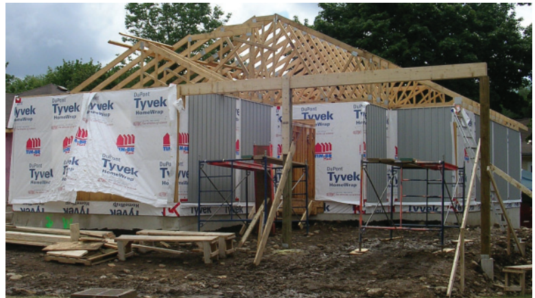
Below: 2.234 The erected roof trusses, carport posts, and carport beam.
