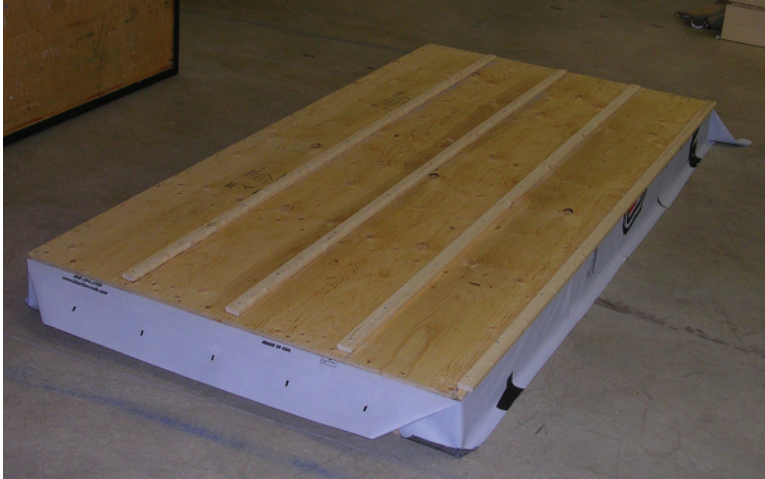
Left: 2.17 Wood battens nailed to the plywood completes the panel.
