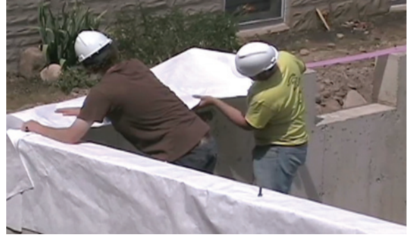
Above Left: 2.169 Installing sill gasket along the top of the foundation wall.
