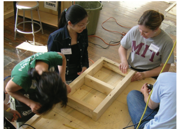
Left: 2.69 Pushing and pulling to force the wood into place. Below Left: 2.70 A small interior wall panel. Below: 2.71 A very small interior wall panel.
