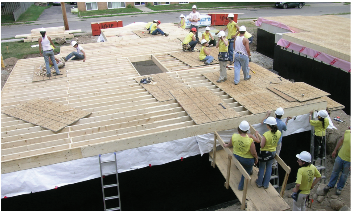
Below: 2.175 All of the joists are installed.
