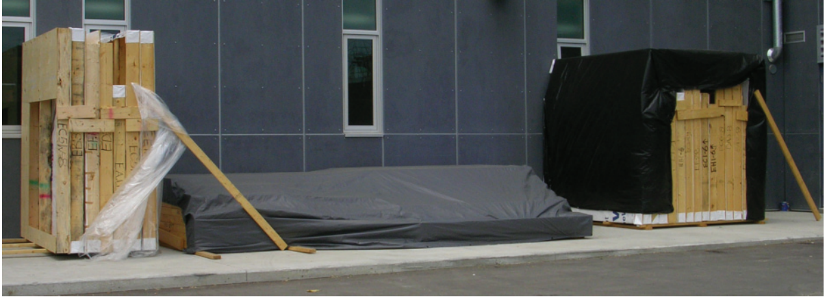
2.124 All of the wall panels required to frame the house.
