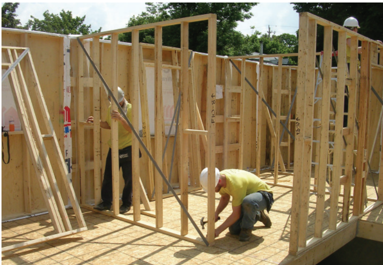
Below: 2.205, 2.206 Erecting interior wall panels.
