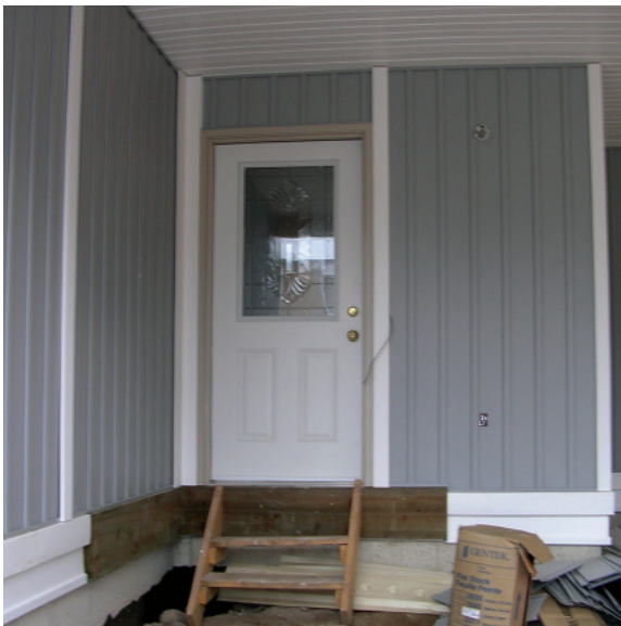
Top: 2.275 Siding complete on the front wall of the house.
