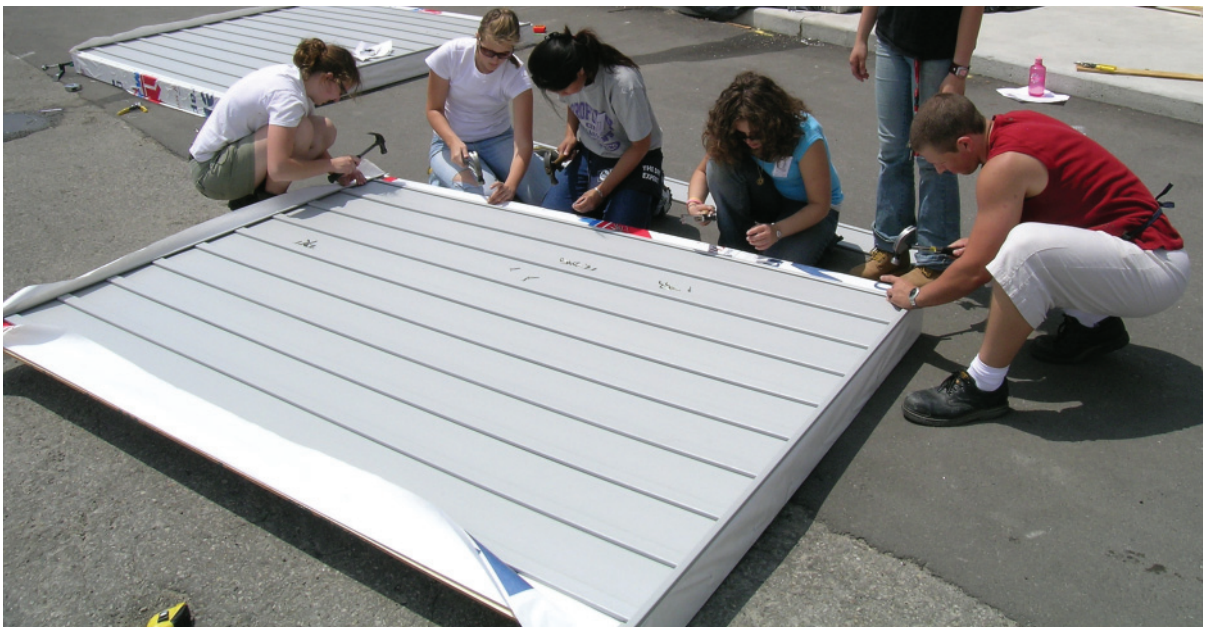
Top Left: 2.138 Trimming the first siding panel to its calculated width.
