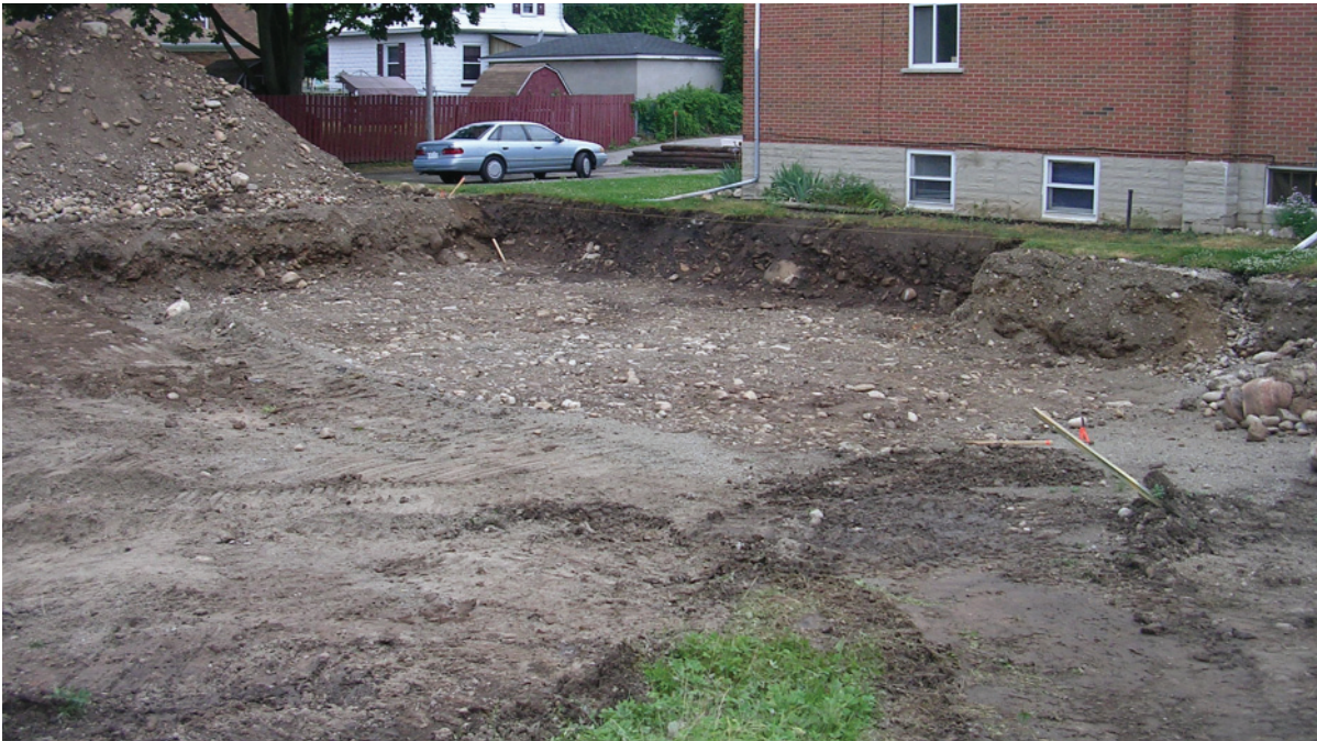
Top 2.126 An outline of the house marked out on the ground.
