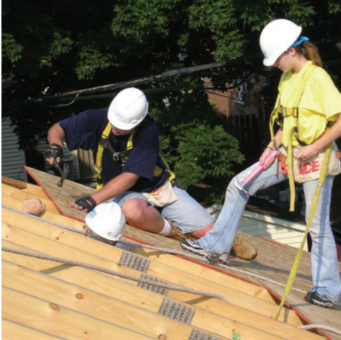
Above: 2.240 Driving a nail at the corner of a sheet of OSB roof sheathing to secure it in place.
