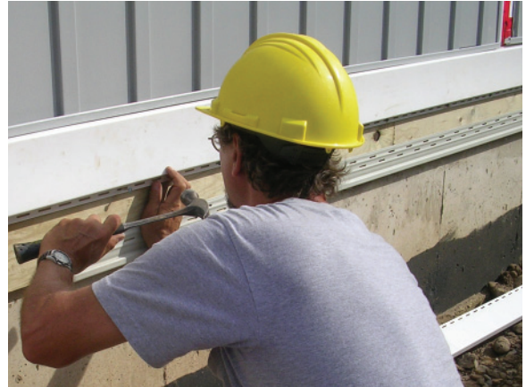
Above Left: 2.270 Installing the starter pieces for the horizontal band of siding.
