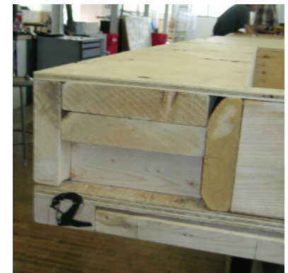
Below: 2.114 The top plate, lintel, and header plate of a completed exterior wall panel.
