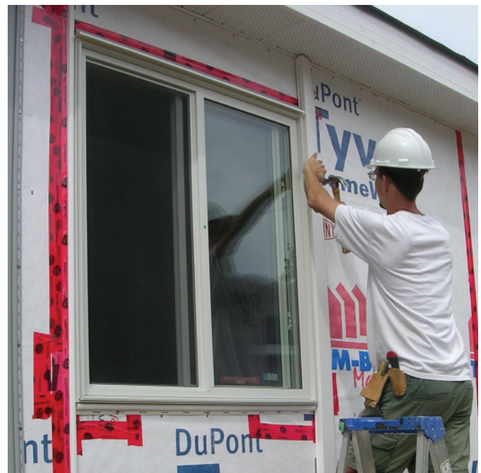
Below: 2.274 Installing a piece of three-and-a-half-inch-wide window trim alongside a window.
