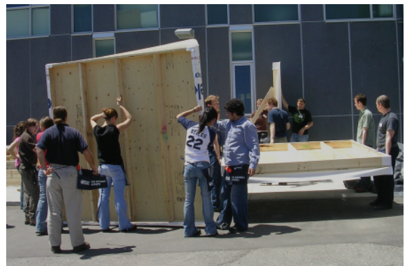
Below: 2.94 Confusion over the correct orientation of the wall panels for storage causes delays.
