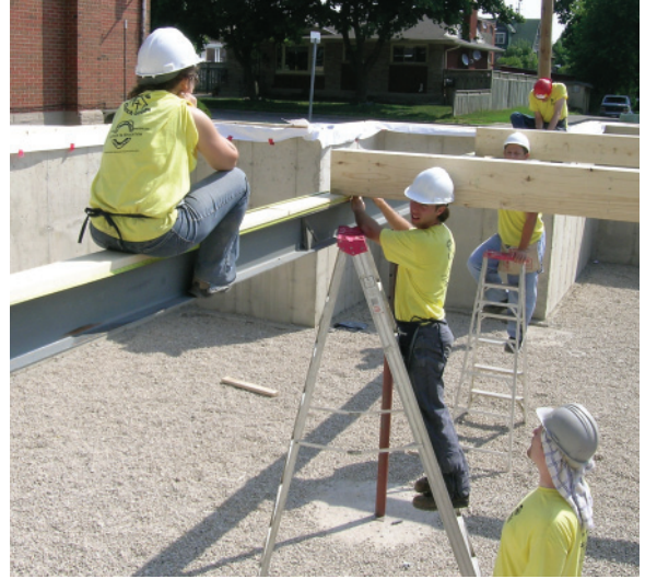
Above Left: 2.172 Installing rim boards.
