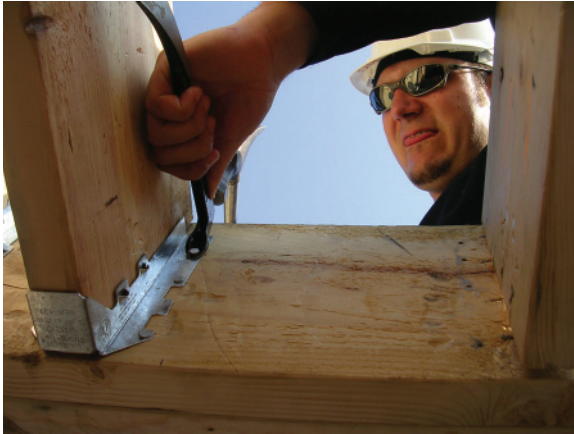
Left: 2.179 Pulling a nail out of a joist hanger.
