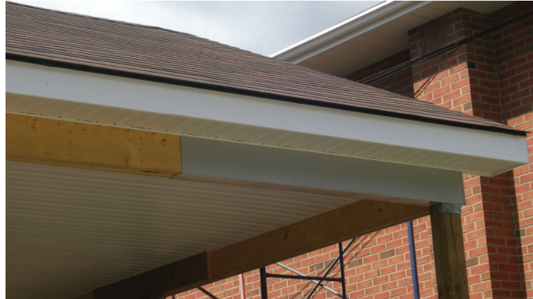
Left: 2.291 The first section of aluminum installed to a carport beam.
