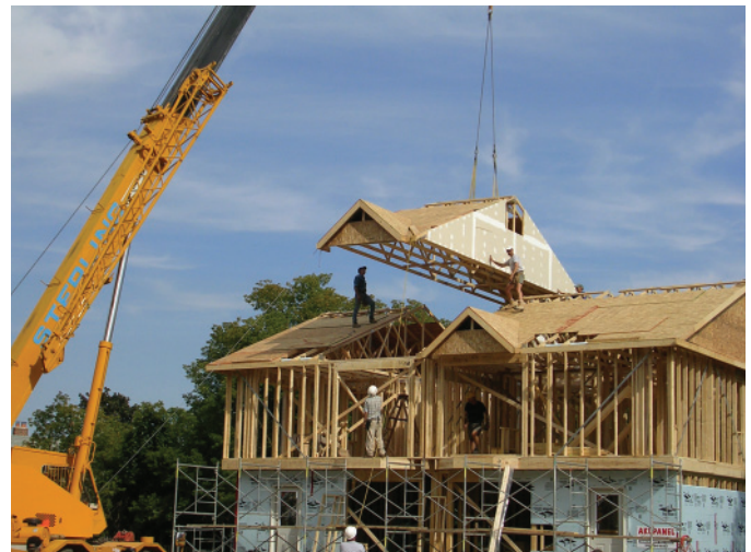
Below: 1.31 Installing the last roof section.
