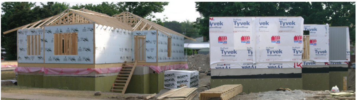
Top: 2.221, 2.222 Erected and capped interior wall panels.
