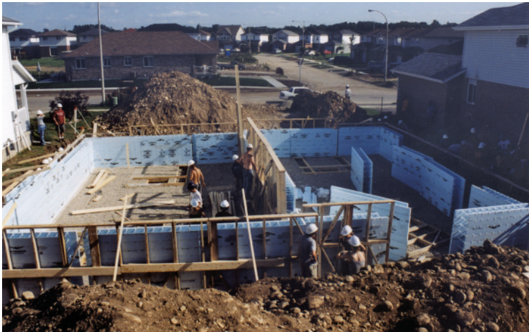
1.2 Carrying preassembled insulating concrete forms into the excavation.
