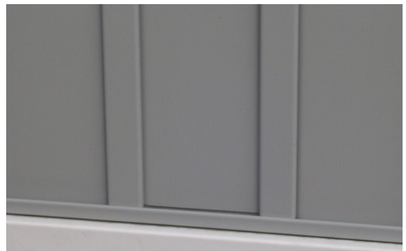
Bottom: 2.290 Siding panels that are installed too low.
