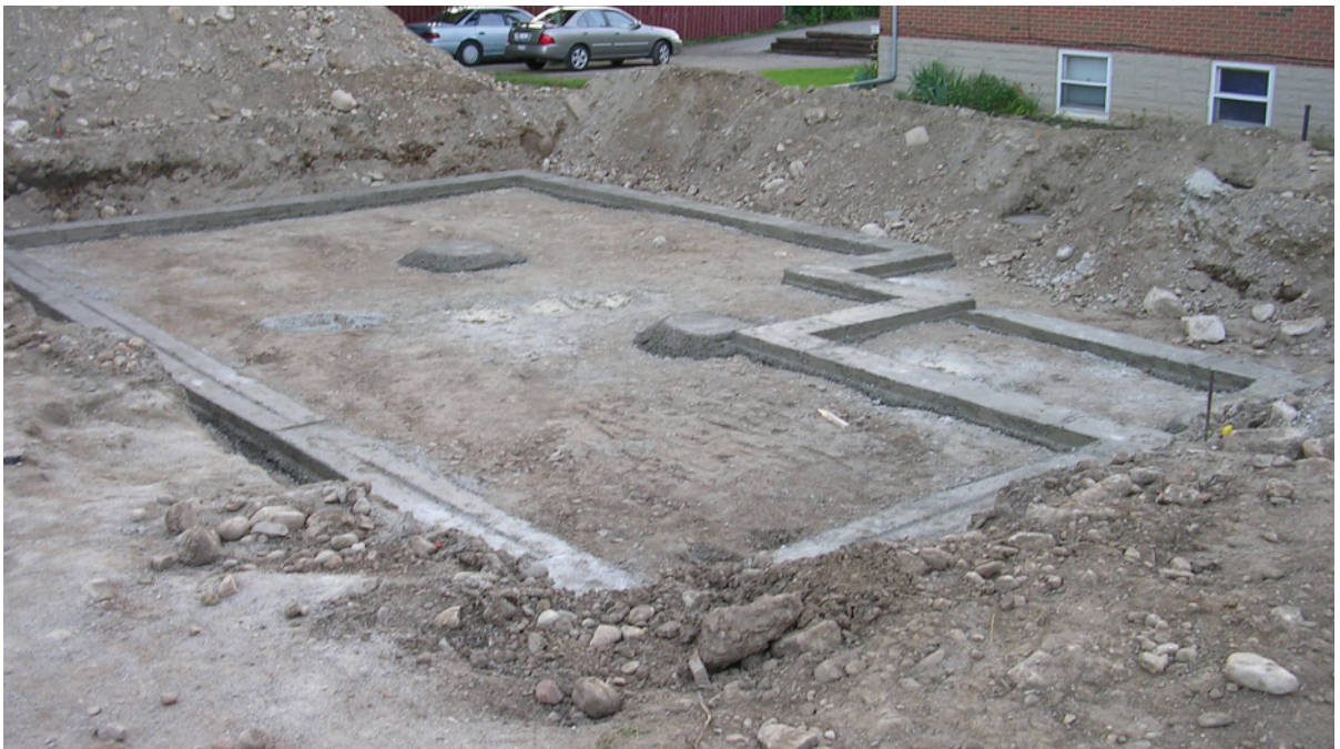
Left: 2.157 Packing dirt around a concrete pier to stabilize it. Below: 2.158 The footings.
