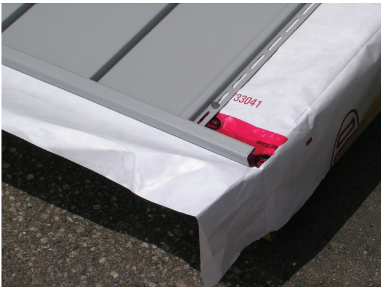
Top Left: 2.138 Trimming the first siding panel to its calculated width.
