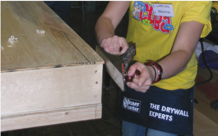
2.103 Sheathing an exterior wall panel on the floor of the workshop.
