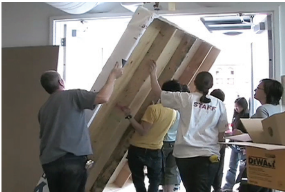
Left: 2.92 Carrying a wall panel at an angle out through the door of the workshop.
