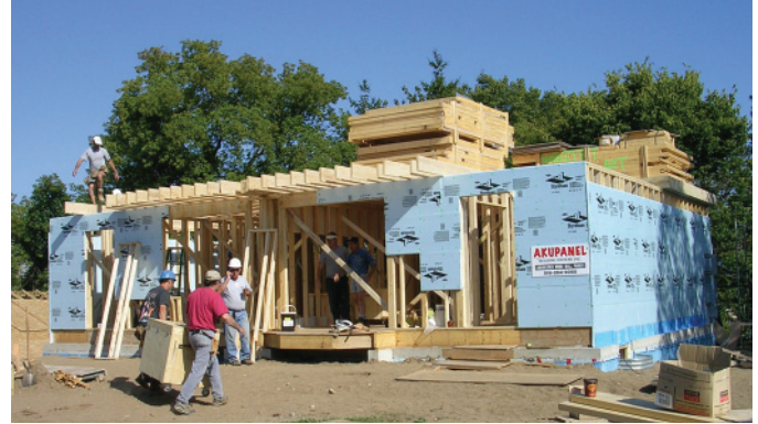
Above Left: 1.27 Lifting a framework of joists and rim boards on top of the first floor walls.
