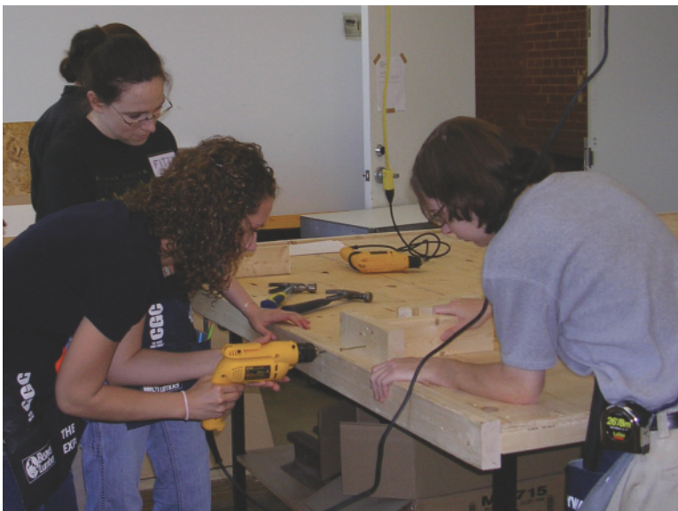
2.45 Practicing to drive screws into two-by-fours with a drill.
