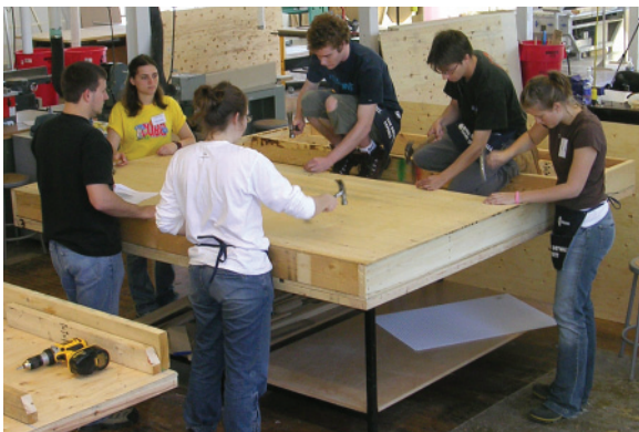
Above: 2.81-2.84 Installing the plywood sheathing.
