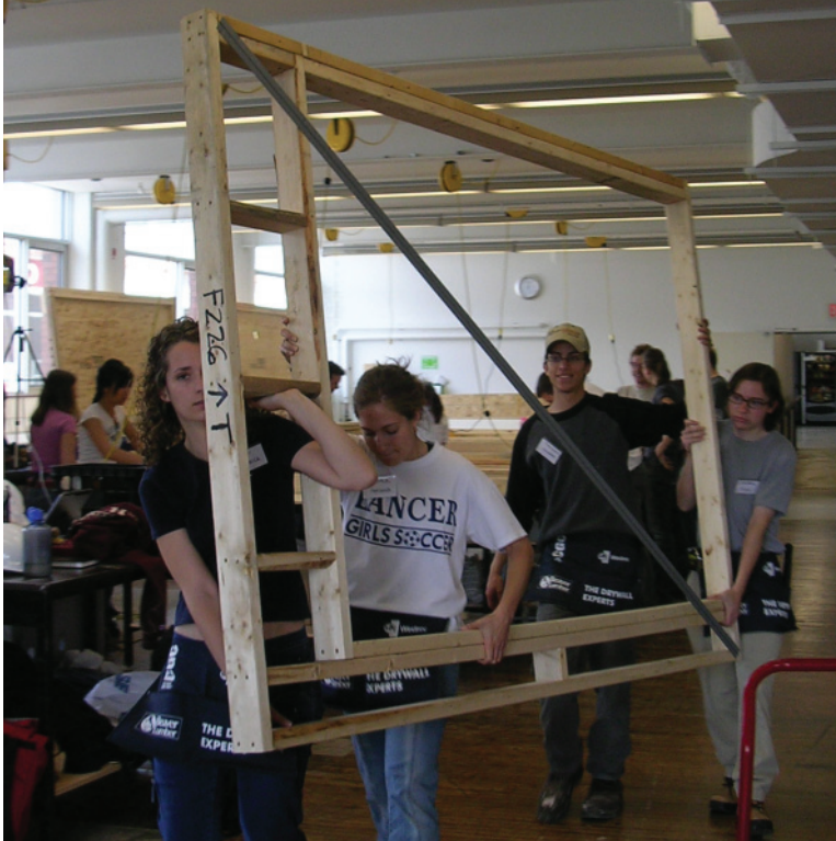
2.53 Carrying a finished interior wall panel through the workshop.
