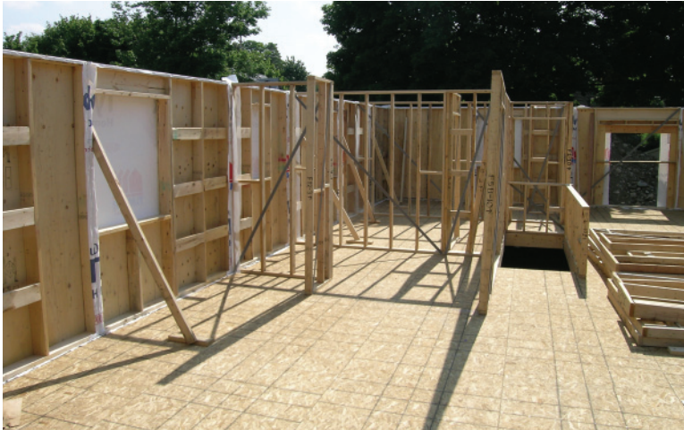
Above Left: 2.207 Installing polyethylene vapour barrier to an exterior wall where an interior wall panel will be installed.
