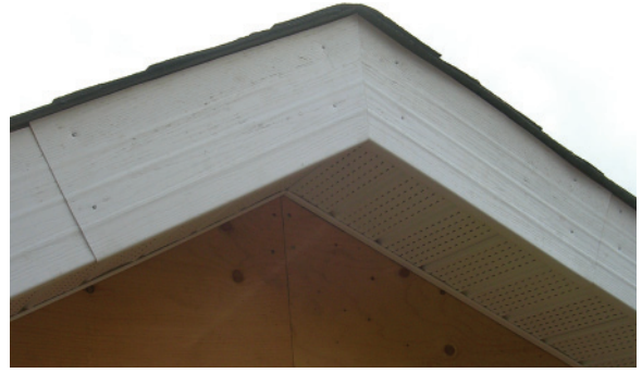
Above Left: 2.285 Poorly installed vinyl fascia.
