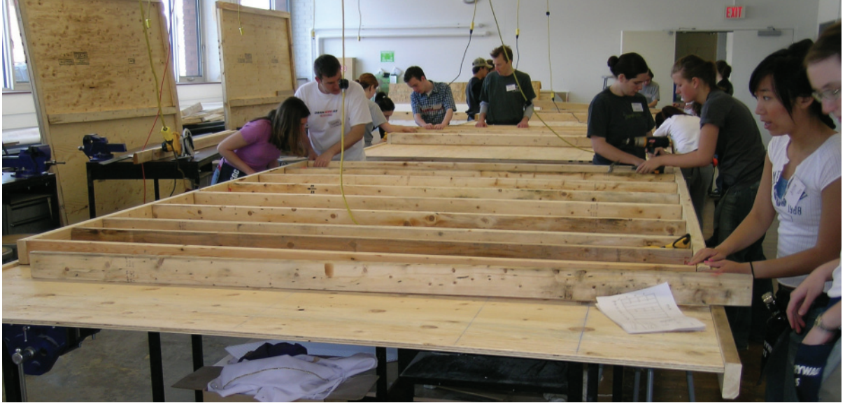
Above: 2.43 Assembling interior wall panels.
