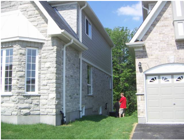
Figure 5.43: Kitchen test site, showing proximity of adjacent house
