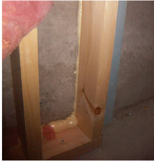
Figure 5.55: Air sealing at perimeter of stud frame walls
