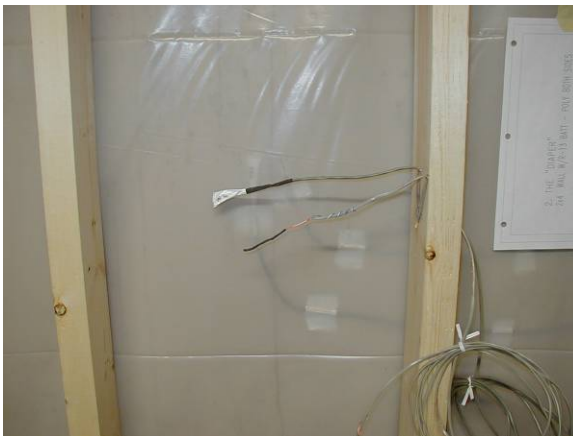
Figure 5.24: Instrumentation package at middle location of stud frame walls (Wall 2)
