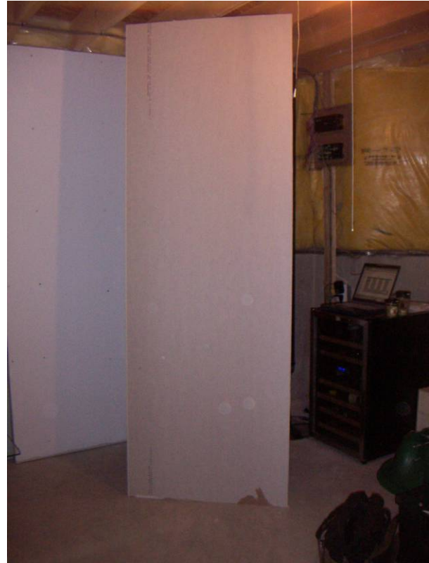
Figure 7.31: Exterior face of drywall in frame-latex paint wall
