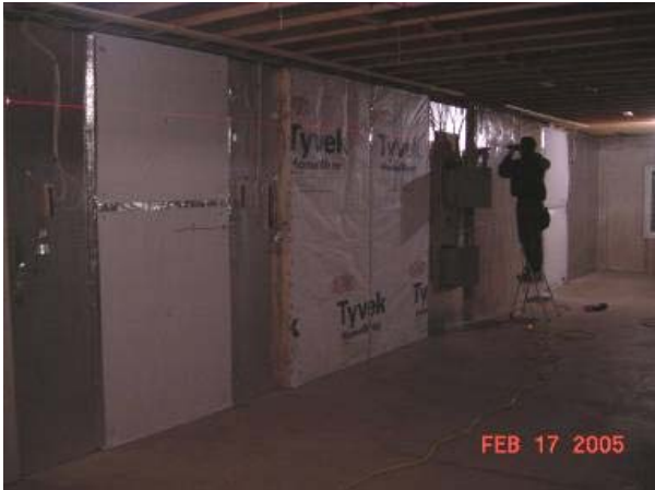
Figure 33: Holes were drilled at the same elevation in each wall
