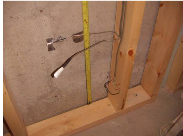
Figure 5.59: Sensors at lower location of stud frame wall
