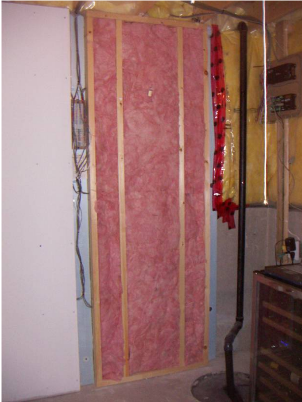
Figure 7.30: Frame-latex paint wall after drywall removal
