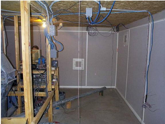
Figure 4.6: Owens Corning basement test (Goldberg and Aloï 2002)
