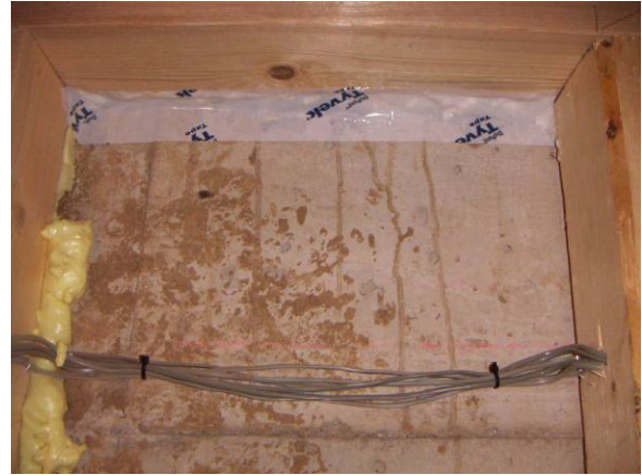
Figure 6.28: Panel 1 top connection sealed with builders' tape
