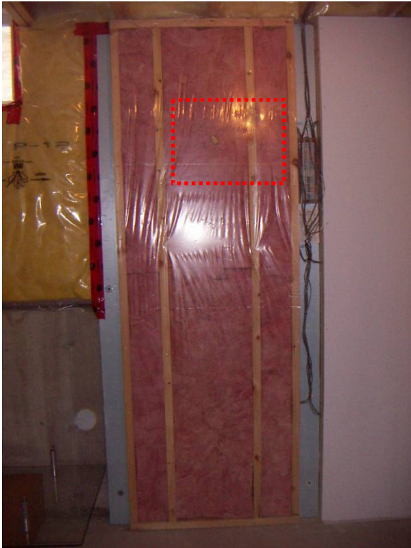
Figure 7.23: Frame-polyethylene wall after drywall removal
