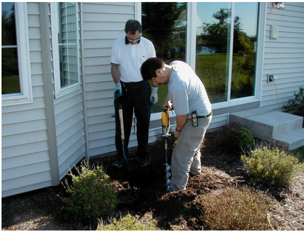
Figure 5.16: Boring for soil sensor installation, Huntley site
