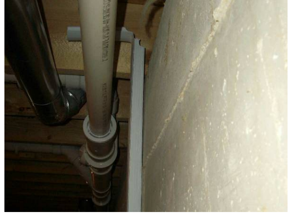
Figure 5.21: Concrete wall upper form extension out of plane
