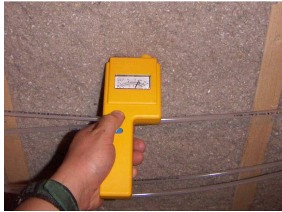
Figure 56: Handheld moisture meter measurement of cellulose insulation
