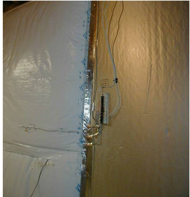
Figure 6.40: Roll blanket lateral seal condition in June 2004
