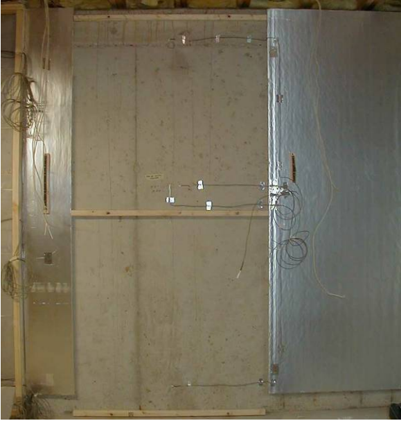
Figure 5.36: Installation of 2x2s at wall 8
