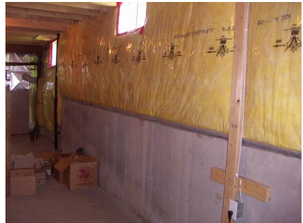
Figure 5.46: Location of test walls at Kitchener site, pre-installation
