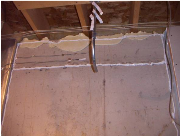
Figure 5.26: Caulk sealing and expanding foam at Wall 3 concrete
