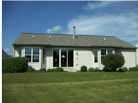
Figure 5.2: Rear elevation of Huntley test house
