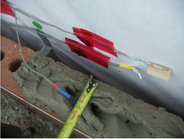
Figure 24: RH sensor and MC wafer in brick space cavity at UW test facility
