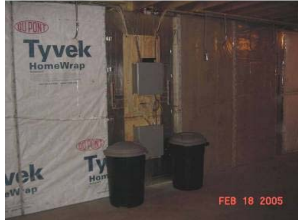
Figure 34: Reservoirs and pump and manifold housing
