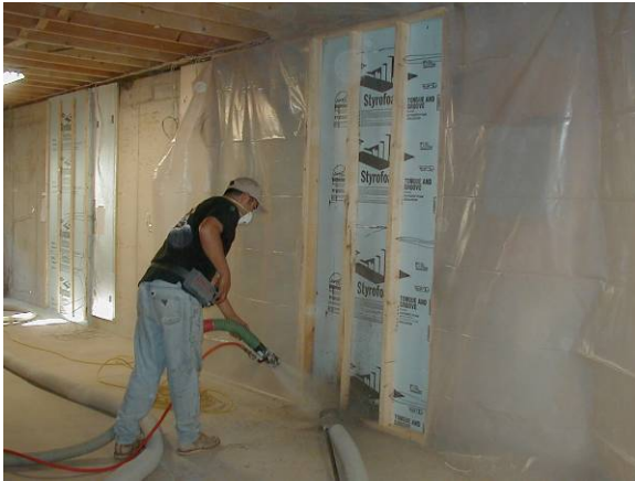
Figure 5.32: Installation of cellulose insulation in wall 6
