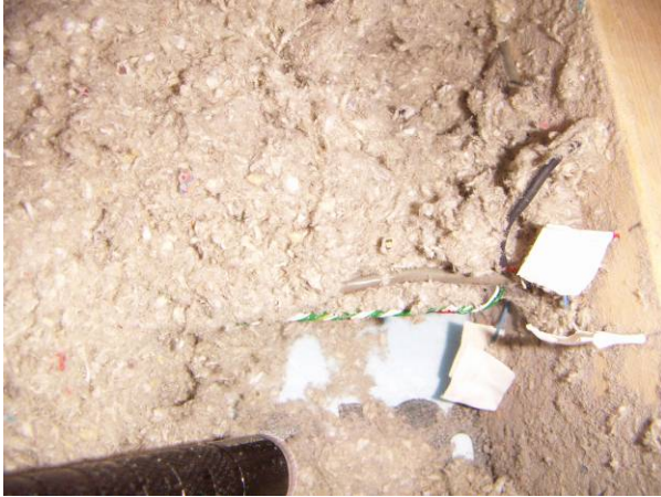
Figure 53: Wrapping pins with electrical tape, 9/05
