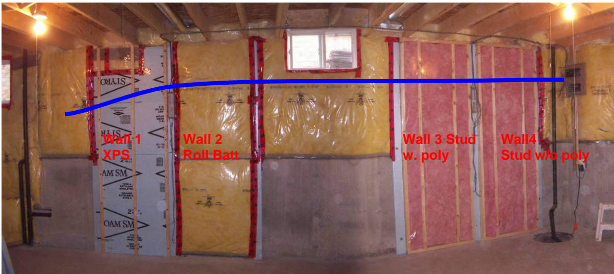
Figure 5.60: Test panels at Kitchener site (pre-drywall); approximate grade level shown
