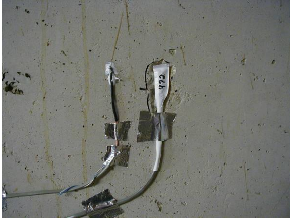
Figure 5.20: T and T/RH sensor at concrete
