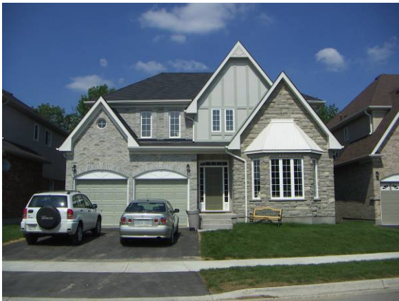
Figure 5.41: Front elevation of Kitchener test location
