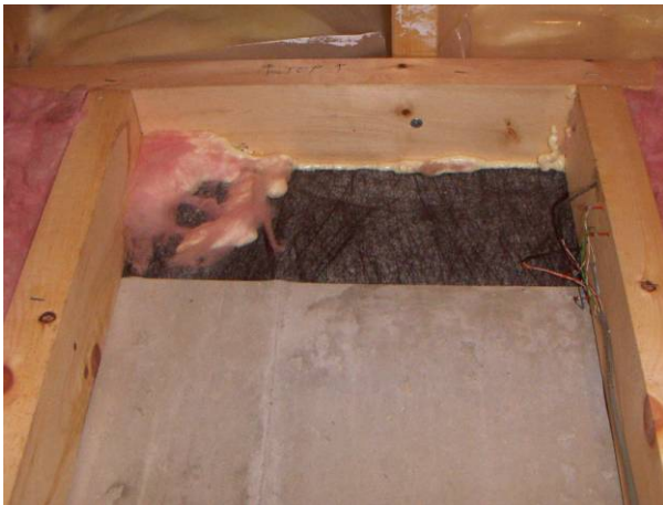
Figure 5.56: Air sealing at top plate of frame walls
