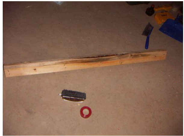
Figure 6.67: Close up of double polyethylene sill plate
