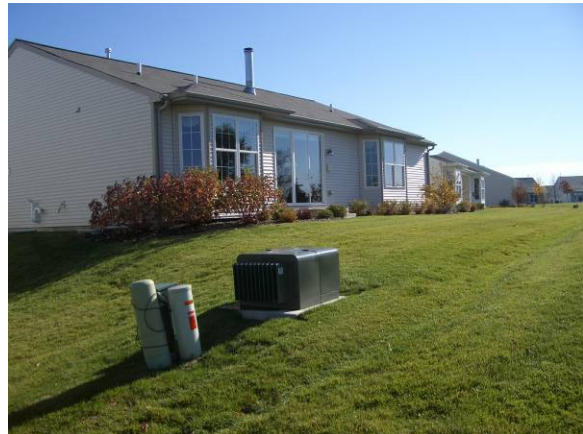
Figure 5.4: Rear oblique Huntley test house
