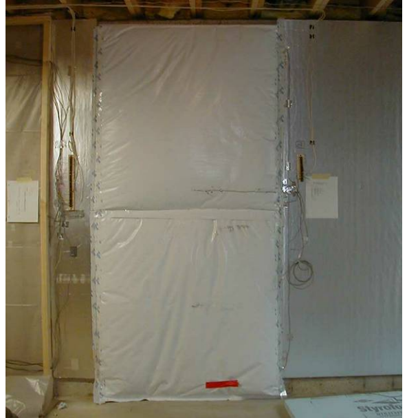
Figure 5.37: Completed installation of wall 8
