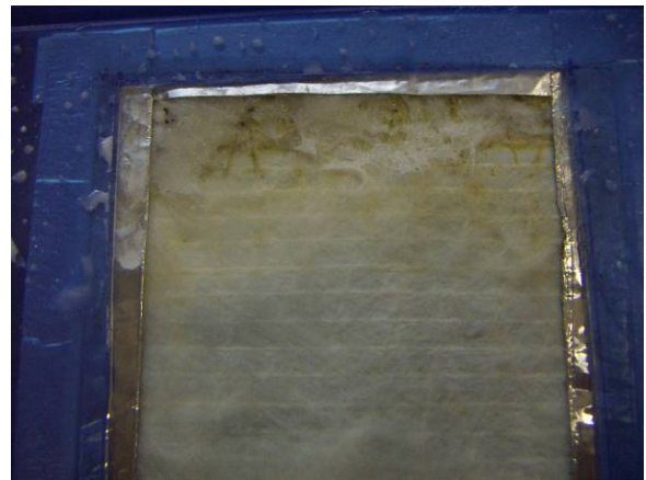
Figure 43: Detail of mold growth, showing water "matting" at one end
