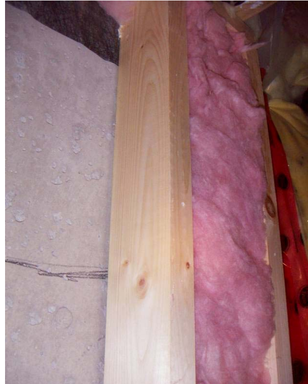
Figure 7.35: Upper right side stud of test bay
