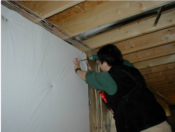
Figure 5.34: Installation of PA-6/rigid fiberglass material (wall 7)
