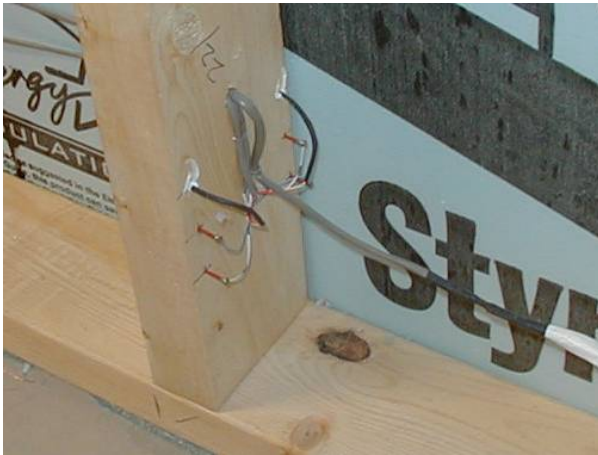
Figure 51: Original installation of MC pins (unpainted)
