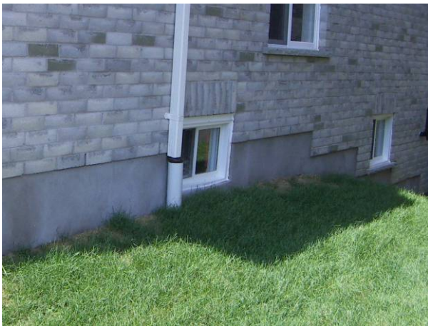
Figure 7.11: Exterior view of basement window, for vertical reference to brick ledge
