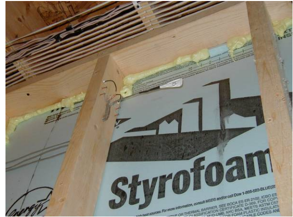
Figure 5.33: Top air sealing detail and foam wedge at wall 5
