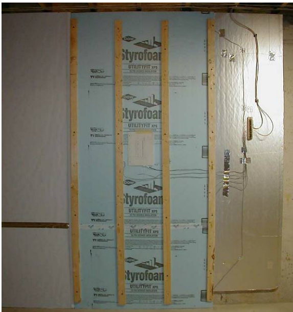
Figure 5.28: Installation of furring strips and foam at wall 4
