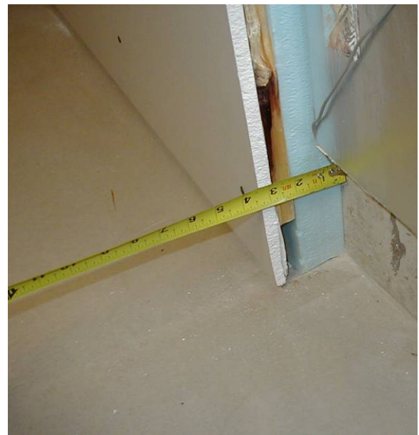
Figure 5.29: Completed assembly (side view) of wall 4
