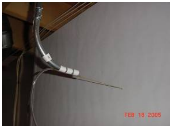
Figure 32: Injector, for size reference and as installed
