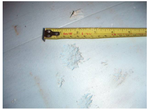
Figure 6.71: Craters or burrows on exterior
