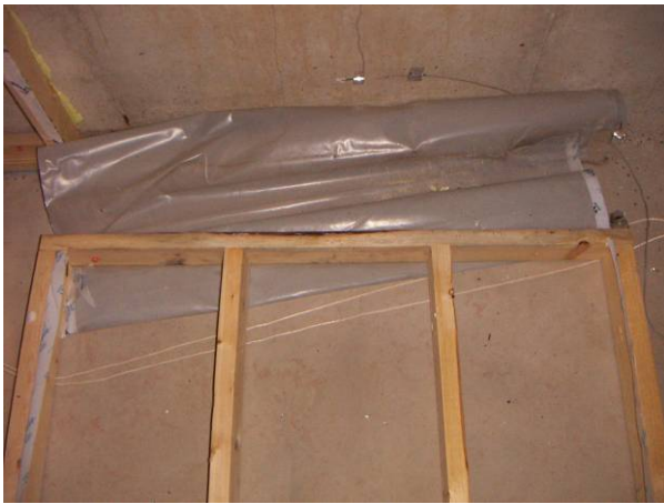
Figure 6.66: Sill plate of double polyethylene wall (panel 2)
