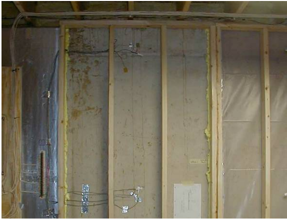
Figure 5.22: Lateral air sealing at Walls 1 and 2 (stud frame walls)
