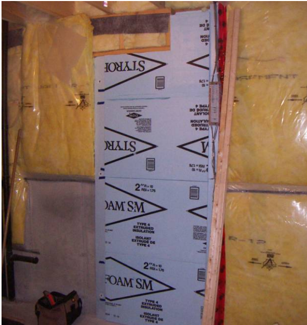
Figure 5.54: Installation of XPS wall at foundation step down
