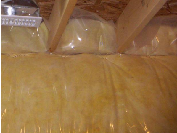
Figure 5.51: Existing rim joist condition at Kitchener site
