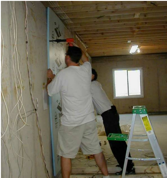
Figure 5.30: Installation of XPS board at wall 6 with powder actuated fasteners
