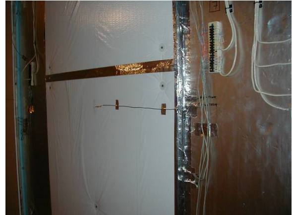
Figure 5.35: Lateral air sealing and joint sealing at wall 7
