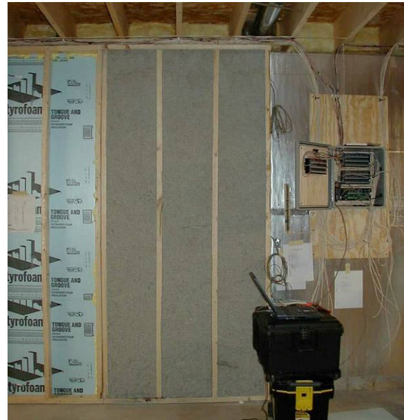
Figure 5.31: Installed cellulose insulation in wall 6
