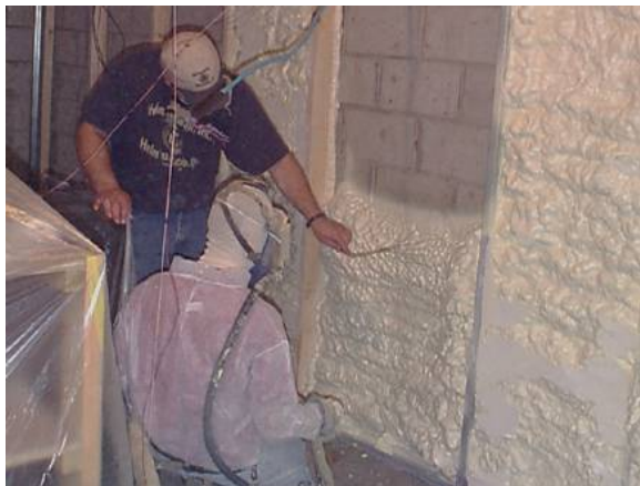
Figure 4.10: Installation of Icynene insulation (Goldberg and Farkas 2004)
