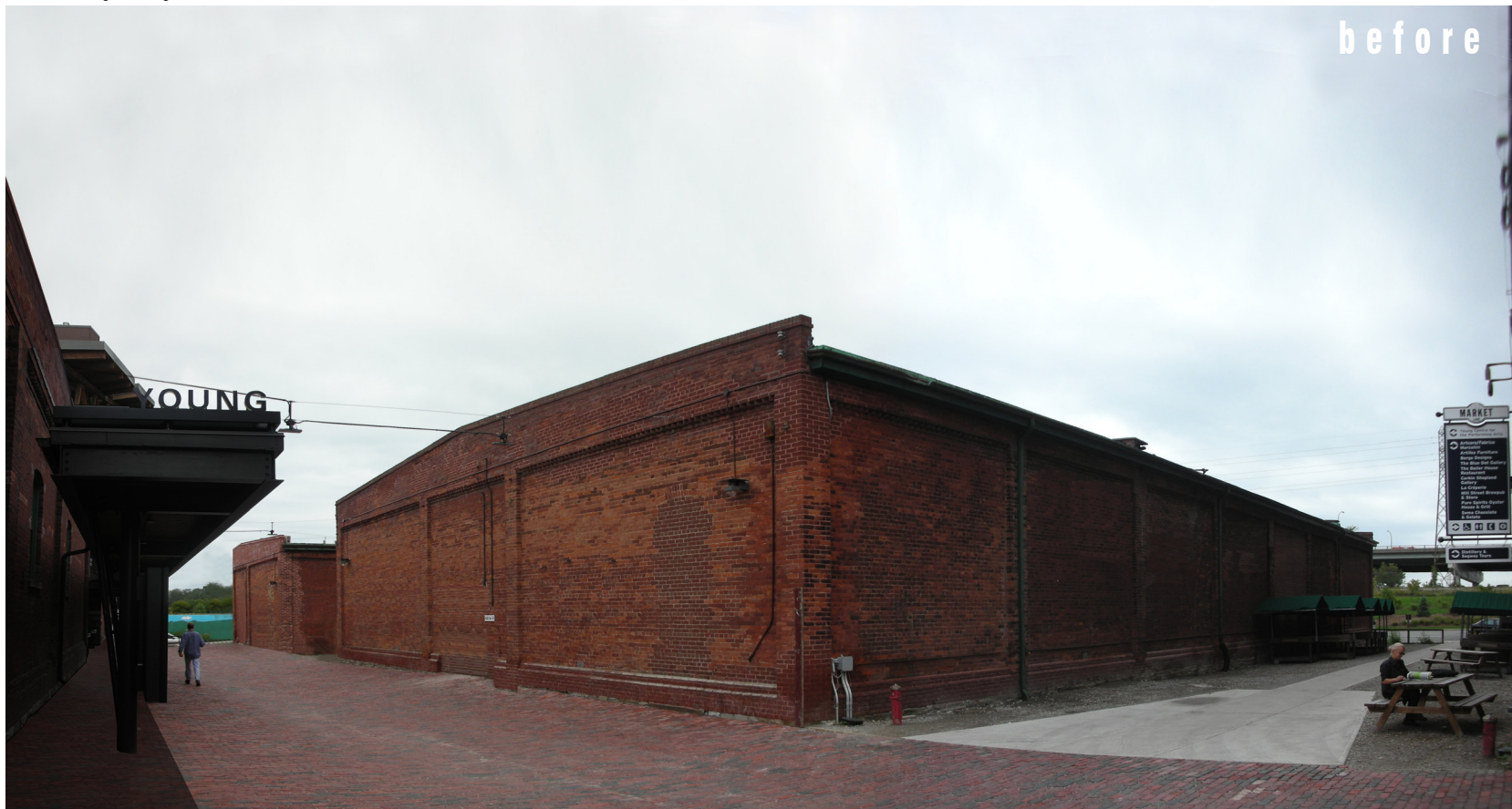
fig. 67 View of Existing Building From Tank House Lane
