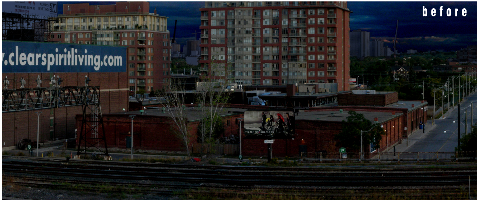
fig. 73 View of Existing Building From Gardiner Expressway at Night
