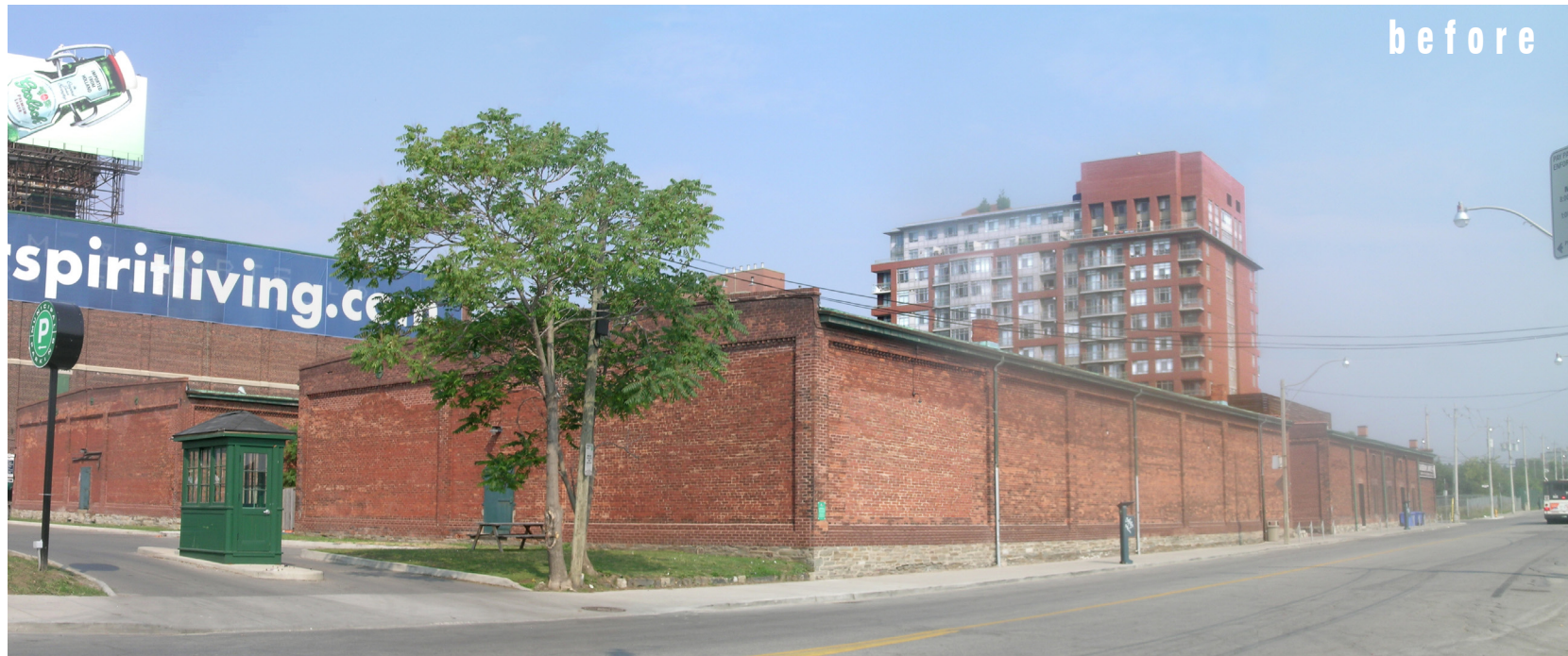
fig. 71 View of Existing Building Entering City Via Cherry Street
