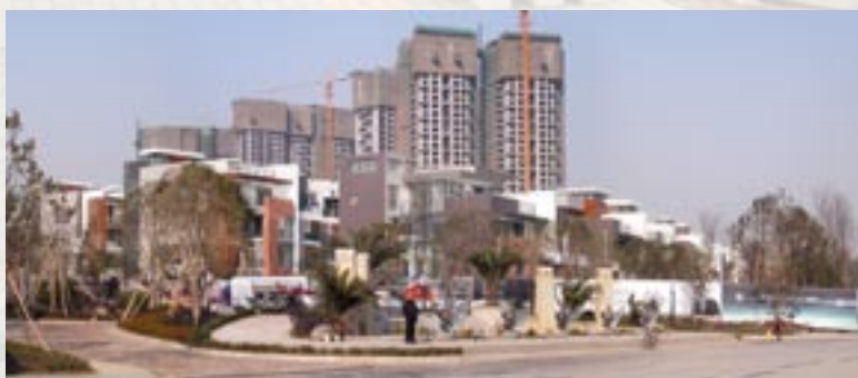
47 (spread) The Water Front Park Under Construction.
