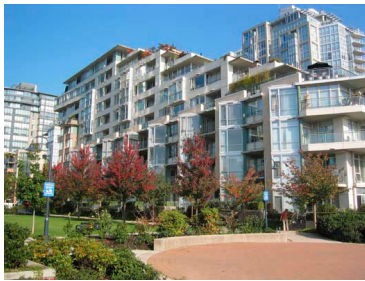
A Vancouver apartment building with directional bay windows, balconies, and roof terraces responds to view and solar orientation.
