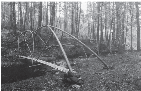
3.3 (c. 1995) The Bartel bent-wood bridge designed by The University of Nova Scotia (TUNS) architecture students and their professor Richard Kroeker. Sackville, Nova Scotia.
