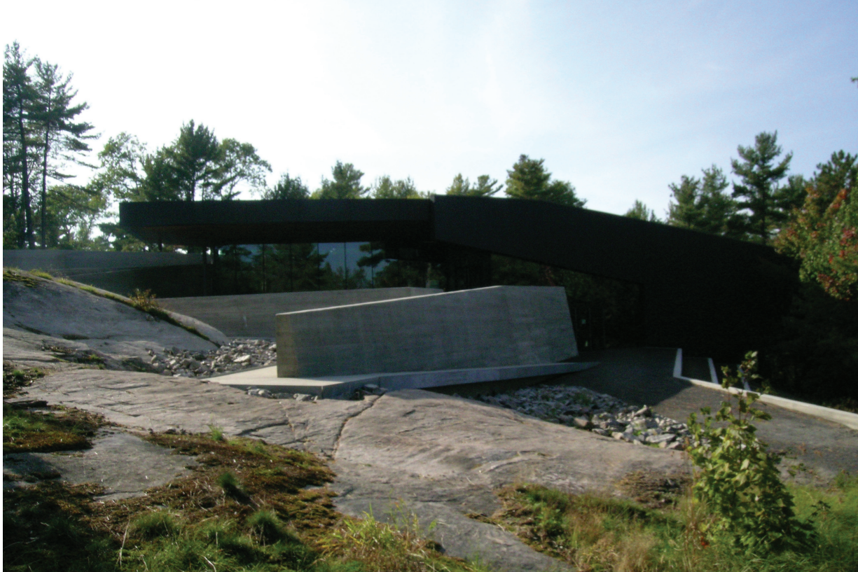
6.3 The French River Provincial Park Visitor Centre. Killarney, Ontario.
